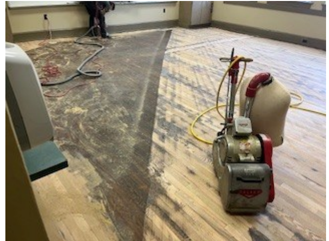
Drum sanding classroom floor 1st pass
