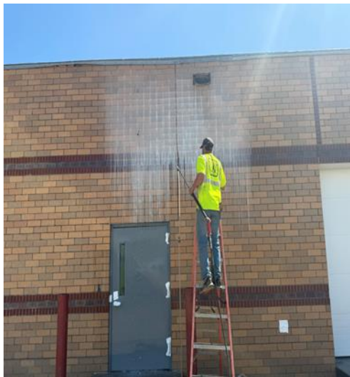
Exterior Acid Wash North Addition
