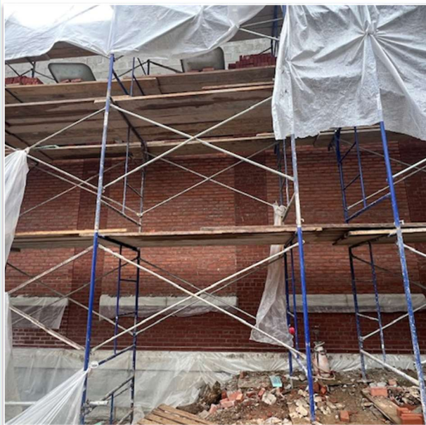
West elevation brick placement at KRS
