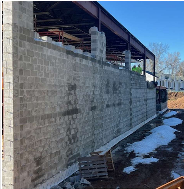
Western CMU Installation at CAS
