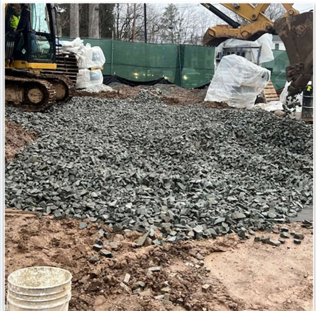
Track pad reconditioning at KRS
