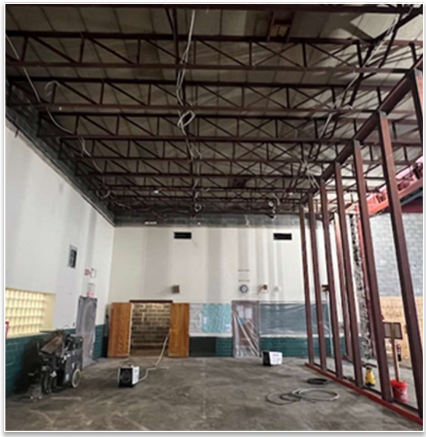
Drop ceiling removal at KRS
