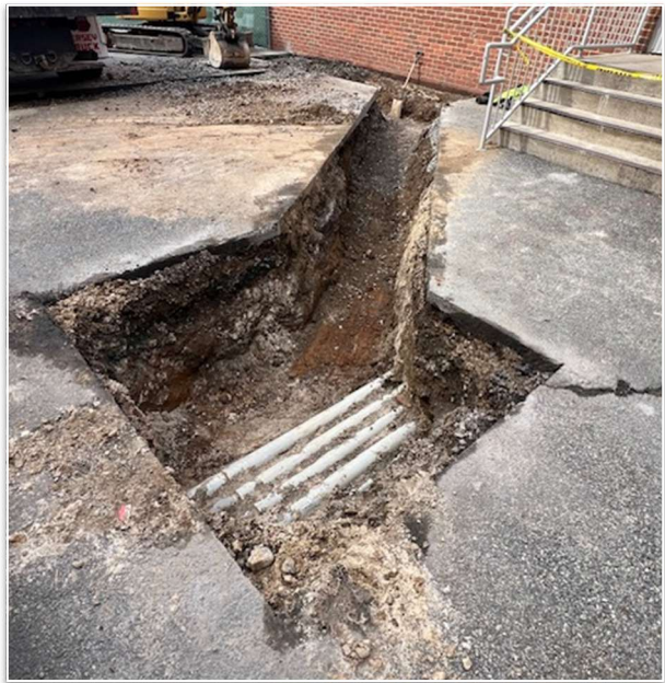
Transformer Excavation at CAS
