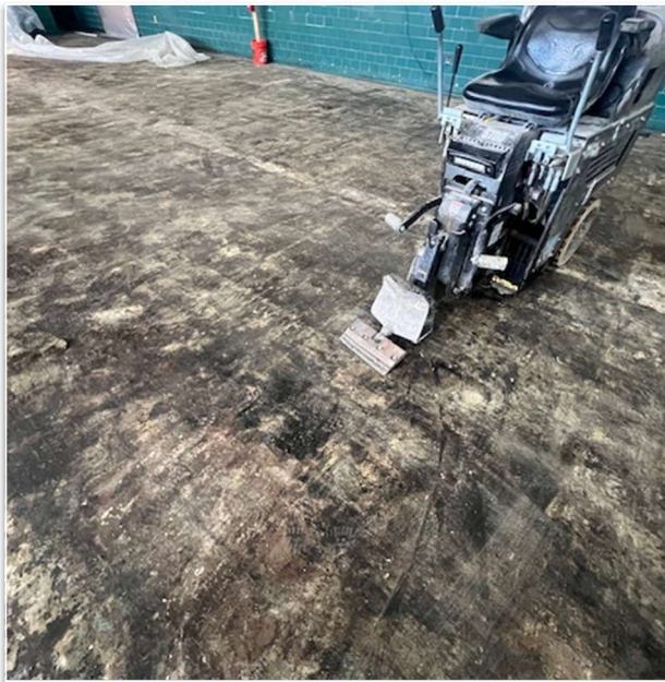
VCT flooring removal at KRS
