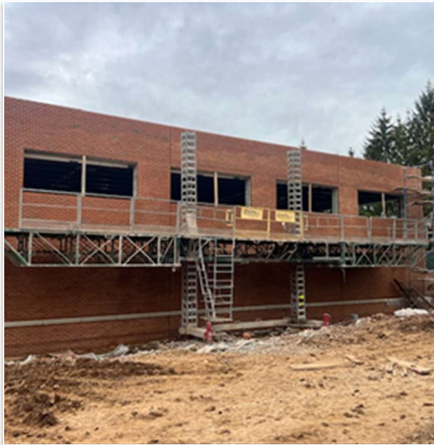
Southern Elevation Brickwork at CAS
