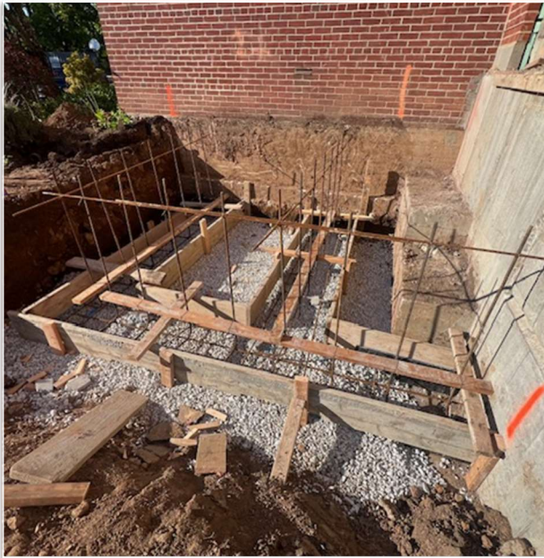
Rebar and Footings at KRS
