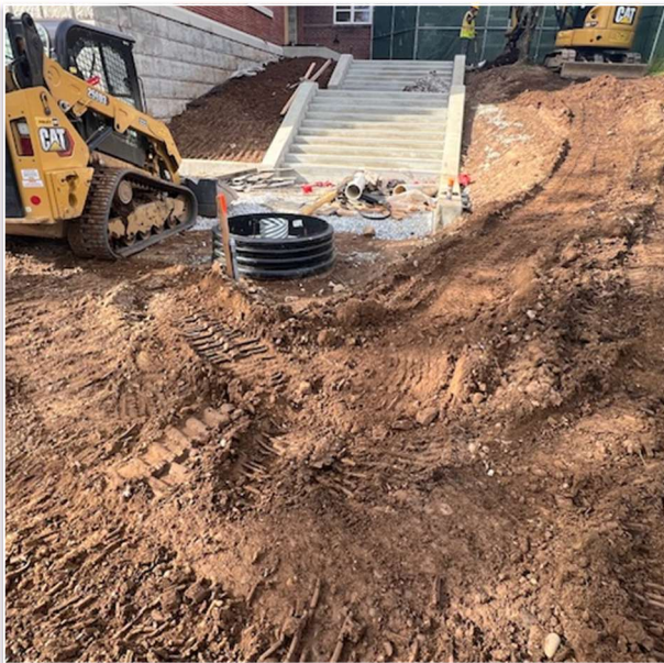
Cleanup and grading at KRS
