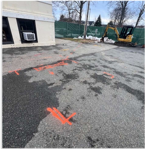
Transformer Excavation Layout at CAS
