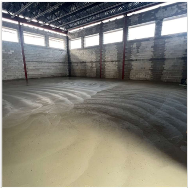
Concrete Slab Placement at KRS
