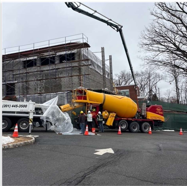
Pump Truck Placement at KRS
