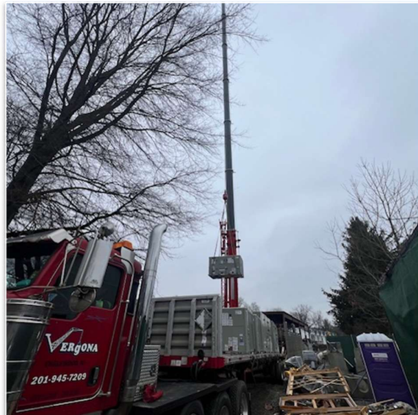
RTU pick with Crane at CAS
