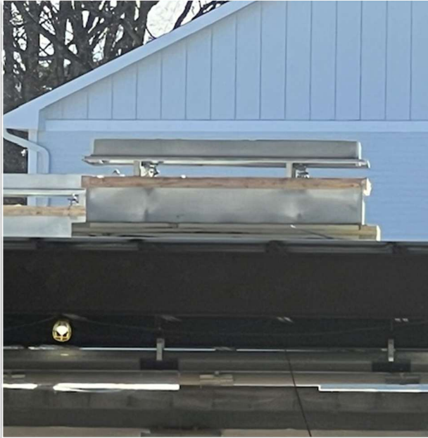
HVAC Curb Installation at CAS
