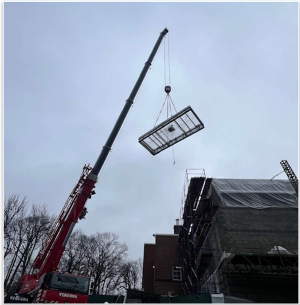
Curb placement with Crane at KRS
