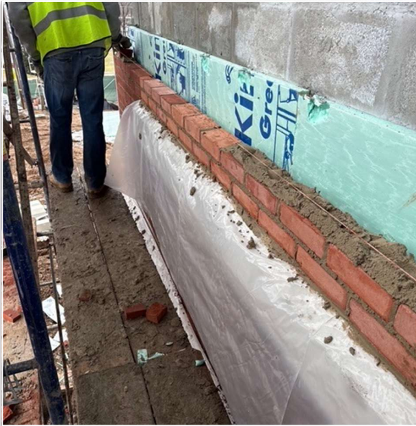
Brick Mock-up wall at KRS
