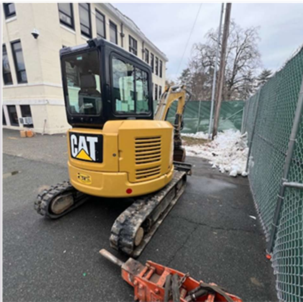
Temp Fence and Equipment at CAS
