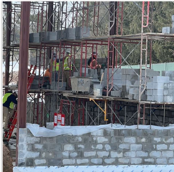
Grout and rebar installation at CAS
