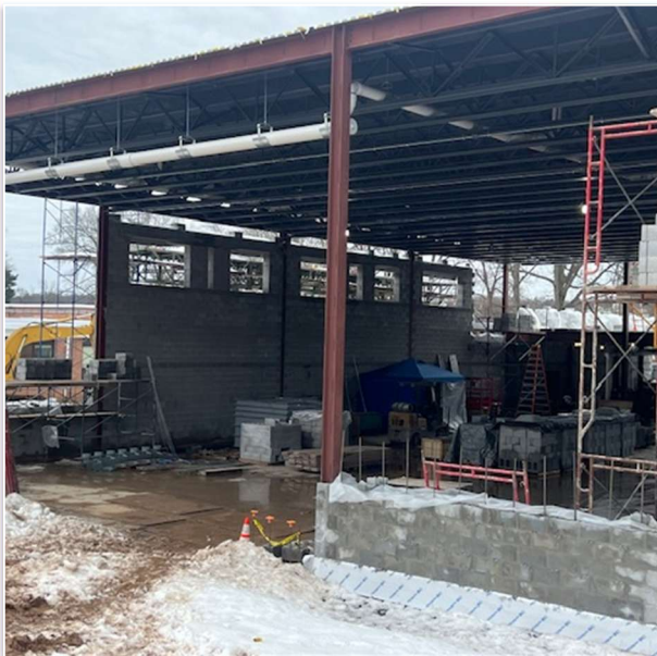
All trades progressing at CAS
