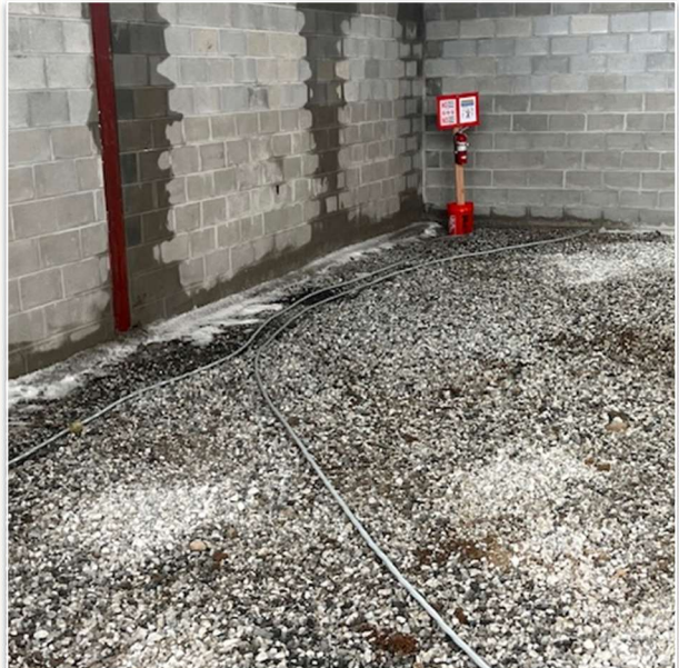
Electrical for Heaters at KRS
