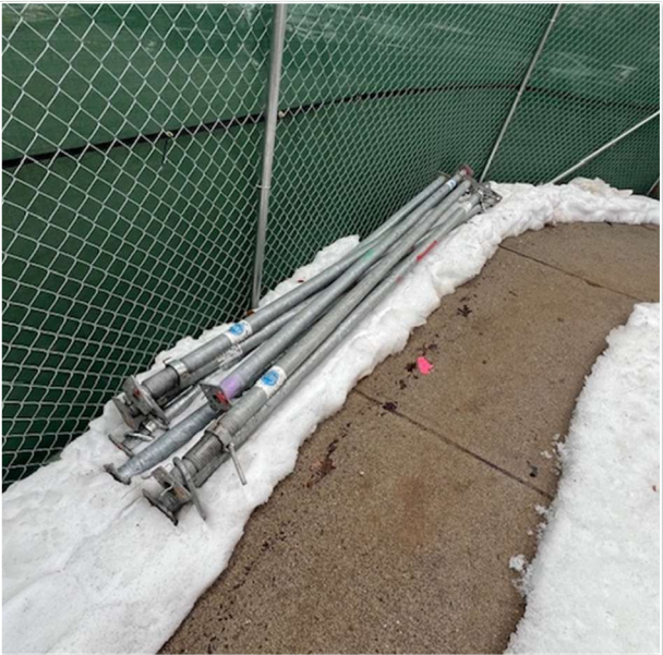
Temporary screw jacks removal at KRS
