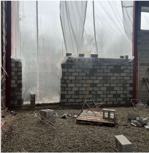
CMU installation West at KRS
