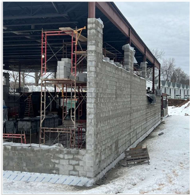
CMU installation Southwest at CAS
