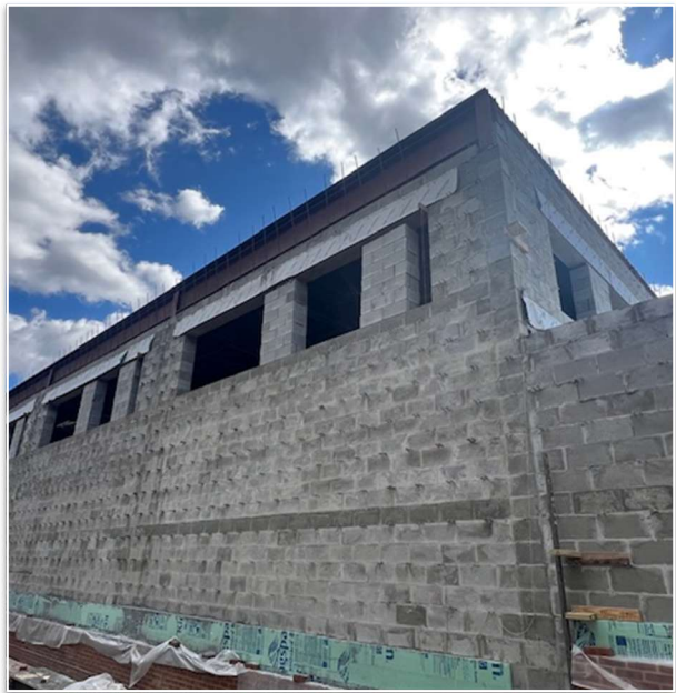
West Brick Work at CAS
