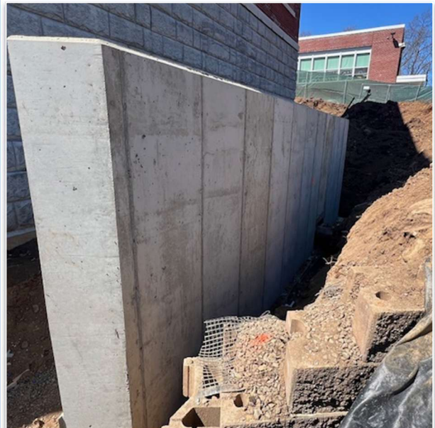
Sidewalk Retaining Walls at KRS
