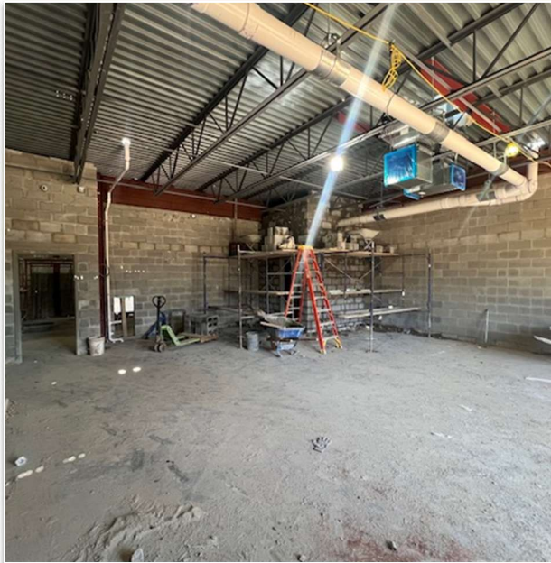
Interior CMU Installation at CAS
