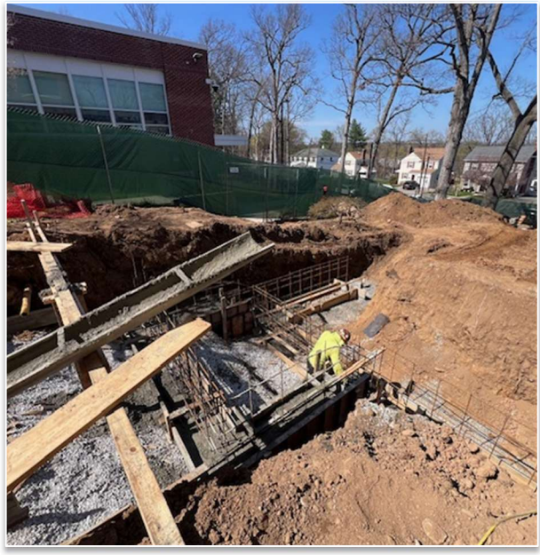
Concrete Placement and Rebar at KRS
