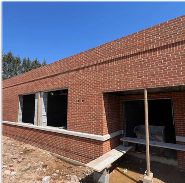
North Brick Placement at CAS
