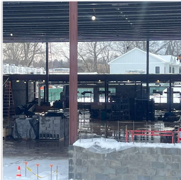
Interior work on hold at CAS
