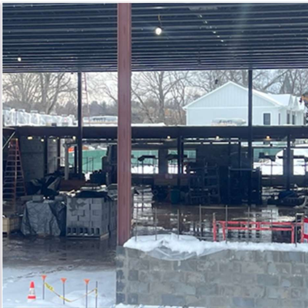
Interior work on hold at CAS
