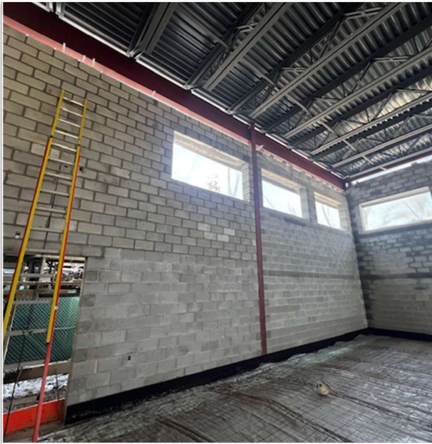
CMU installation West at KRS
