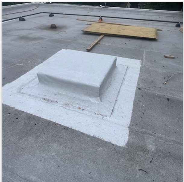
Roofing Repairs at KRS
