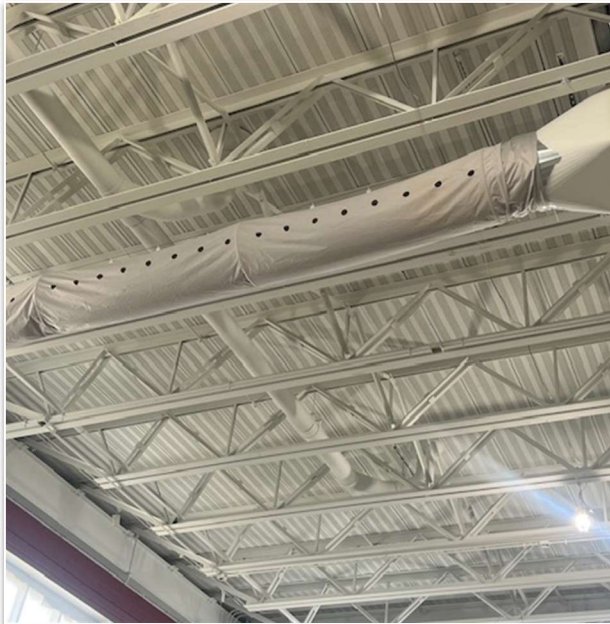
Duct Sock Installation at CAS
