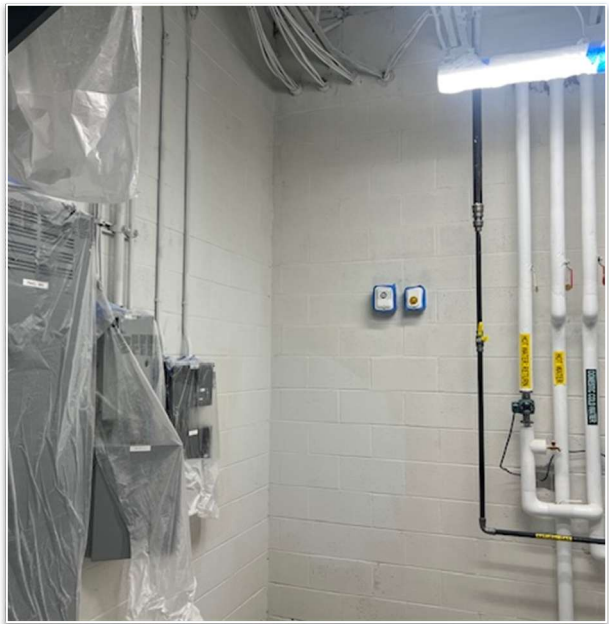
Storage Room Painting at CAS
