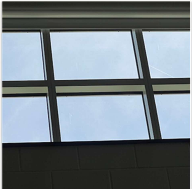
Roller Shade Installation at KRS
