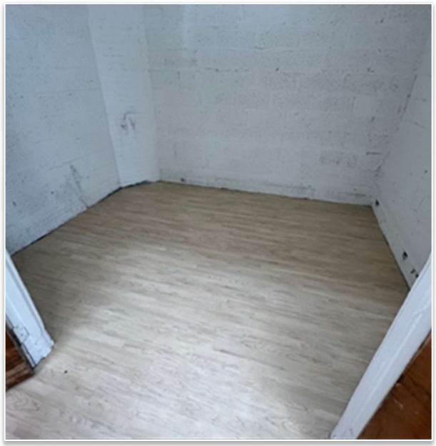
LVT Flooring Installation at KRS
