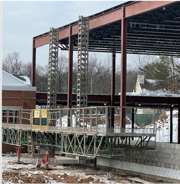
Scaffolding for CMU at CAS
