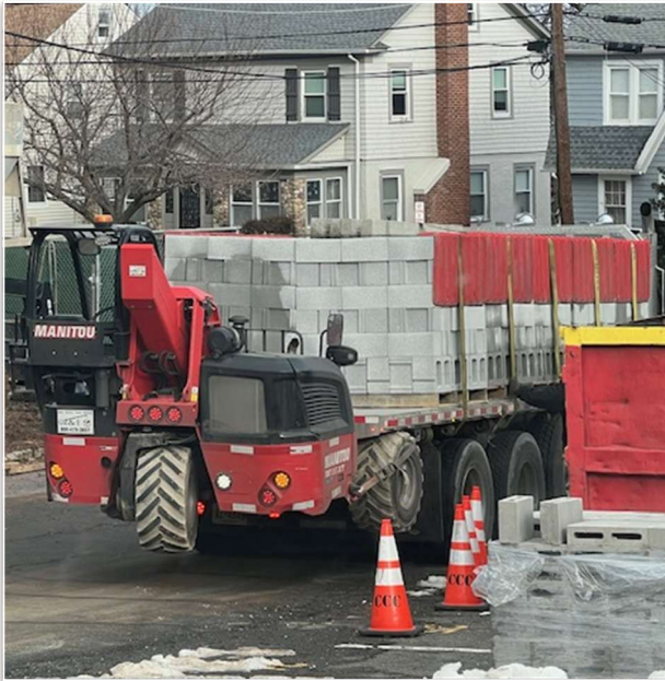
CMU deliveries at KRS
