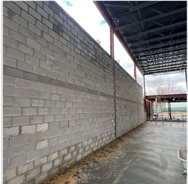
CMU installation at CAS
