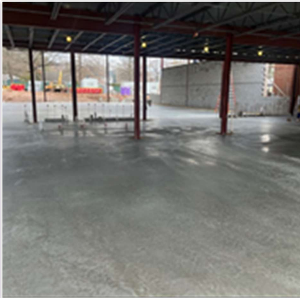
Slab on grade at CAS
