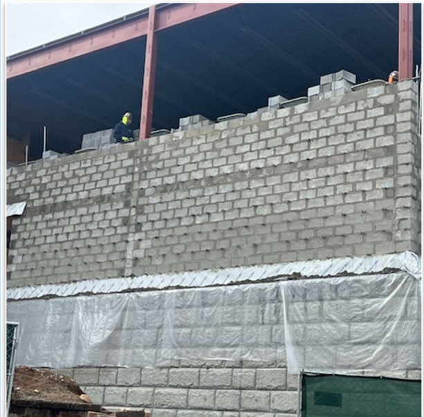
CMU installation at KRS
