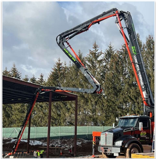
Concrete pump truck at CAS
