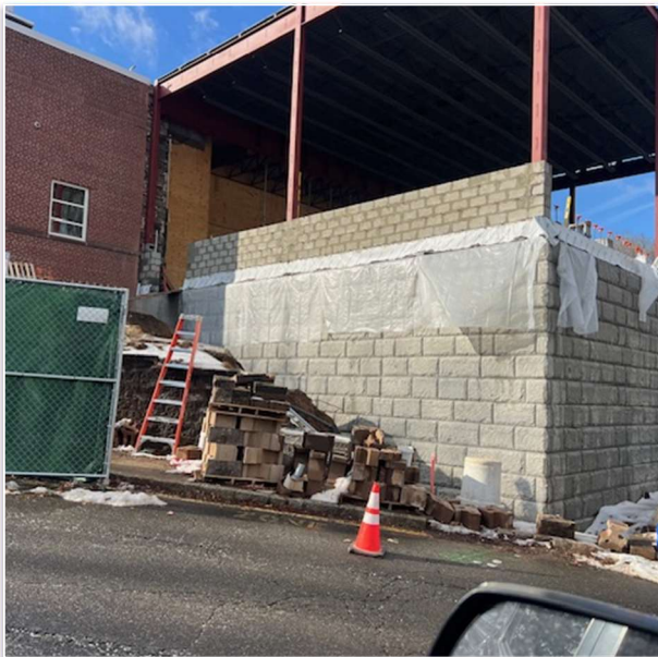
CMU preparation and protection at KRS
