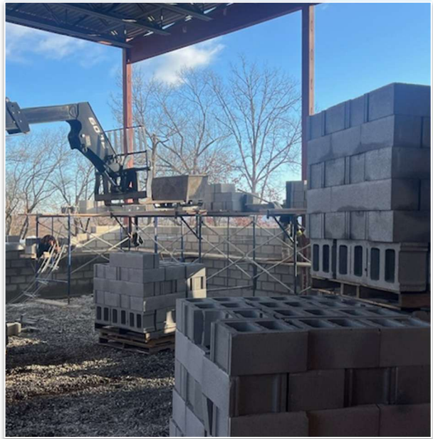
Scaffolding and CMU preparation at KRS
