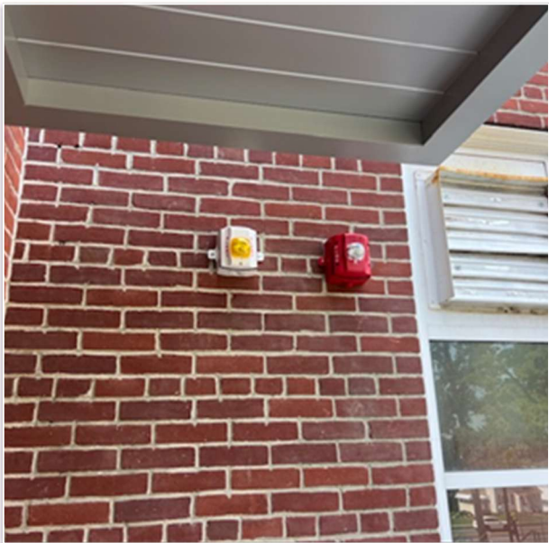
Fire Equipment Replacement at KRS
