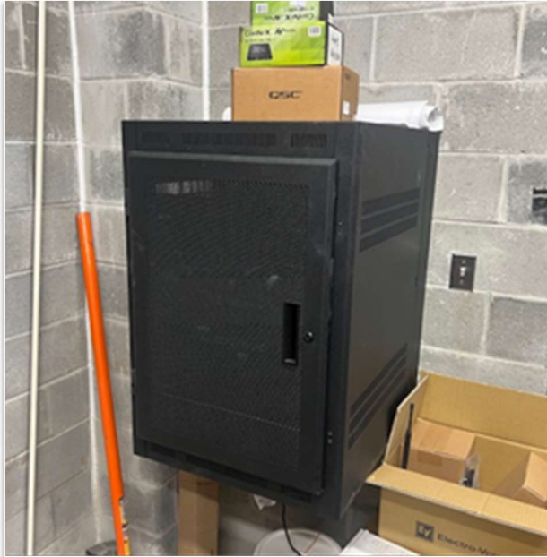
Audio Equipment installation at CAS
