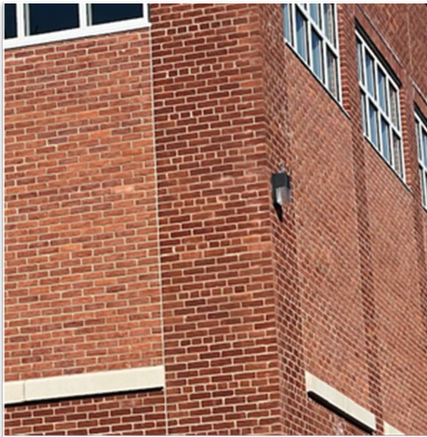
Exterior Lights Installation at KRS
