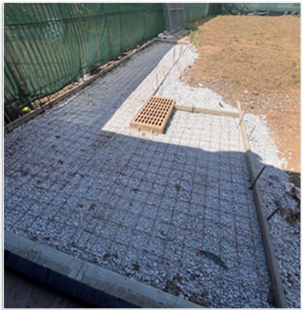
Concrete sidewalk Placement at CAS
