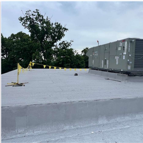
Transition Roofing at KRS
