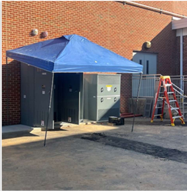
Electrical Switchgear Work at CAS
