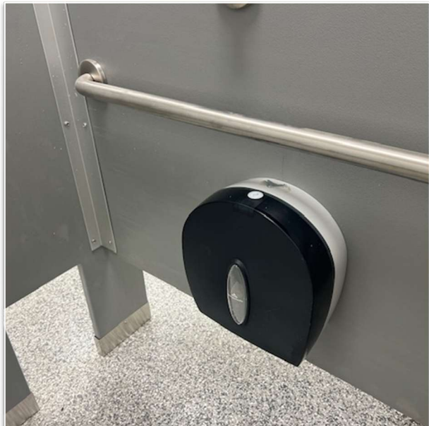
Bath Accessories Installation at CAS
