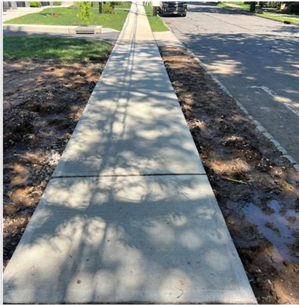
Sidewalk Replacement Work at CAS
