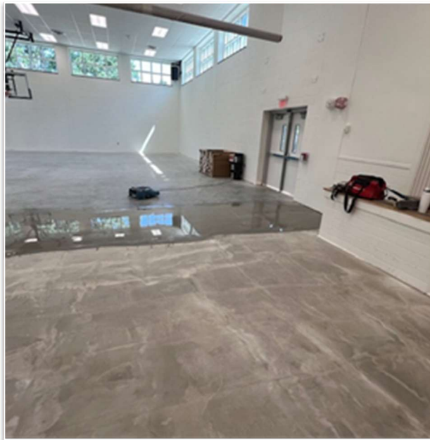
Flooring preparation at KRS
