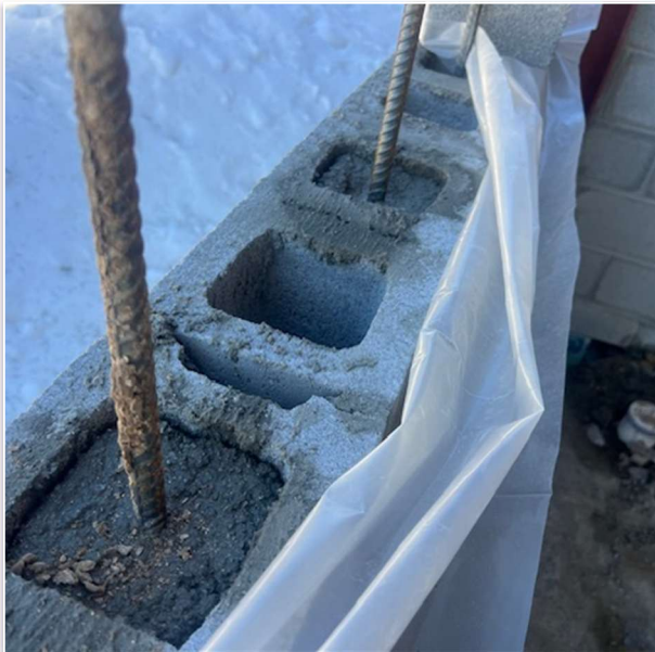
Grout and rebar placement at CAS
