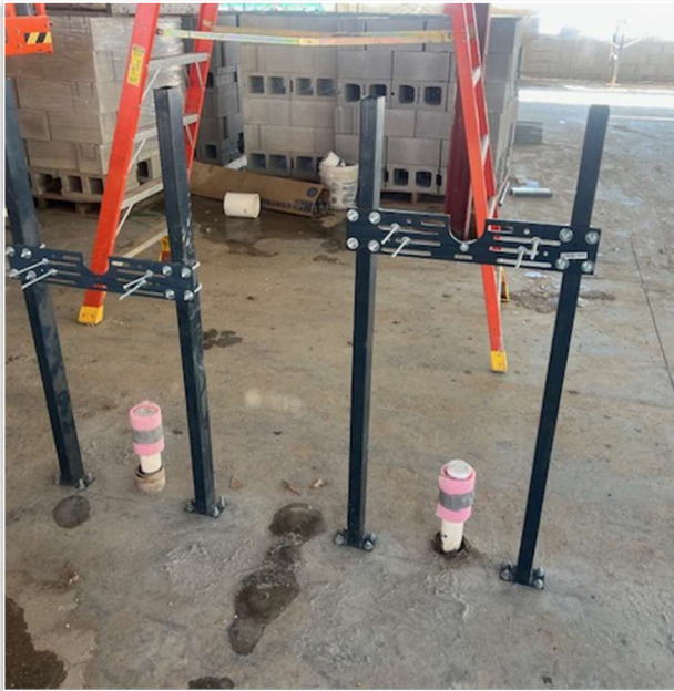
Lavatory racks installation at CAS
