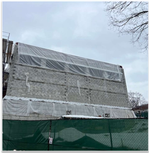
Plastic sheeting Installation at KRS
