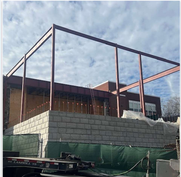
Steel erection at KRS
