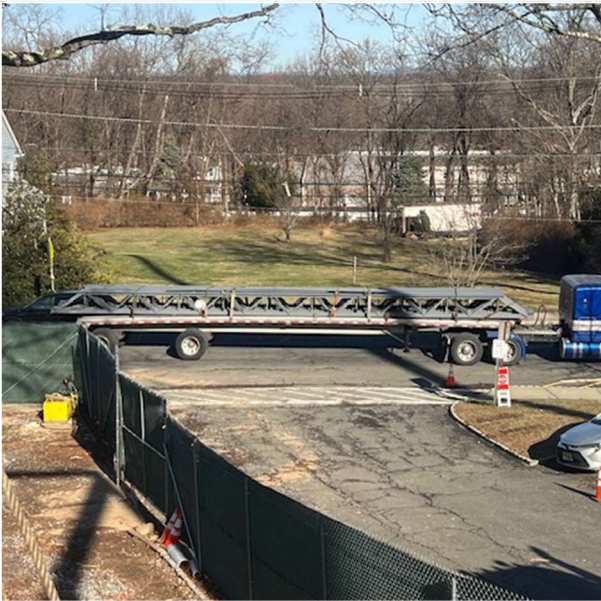
Steel/truss deliveries at KRS
