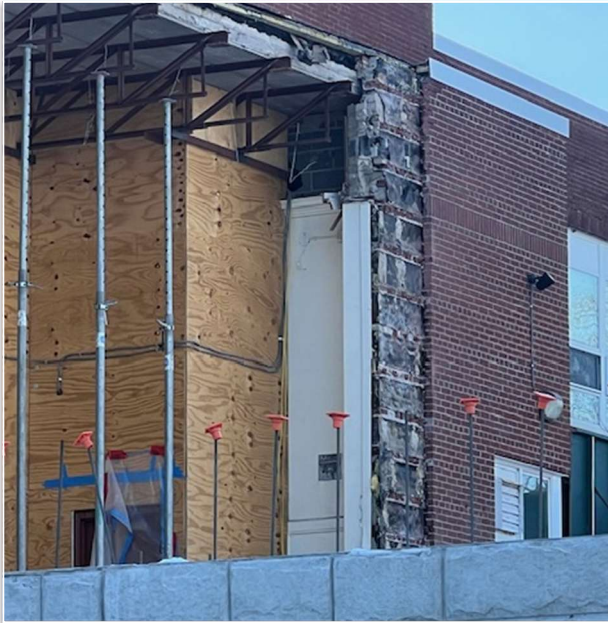
Exterior wall demolition at KRS
