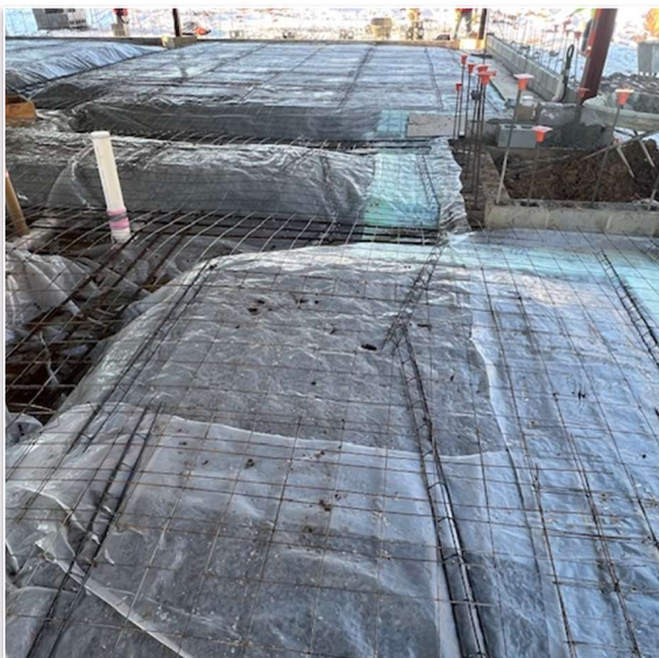
Rebar/ wire mesh at CAS
