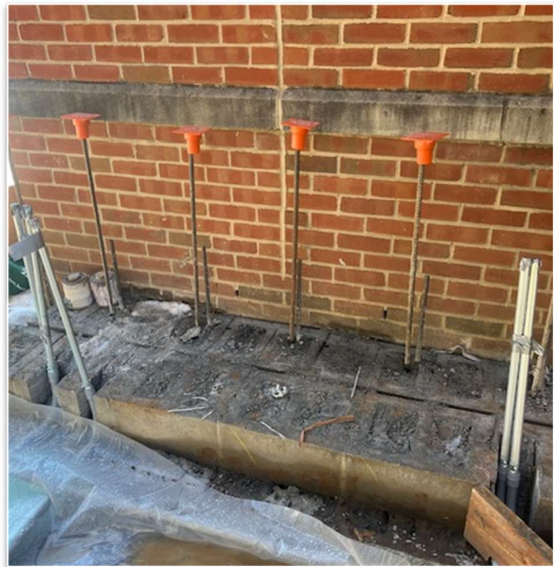
Electrical stub ups at CAS
