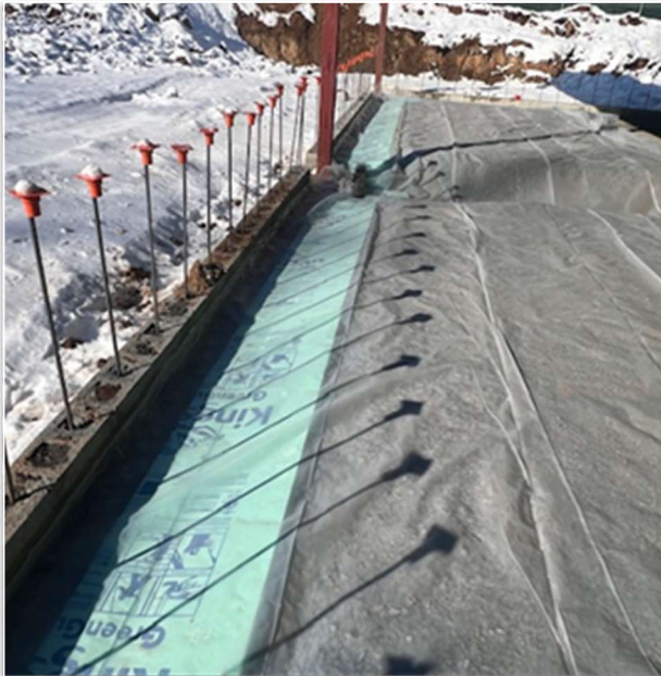
Rigid insulation installation at CAS
