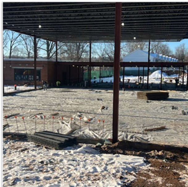
Vapor barrier installation at CAS
