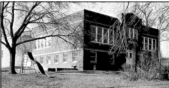
Rantoul School Building
