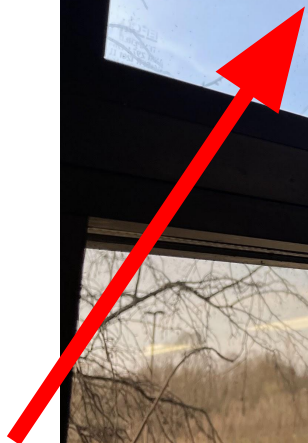
On the Right- Prairieview window example-failed thermal window seal.
