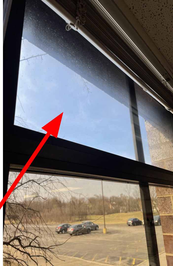
On the Right- Prairieview window example-failed thermal window seal.
