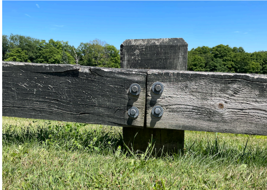
Photo 2: Typical post and rail connection showing rail overlap and lag screw installation.
