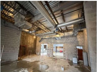
Installation of duct work in kitchen
