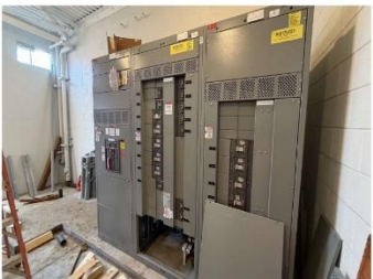
Installation of switch gear in main electric room
