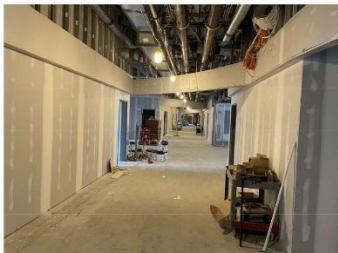
Drywall installation in Middle School wing
