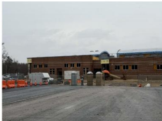
Installation of standing seam barrel room has begun
