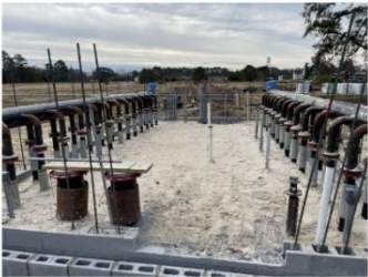
Pump House slab-on grade prep
