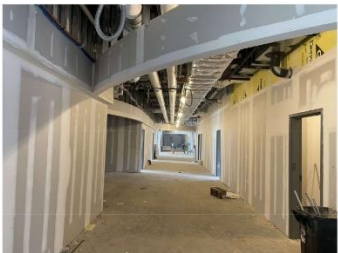
Drywall installation in Middle School wing
