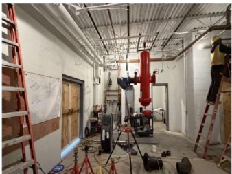
Installation of equipment in main mechanical room
