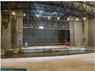
Framing for the stage opening
