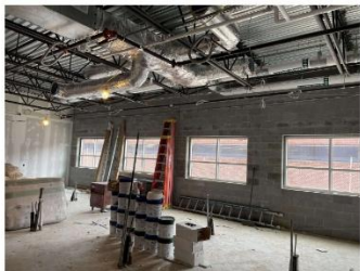
Duct insulation above ceiling in Middle School wing
