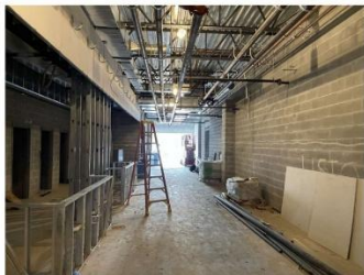
Installation of above ceiling mechanical piping
