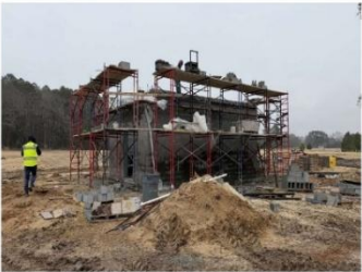
Installation of pump house exterior walls
