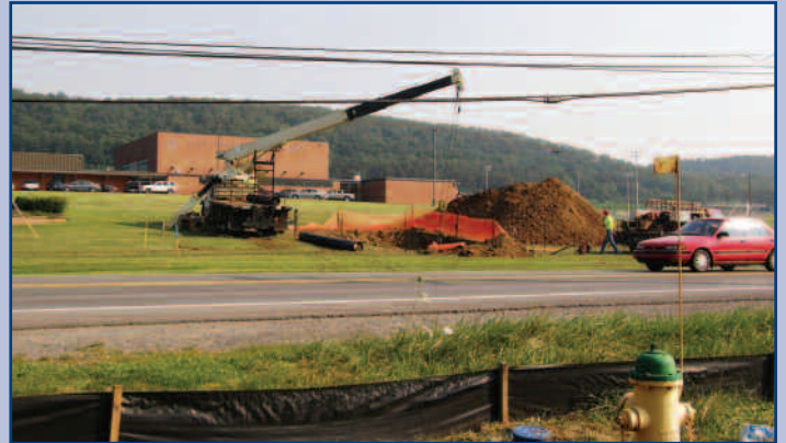
Workers relocate utilities in front of the Bald Eagle High School.
