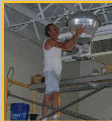
Chris Park from BEA maintenance replaces a light in the high school wrestling room.
