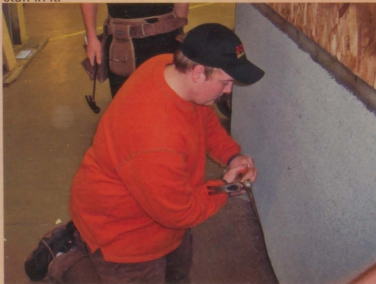
Keith Lounds is working on the wall that Jorden and Joe had constructed earlier. He's putting the finishing touches on it.
