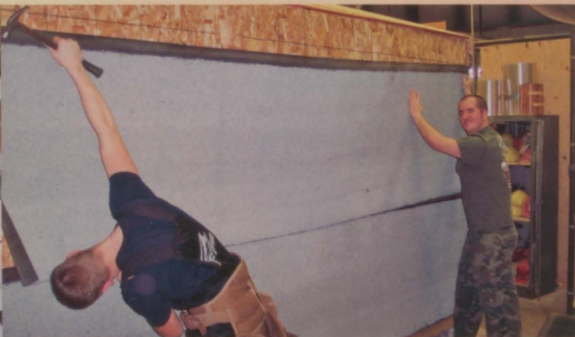
Jorden Mayer and Joe Meehan are busy working at the Construction site located in the Skill Center. Joe jocularly comments, "It takes studs to build a house."
