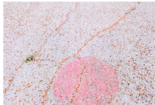
Closer View of Asphalt Surface
