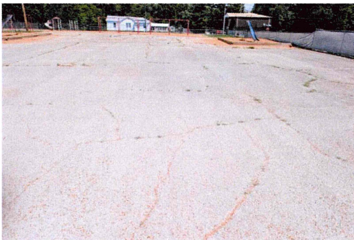
Surface Looking North
