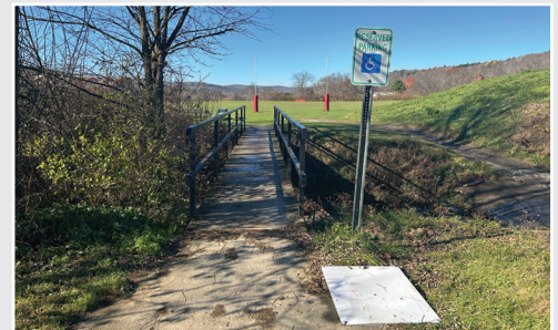
Footbridge access that remains difficult for those with mobility needs.
