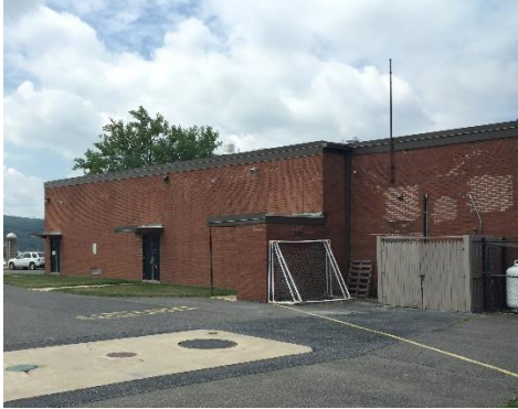
Detail of existing brick
