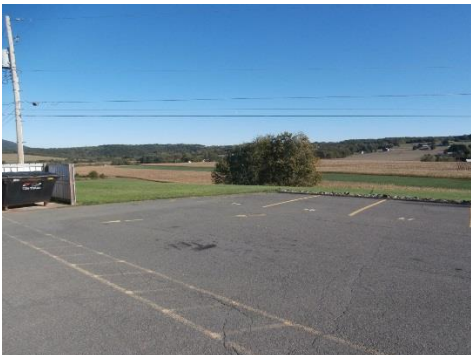
Looking east at paving (note rock lined stormwater facility behind curb at right)
