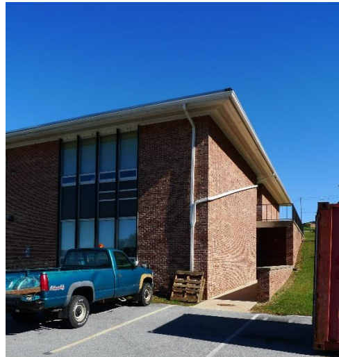
Downspouts and exterior glazing
