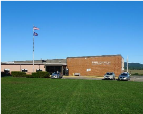
Exterior of building
