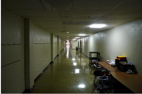
Lower level ceiling and original flooring
