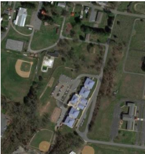
Aerial view of site
