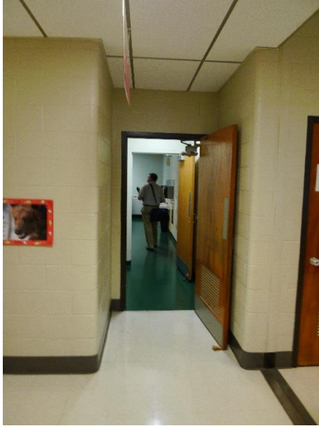
Approach to restroom
