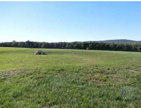
Stormwater management basin
