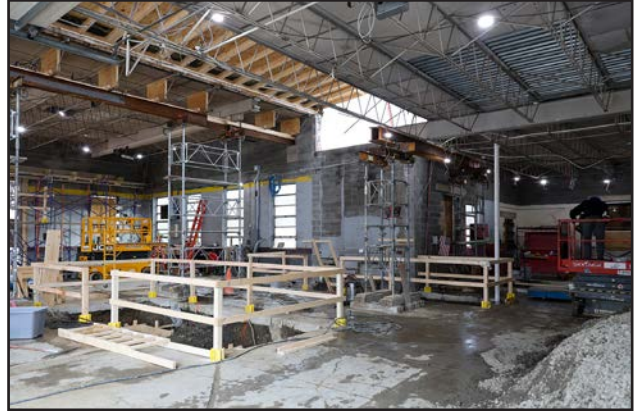
Below: Bus garage renovations are underway.
