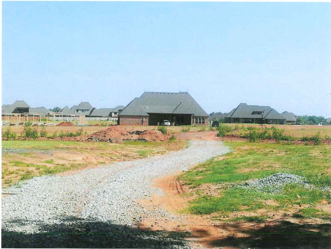
Looking northward into what will become Magnolia Trace 6 along existing construction entrance
