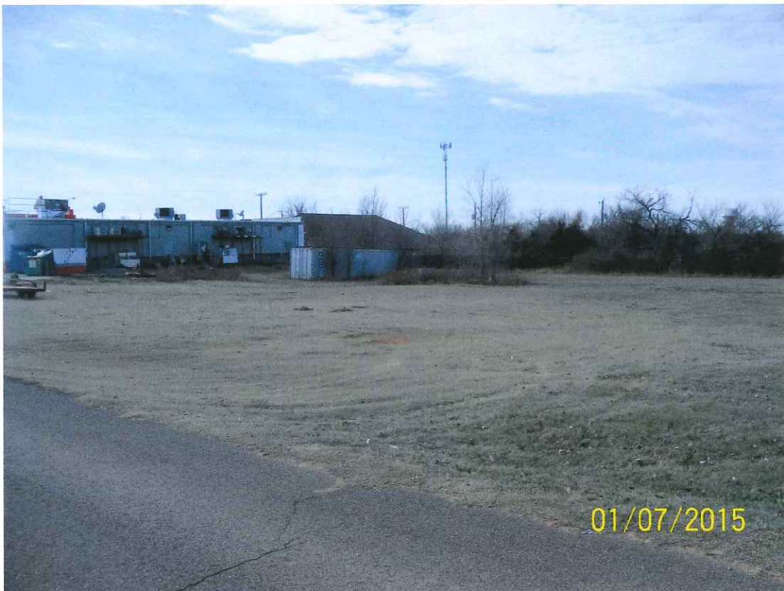
View from Northeast on N. Pine Terrace
