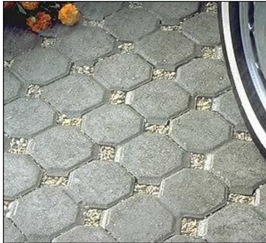
Figure 3 – Open-Jointed Paving Block
