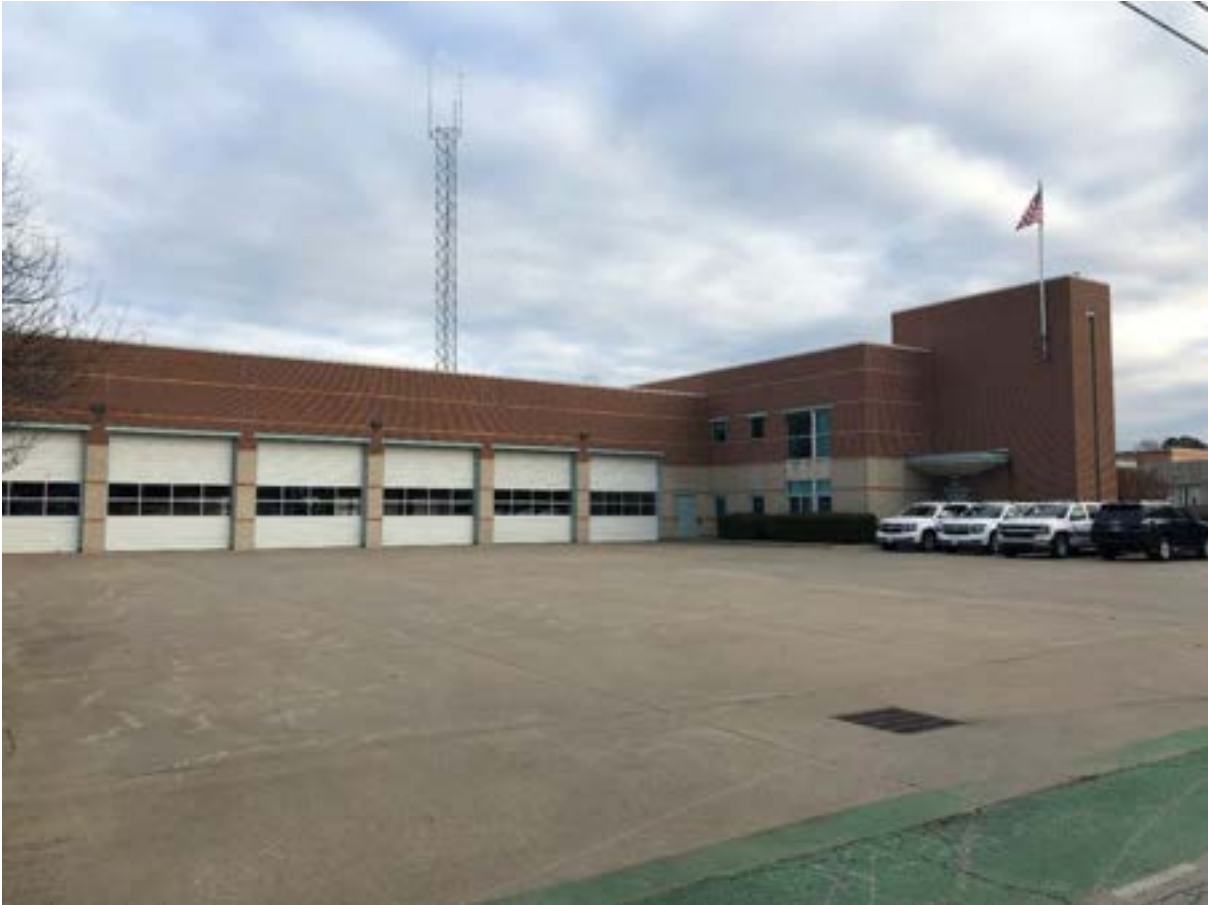
Figure 40- Station 1, Fire Administration
