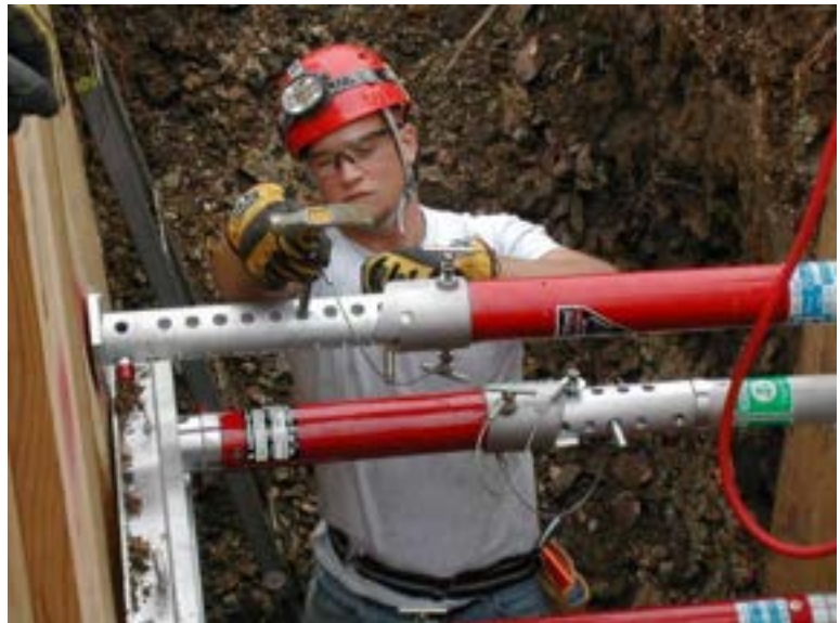
Figure 6- Early Trench Rescue Training
