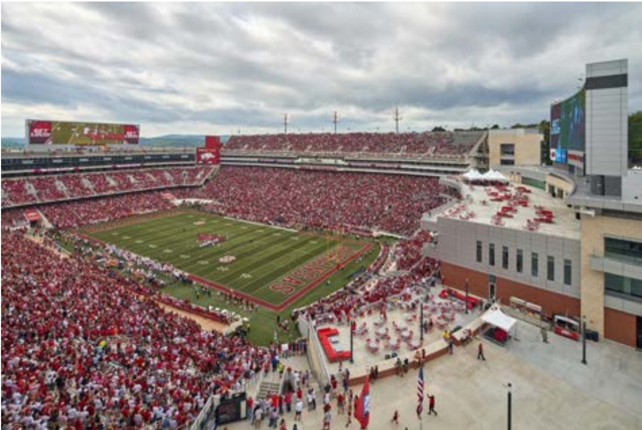
Figure 26 - Reynolds Razorback Stadium, UofA Fayetteville
