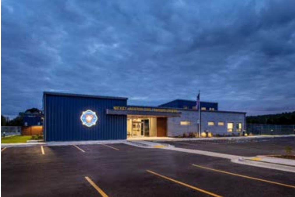
Figure 31 - Training Division Offices and Classroom Building at MJTC/2022 Training Hours
