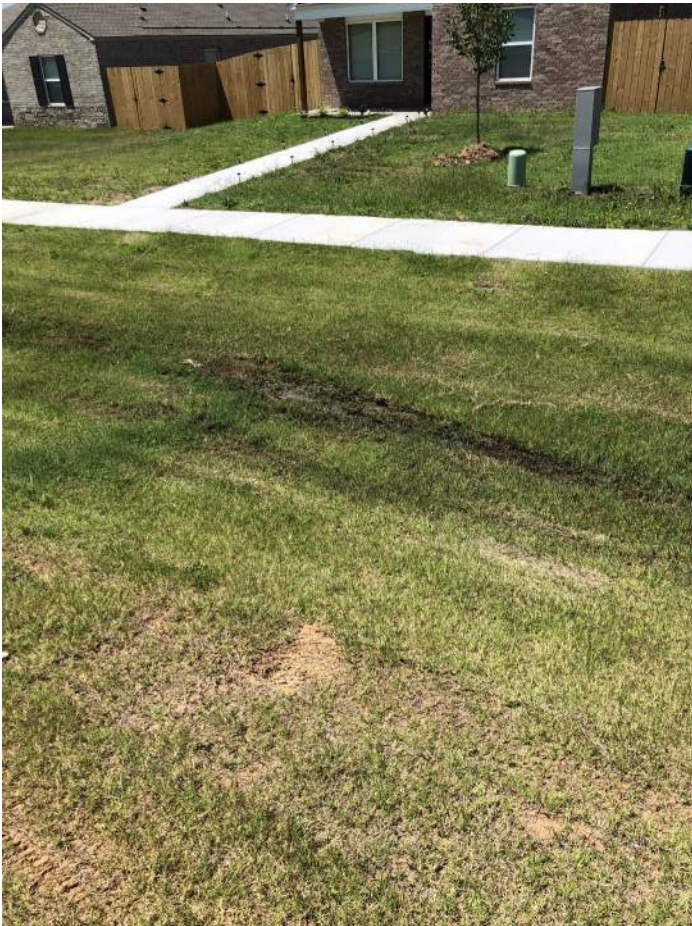
Standing Water - Public Green Space - Detail
