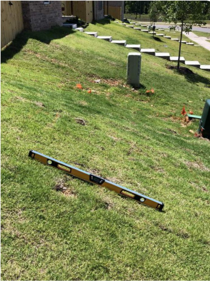
Front Yard Grade
