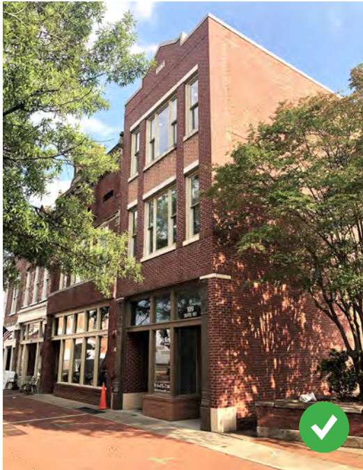
A range of traditional materials are used for this new building, including brick cladding, cast iron pilasters, wooden windows, and concrete lintels and sills.
