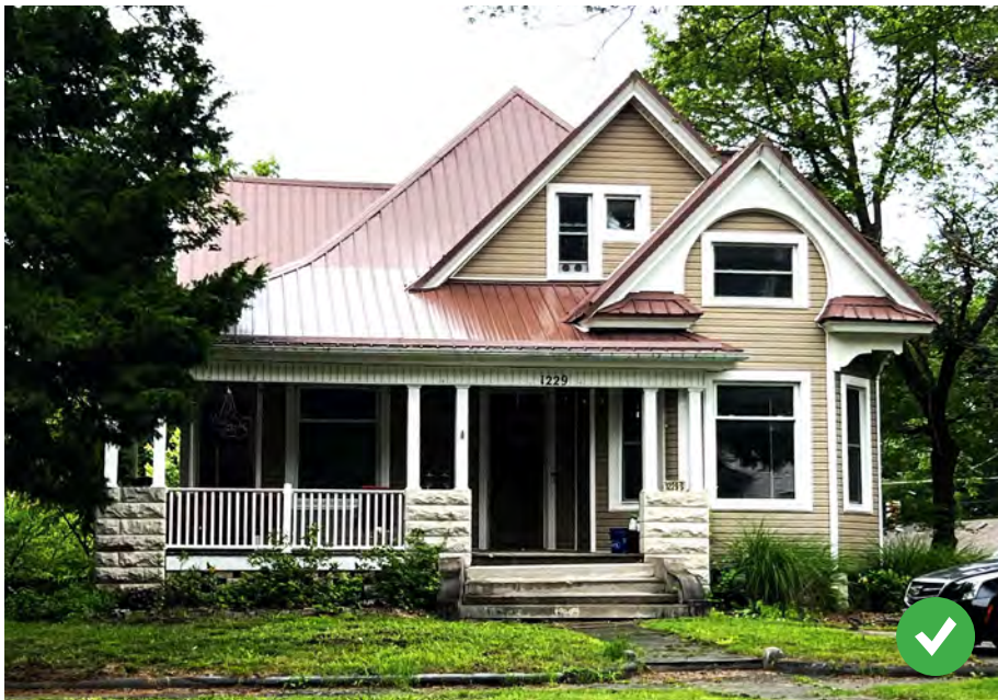
This Folk Victorian house at 1229 South Garrison Street has a non-original metal roof. While metal roofing is not very prevalent for historic houses in Carthage, they would have historically been true standing-seam metal rather than the V-crimp metal roof on this house, which only approximates the standing-seam roof type.
