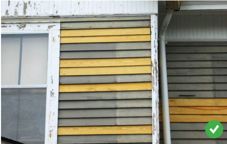
Although this exterior wall still needs repainting, these new clapboards match the originals with respect to their exposure width and other characteristics
