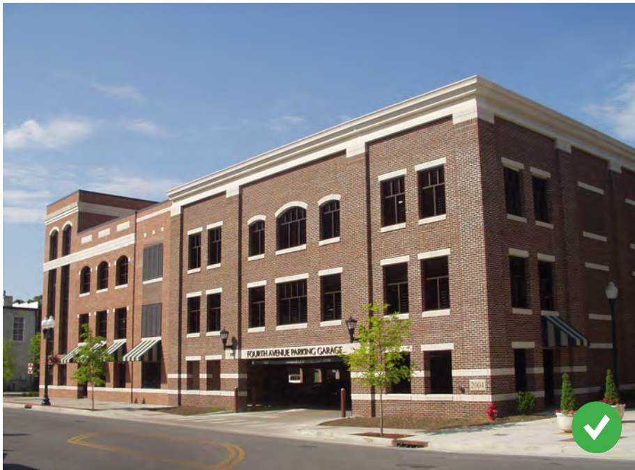
This parking garage does not include ground floor retail because it is not on a segment of a Downtown street featuring that use. However, it fits in nicely with a historic Downtown based upon its scale, orientation to the street, materials, and the size, orientation and rhythm of its openings.
