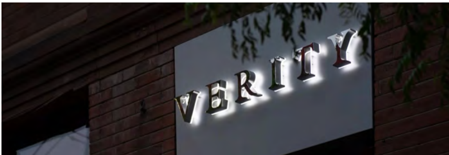
This back-lit sign features lighting that illuminates the letters of the sign but not the entire sign.
