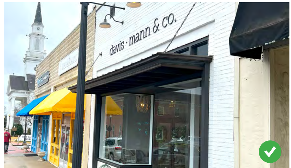
This canopy from another community is located above the main entry of the building and supported by hanger chains.
