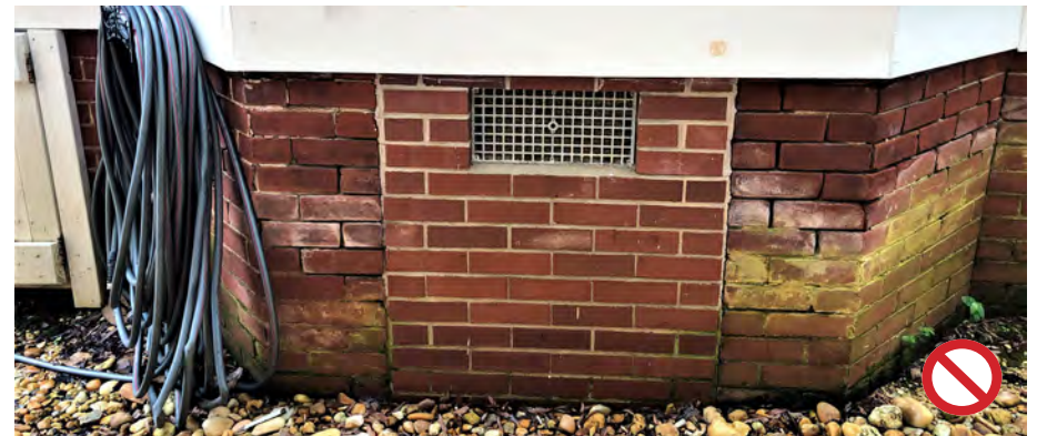
The design of the brick infill between the historic brick piers is inappropriate. If permitted, it should be recessed.
