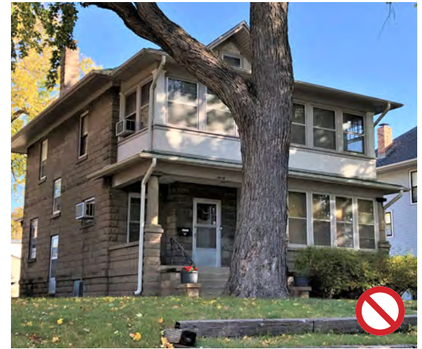
The enclosed upper and lower floor porches are an inappropriate alteration.
