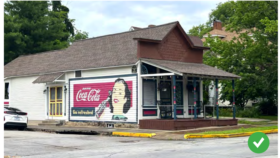
This mural on a commercial building at the intersection of S. Garrison Ave. and Pine St. is located on a blank portion of the facade and does not obscure architectural features.
