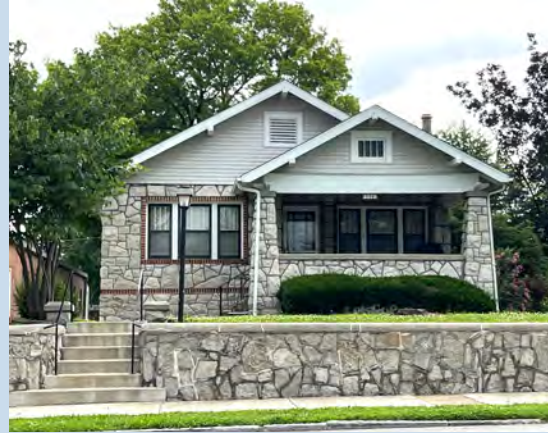
RUBBLE STONE WALL WITH CONCRETE CAP & STEPS
