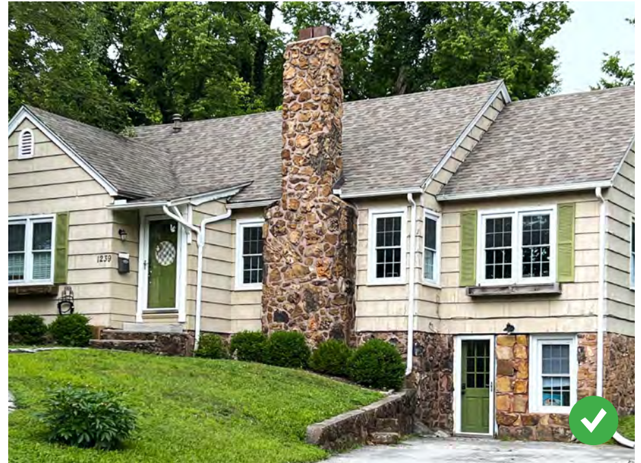
The massive rubble stone chimney on this mid-20th century cottage is a character-defining feature. Located on Grand Avenue in the South Carthage Historic District, it utilizes the same stone as the house's foundation.
