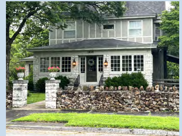
RUBBLE STONE WALL WITH ASHLAR PIERS
