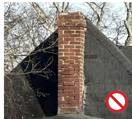
Above left: The lower half of this brick chimney is missing mortar, making it vulnerable to collapse during high winds.
