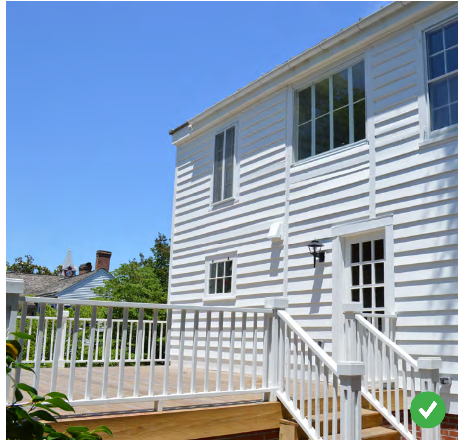
This deck from another community is a good example of a rear addition.
