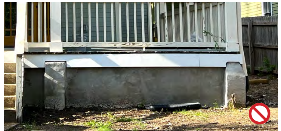
This house's brick foundations have been parged with concrete, which alters the historic appearance and traps in moisture that can lead to future deterioration.
