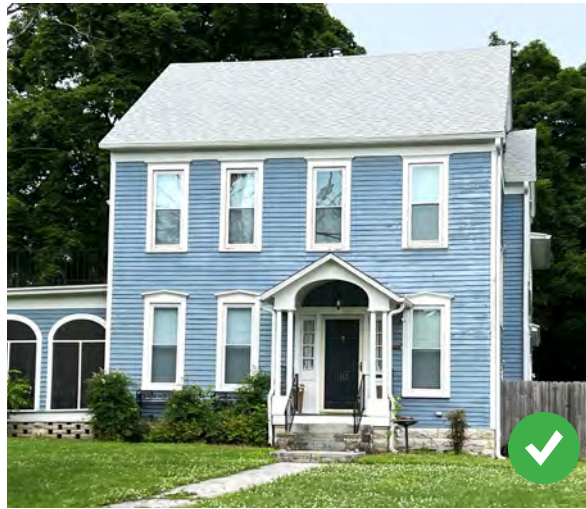
This two-story frame house from the late-19th or early-20th century is located at 1113 South Grand Avenue. The front door's sidelights and portico provide a Colonial Revival styling.
