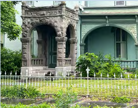
DECORATIVE IRON FENCE WITH THIN BALUSTERS
