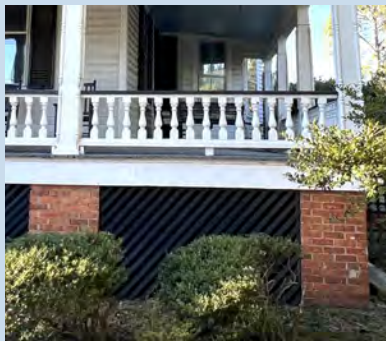
BRICK PIERS WITH WOODEN LATTICEWORK
