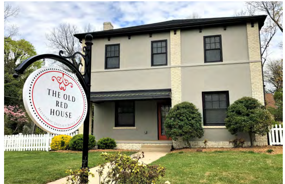
Above: This free standing sign is appropriate.
