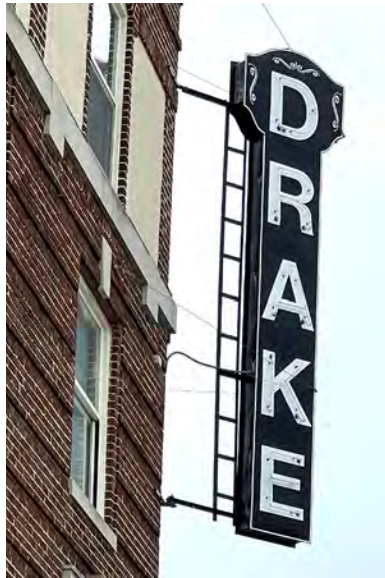
The sign on the former Drake Hotel is historic and should be preserved.
