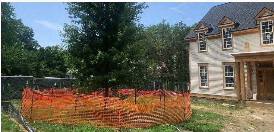
This photo from another community illustrates proper fencing to protect an existing tree from damage during construction.
