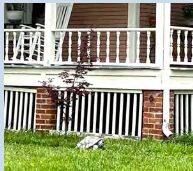
BRICK PIERS WITH VERTICAL WOODEN SLATS
