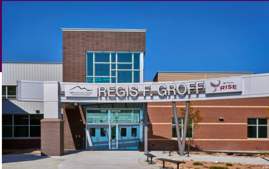
CONSTRUCTION TO COMPLETION
