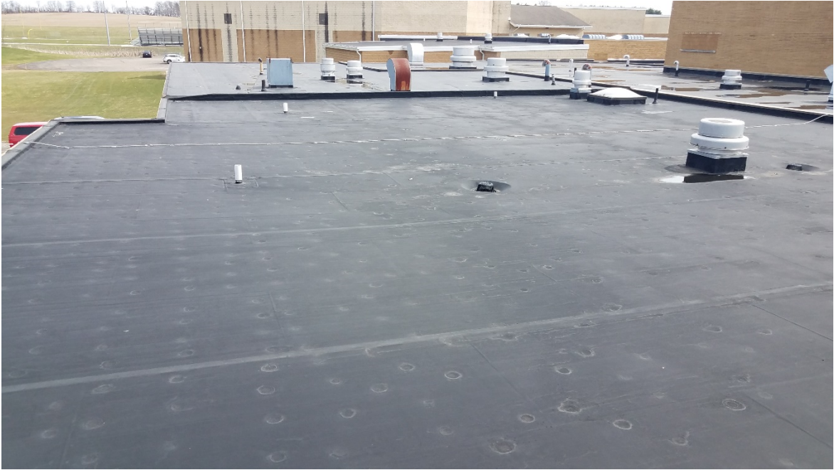
Roofing at High School
