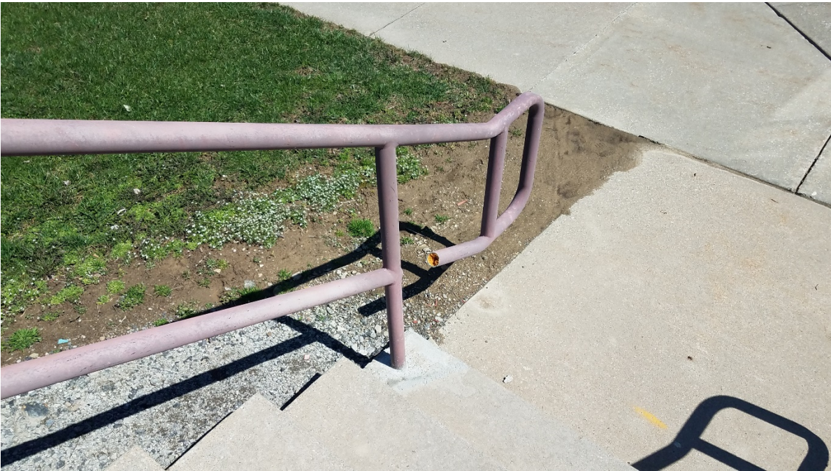
Handrail at Front Parking Lot
