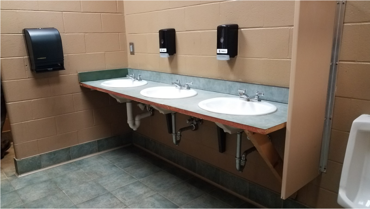
Lavatory Counters in Toilet Rooms
