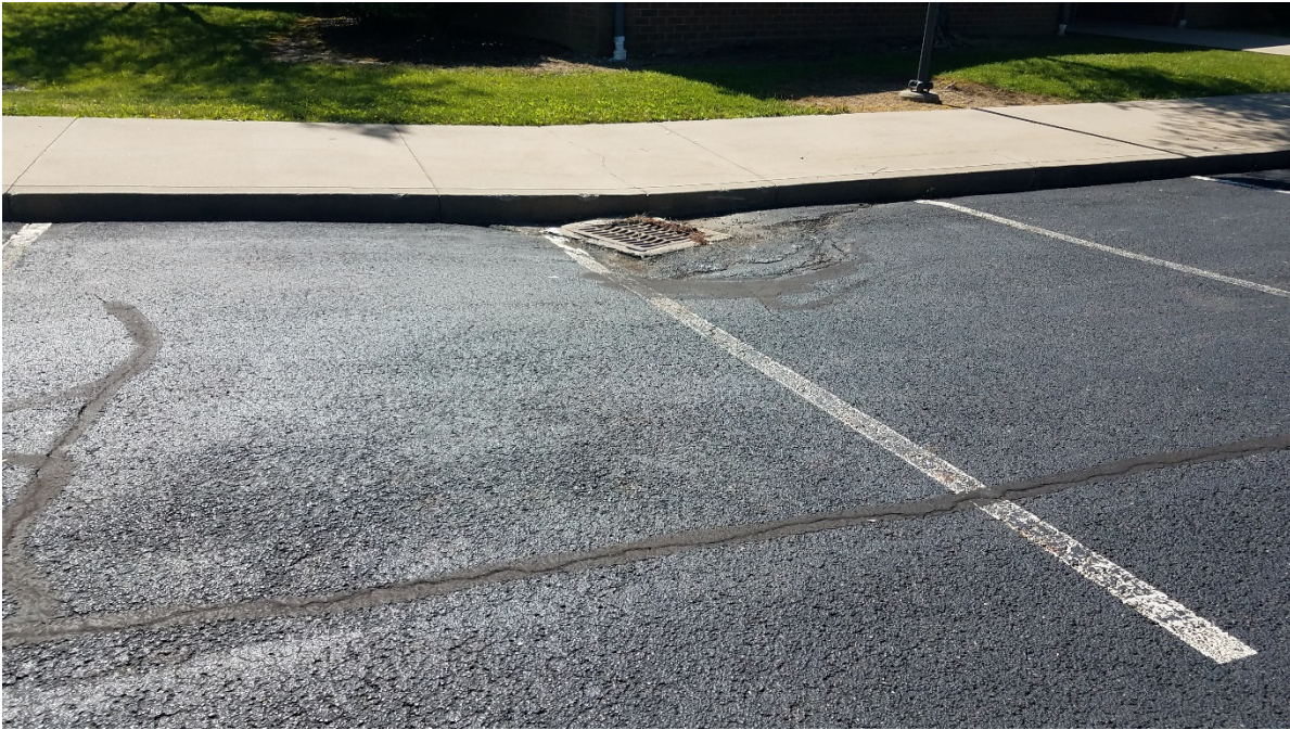
Paving at Parking Lot
