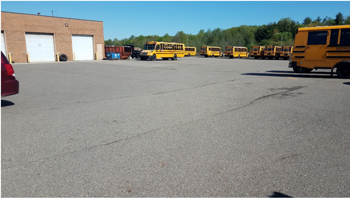
Paving Condition on Site
