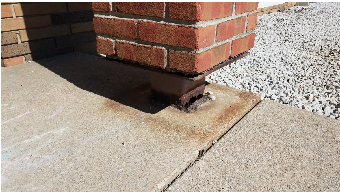
Column Base at Entry Overhang
