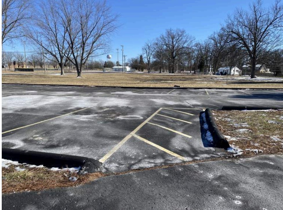
Area E - Looking south. Asphalt rolled curb
