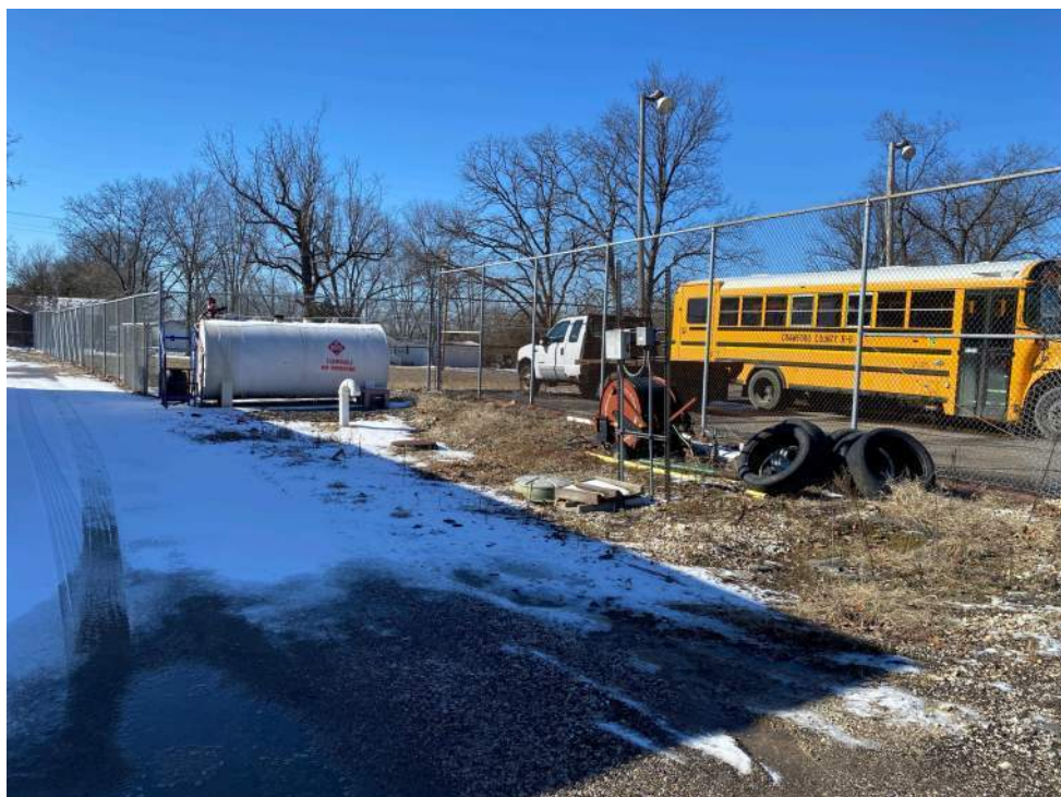
Bus Facility - North elevation looking west.
