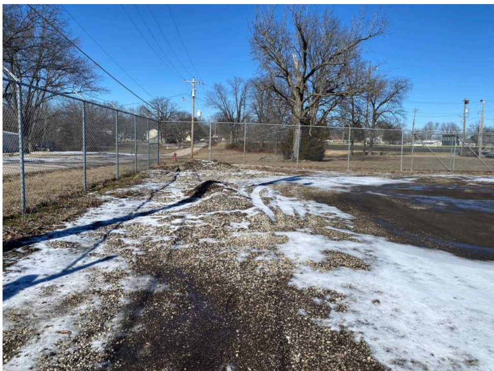
Bus Facility - West end of parking lot looking North
