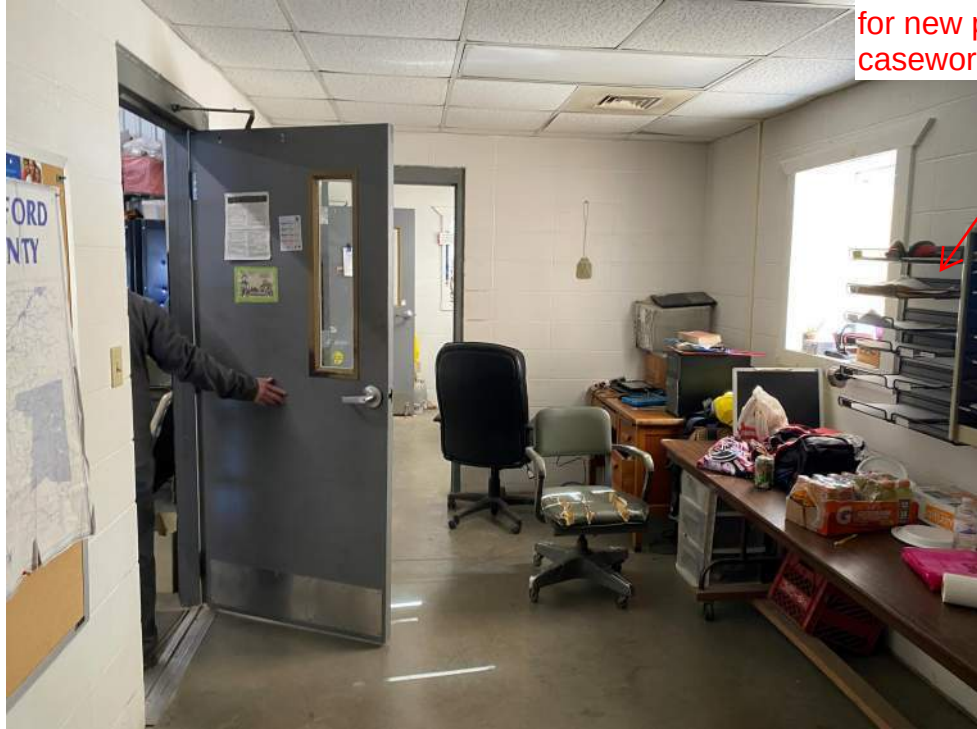
Bus Facility - Breakroom
