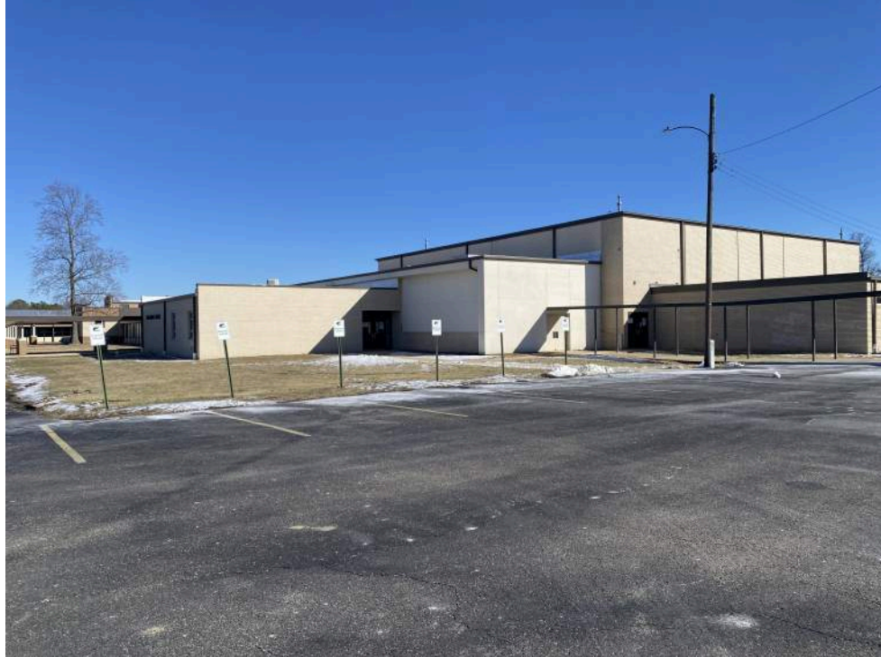
Area C - Looking east from the High school towards Middle school.
