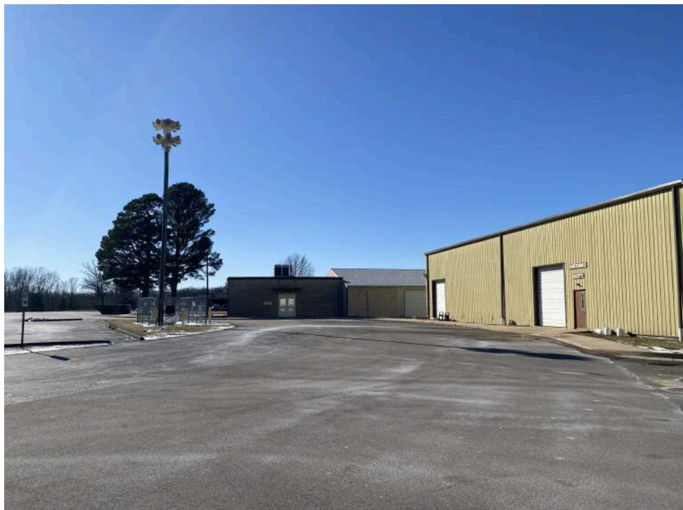
Area E - Looking west. Maintenance building is on the right side of photo
