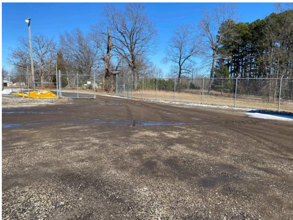
Bus Facility - Looking Northeast at vehicle gate.
