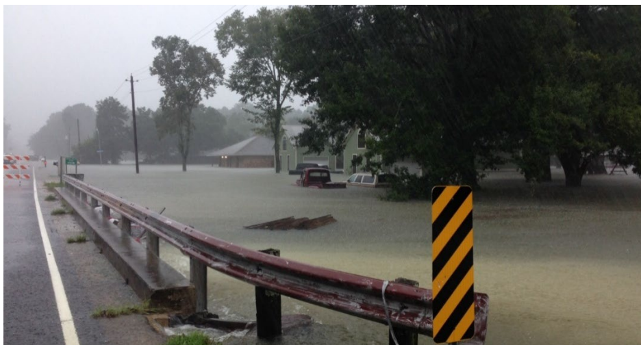
Figure 10. Gurney Road, just east of Centerra Court (looking west) during the 2016 Flood Event
