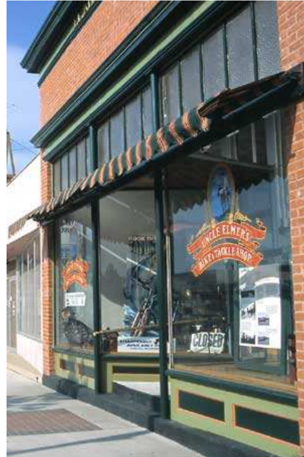
This storefront shows a greater number of voids to solids, and an appropriate bulkhead at the base of the storefront windows.
