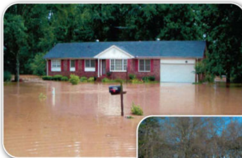
Flooding in Del Norte
