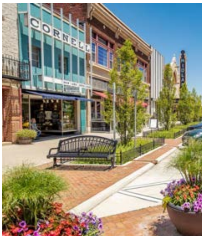
Newark's downtown revitalization included major streetscape transformations that created a more enjoyable and business-friendly environment for pedestrians.
