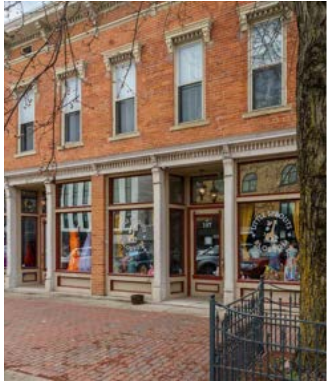
Downtown London's streetscape has many historic details like brick sidewalks and recessed entrances that contribute to its character.
