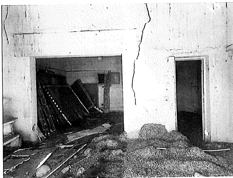
Figure 7 – Interior of Building
