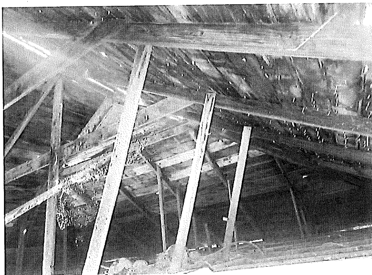
Figure 6 – Roof Framing Condition
