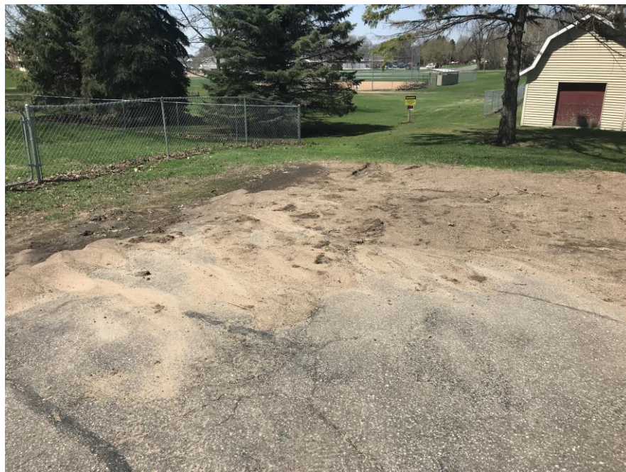
Parking Lot West of Elementary School Building
