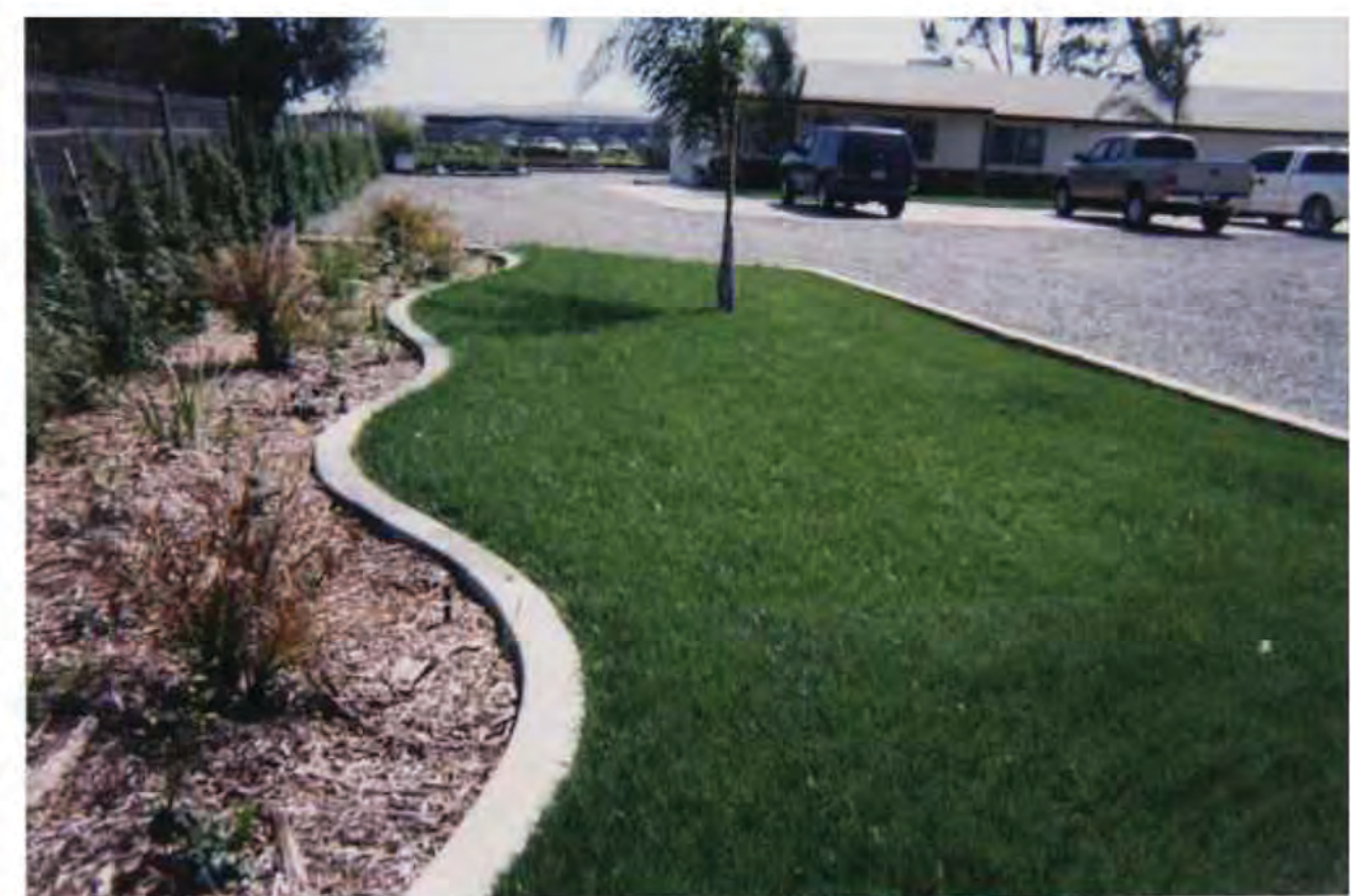
CONCRETE MOW STRIP IN VETERAN'S AREA
