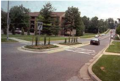
Median Refuge Near Intersection
