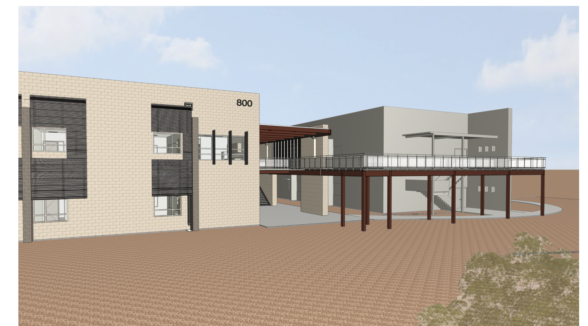
Classroom Building Addition - South View
