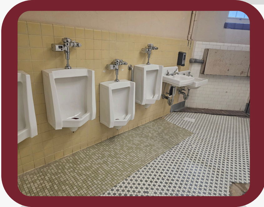
GWMS Basement Bathroom Renovation
