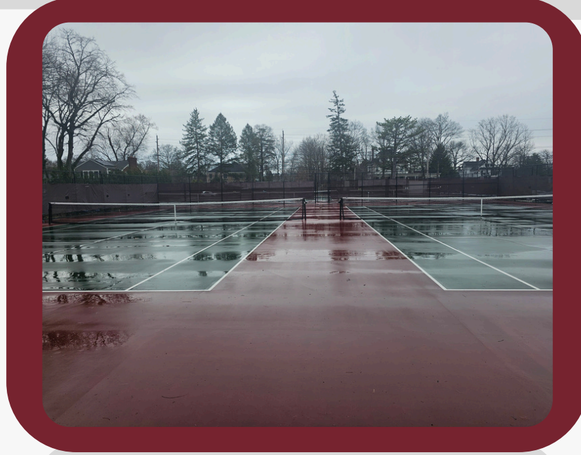
RHS Tennis Court Replacement
