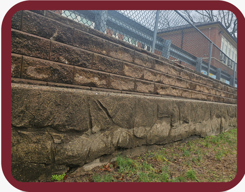
Willard Elementary Retaining Wall
