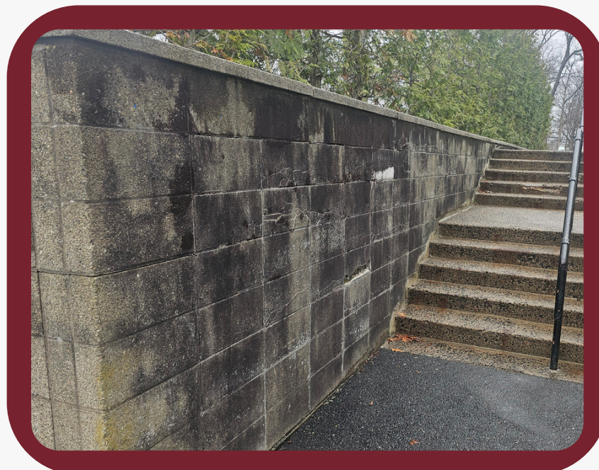
Ridge Elementary Retaining Wall
