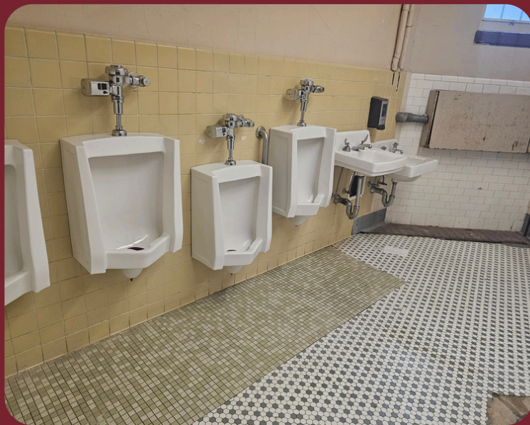
GWMS Basement Bathroom Renovation
