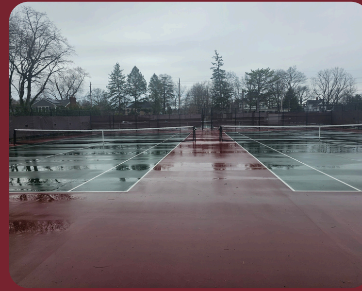
RHS Tennis Court Replacement
