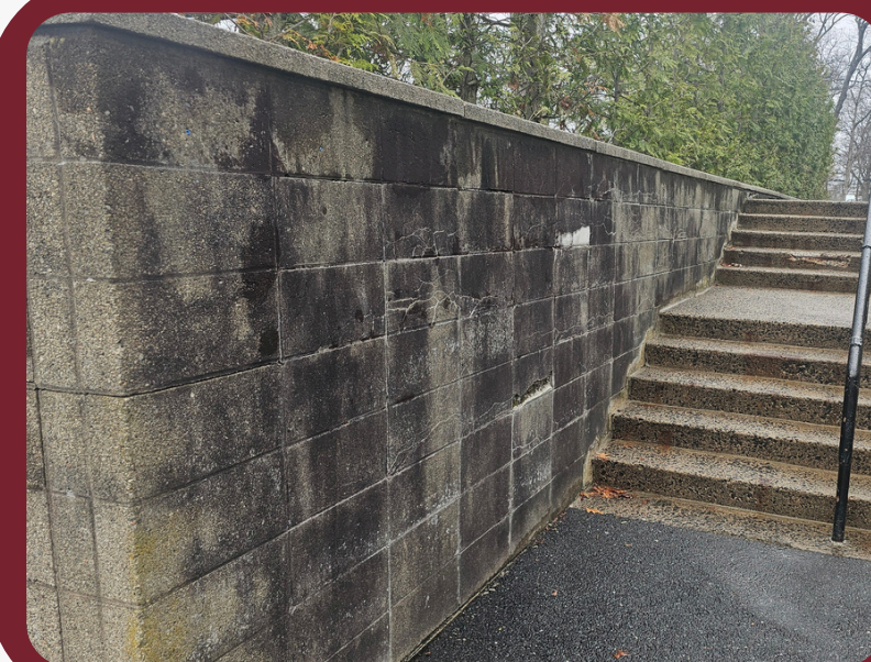
Ridge Elementary Retaining Wall
