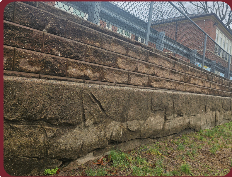
Willard Elementary Retaining Wall
