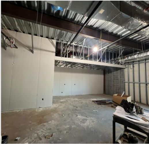
Gantner- First floor sheetrock
