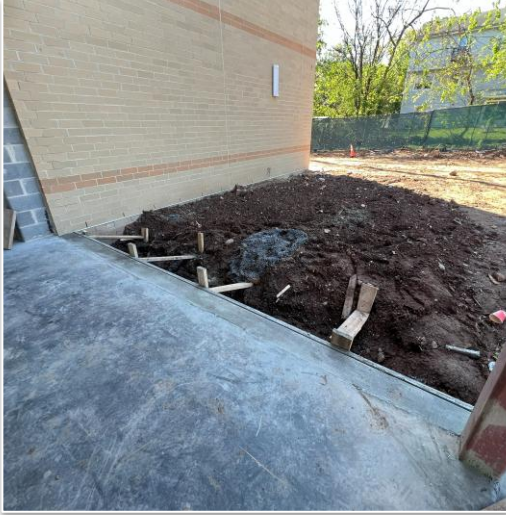
Gantner- Concrete curb for curtain wall
