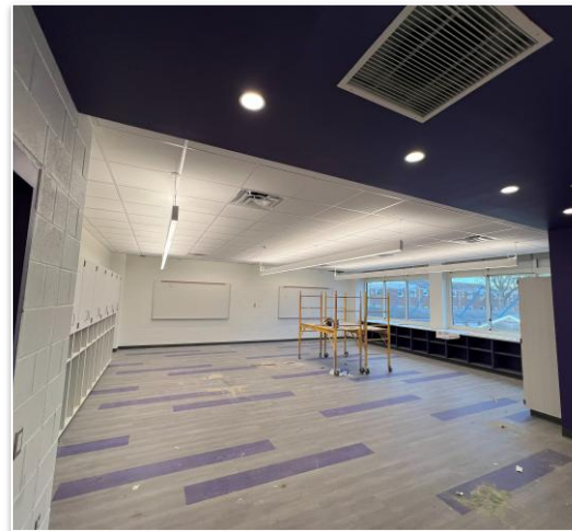
16th- Classroom ceiling
