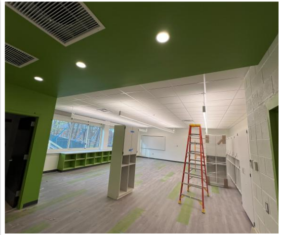
16th- Classroom ceiling
