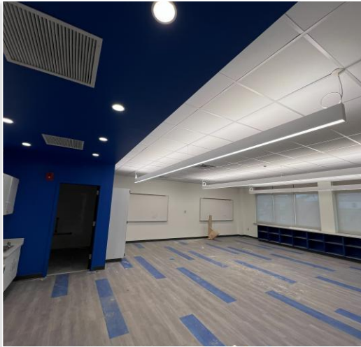
16th- Classroom ceiling
