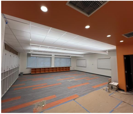
16th- Classroom ceiling
