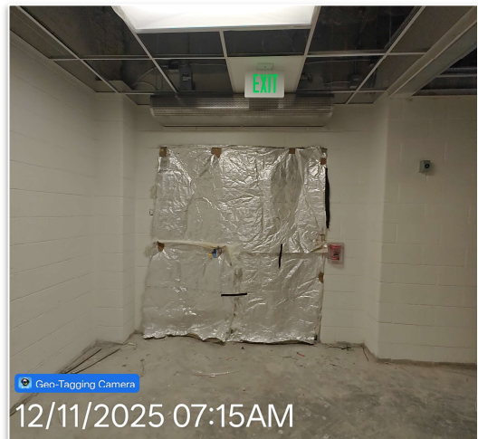
Gilbert- Exit Signs Installed and Heat Curtain Installed
