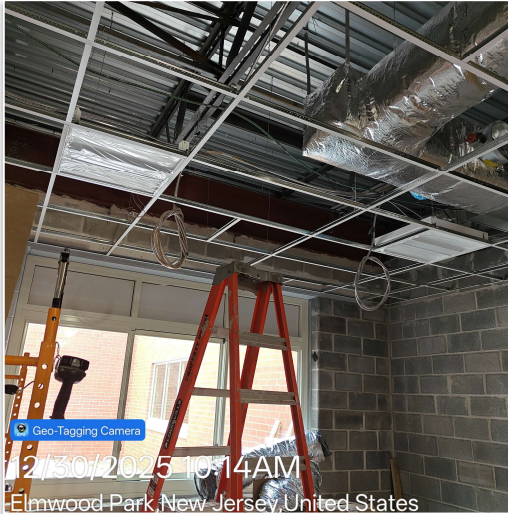
16th- Internal classroom Ceiling grid and lighting
