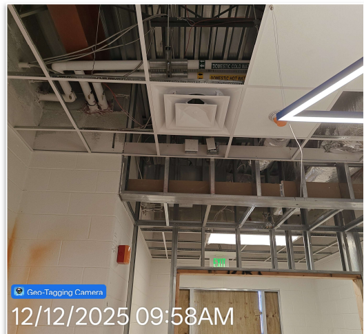
16th- Flex duct and Diffusers Installed
