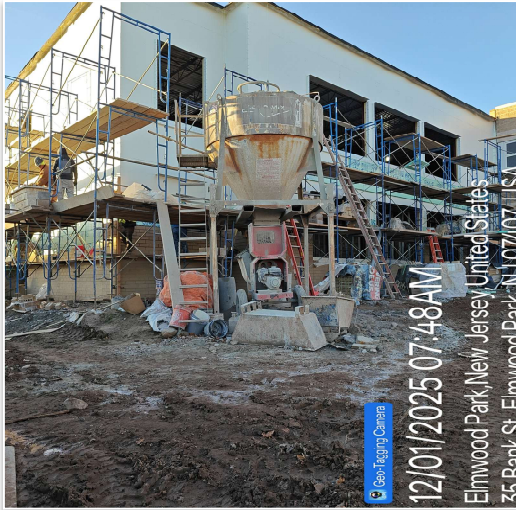
Gantner- Brickwork Continues
