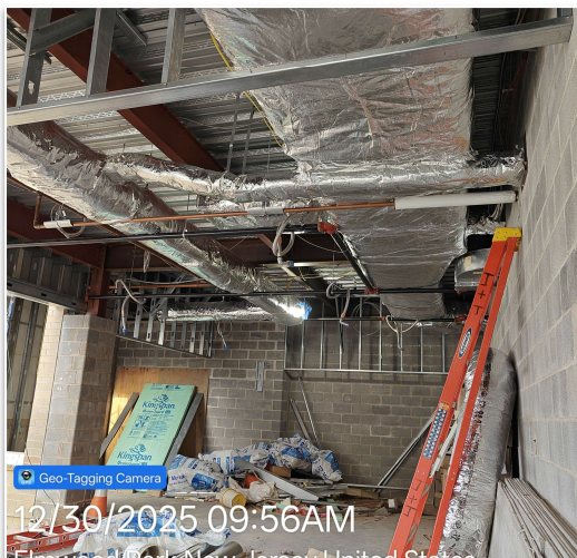
Gantner-Phase I duct insulation Completed
