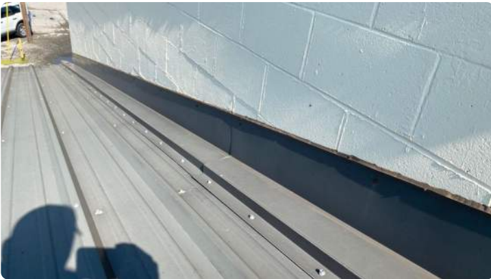
Photo showing condition of the perimeter flashings.
