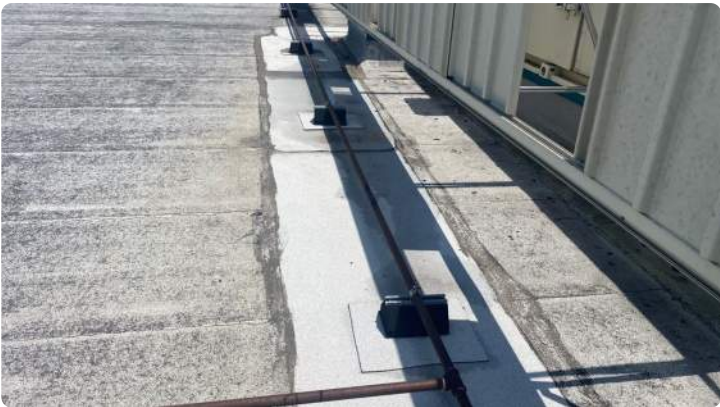
Photo showing area with new Mod Bit under sleepers.
