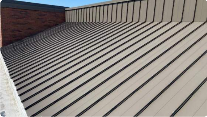
Photo showing condition of the metal awning.
