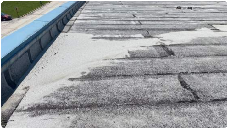
Photo showing granules piled up from deteriorated field.
