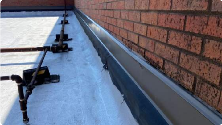
Photo showing condition of the perimeter flashings.
