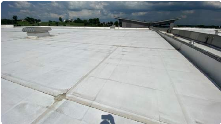
Photo showing additional overview of Area 14 roof.
