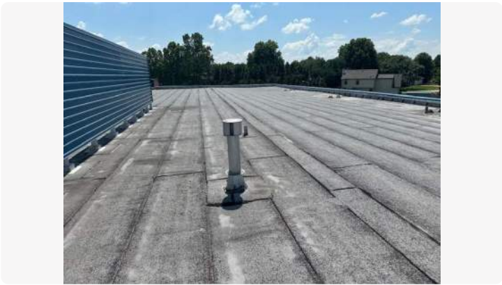
Photo showing overview of Area 08 roof.
