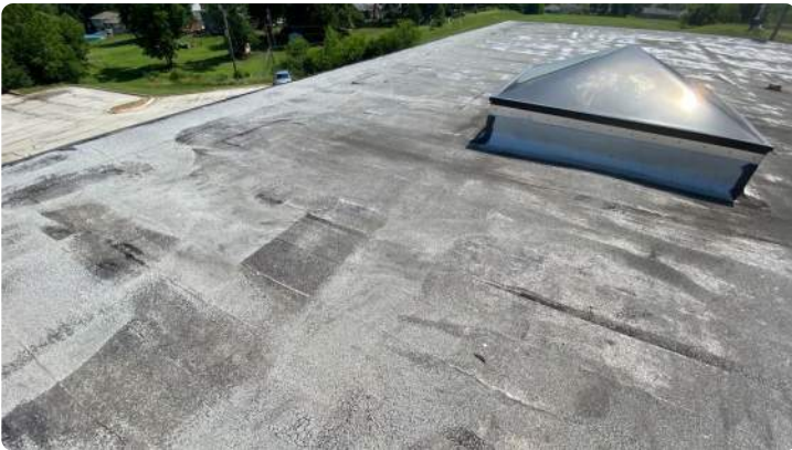
Photo showing additional overview of Area 08 roof.
