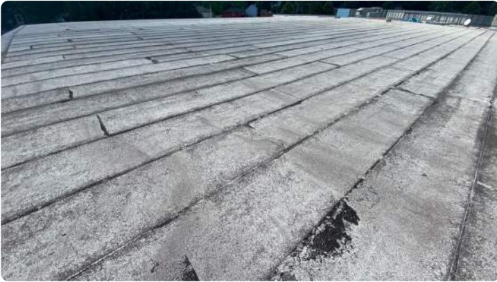
Photo showing overview of Area 02 roof.
