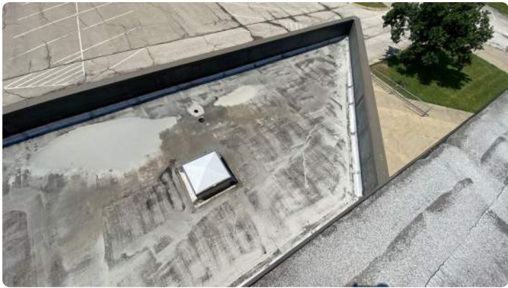
Photo showing additional overview of Area 14 roof.
