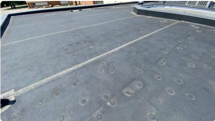
Photo showing overview of Area 09 roof.
