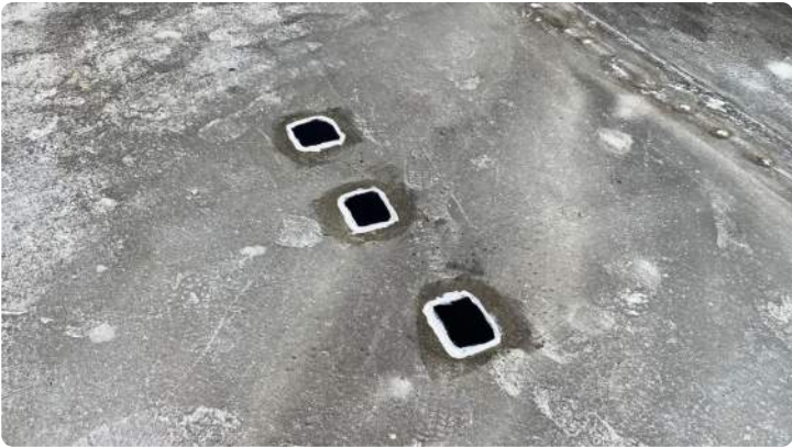
Photo showing repairs made to the field membrane.
