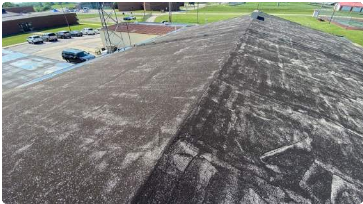
Photo showing additional overview of Area 04 roof.
