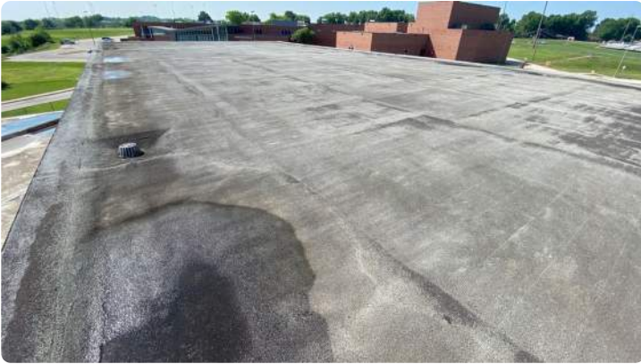
Photo showing overview of Area 04 roof.
