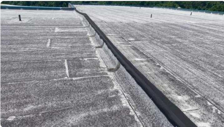
Photo showing condition of the expansion joint.
