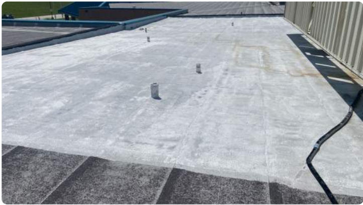
Photo showing section of roof that was previously coated.
