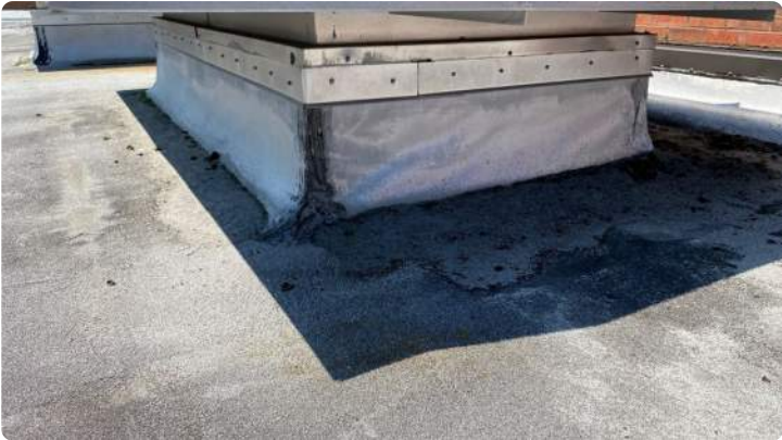
Photo showing condition of the perimeter flashings.
