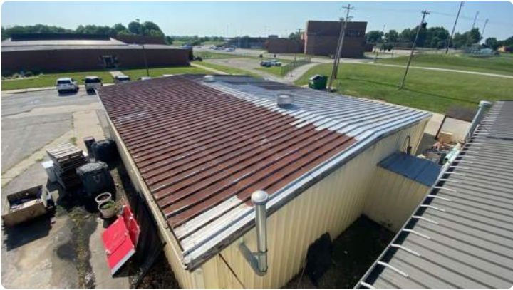
Photo showing overview of Area 06 roof.
