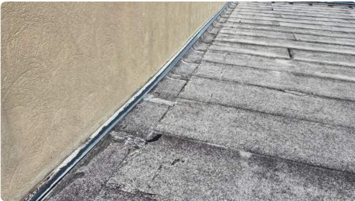
Photo showing condition of the perimeter flashings.
