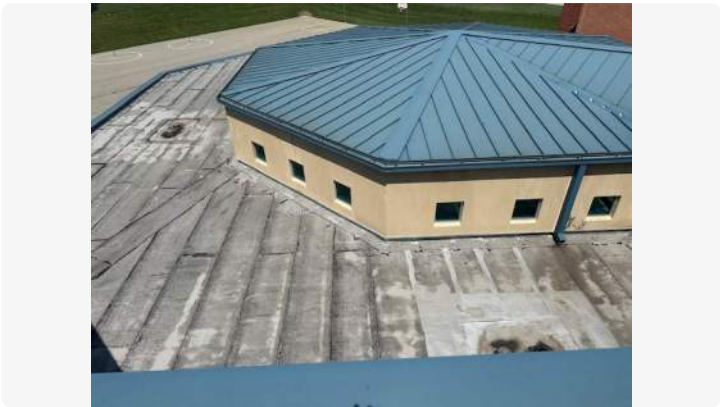
Photo showing overview of Area 07 roof.
