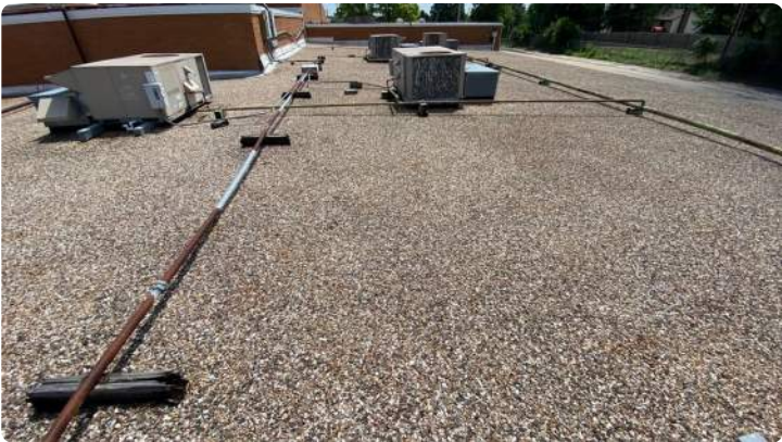
Photo showing additional overview of Area 17 roof.
