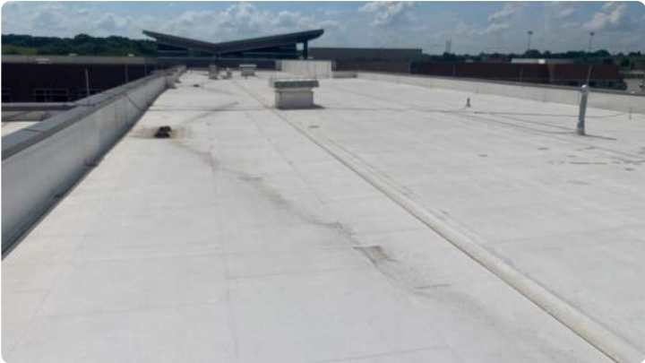
Photo showing overview of Area 13 roof.
