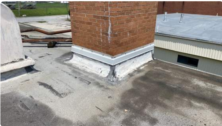
Photo showing condition of projection flashings.
