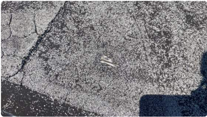
Photo showing gouge in field with exposed skim.
