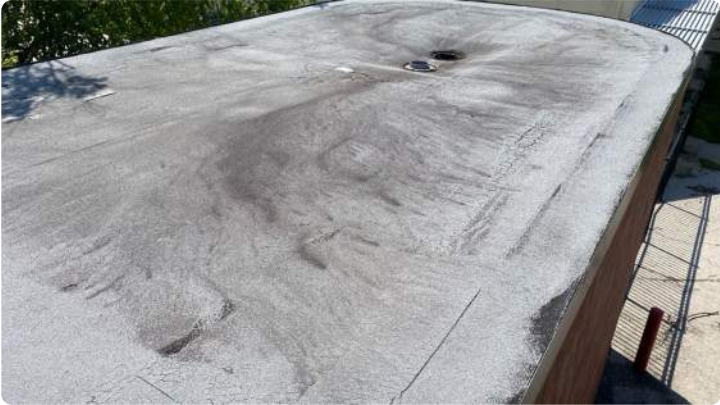
Photo showing overview of small roof section.
