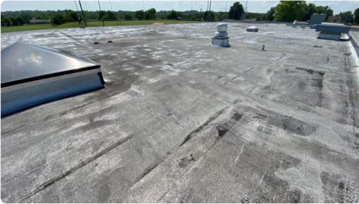
Photo showing overview of Area 08 roof.
