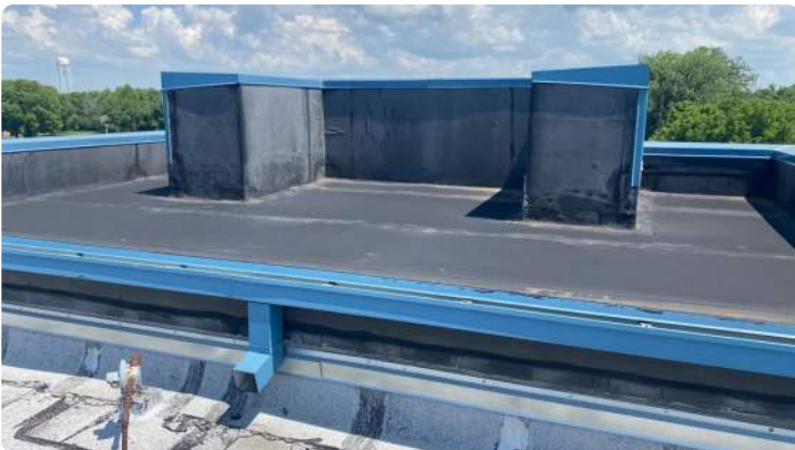
Photo showing condition of adjacent EPDM roof.
