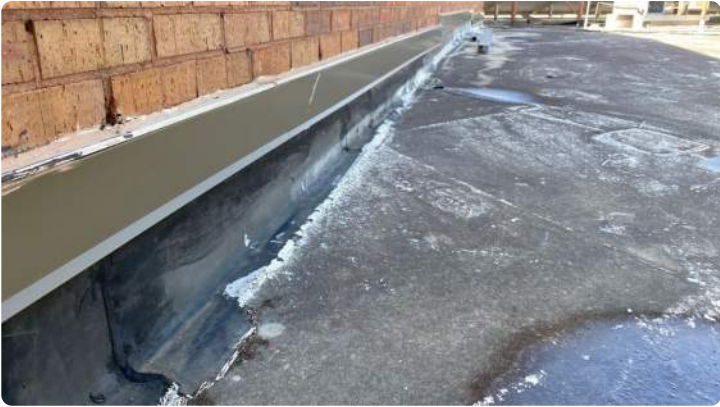
Photo showing condition of the perimeter flashings.
