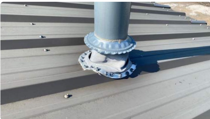
Photo showing condition of the projection flashing.
