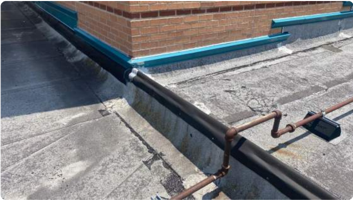
Photo showing condition of the expansion joint.
