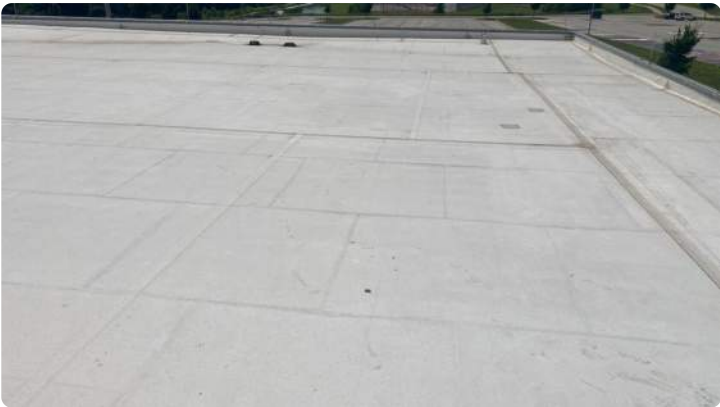
Photo showing overview of Area 17 roof.
