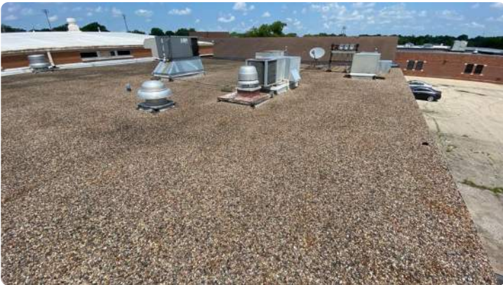
Photo showing additional overview of Area 20 roof.
