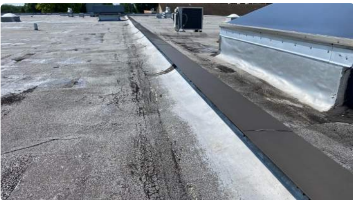
Photo showing condition of the perimeter flashings.
