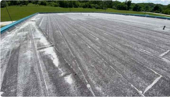
Photo showing overview of Area 07 roof.
