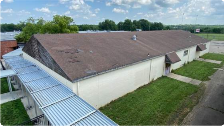
Photo showing overview of Area 23 roof.
