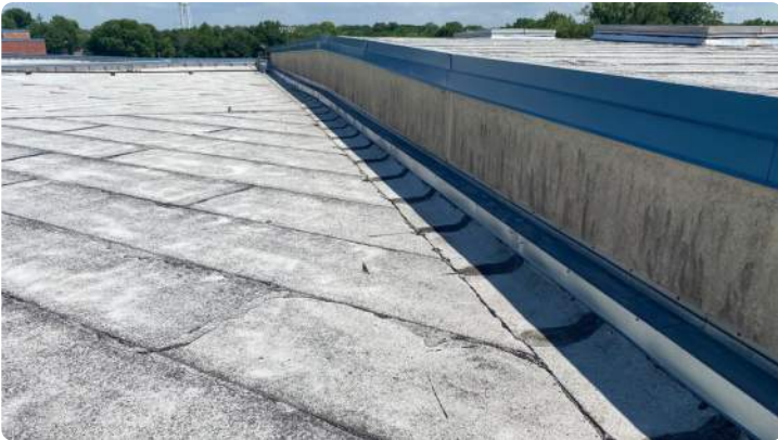
Photo showing condition of the perimeter flashings.
