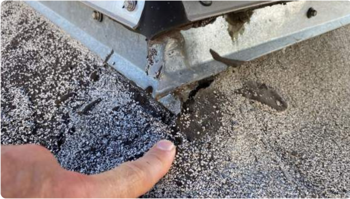
Photo showing a hole in the projection flashings. Repaired as part of the maintenance agreement.
