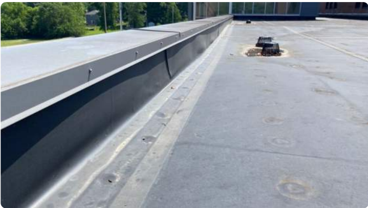
Photo showing condition of the perimeter flashings.
