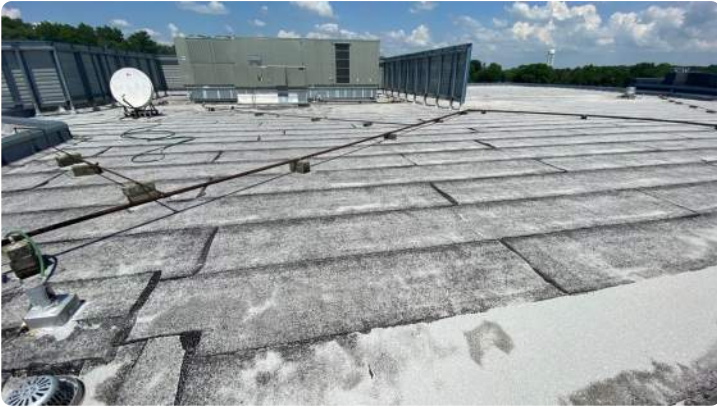
Photo showing overview of Area 06 roof.
