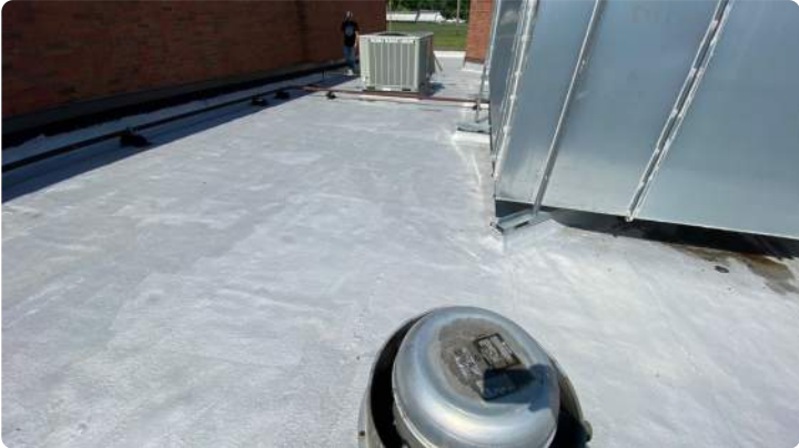
Photo showing additional overview of Area 01 roof.
