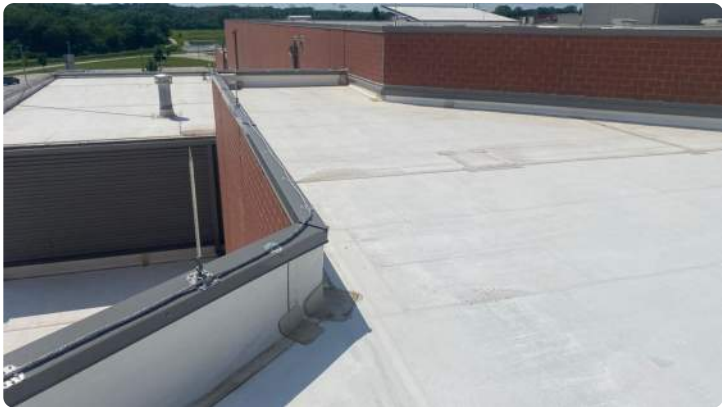
Photo showing overview of Area 08 roof.
