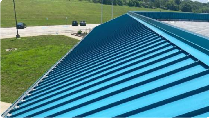
Photo showing overview of adjacent metal roof.
