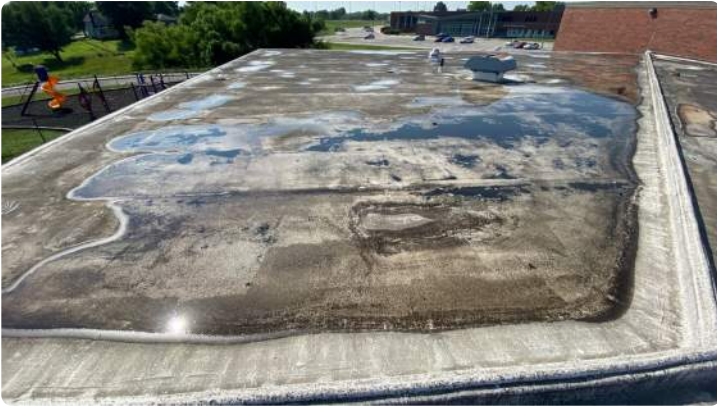
Photo showing overview of Area 02 roof.
