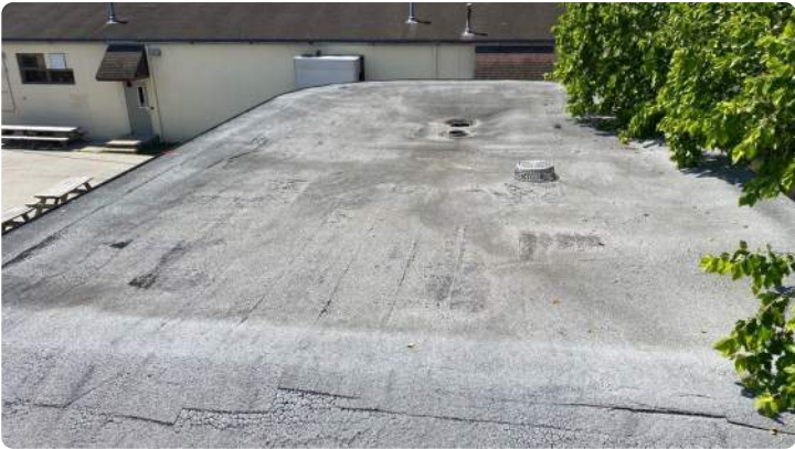
Photo showing overview of small roof section.
