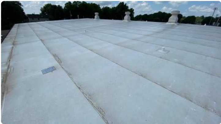
Photo showing overview of Area 21 roof.
