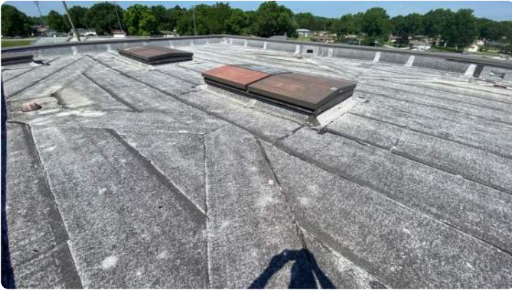
Photo showing overview of Area 04 roof.
