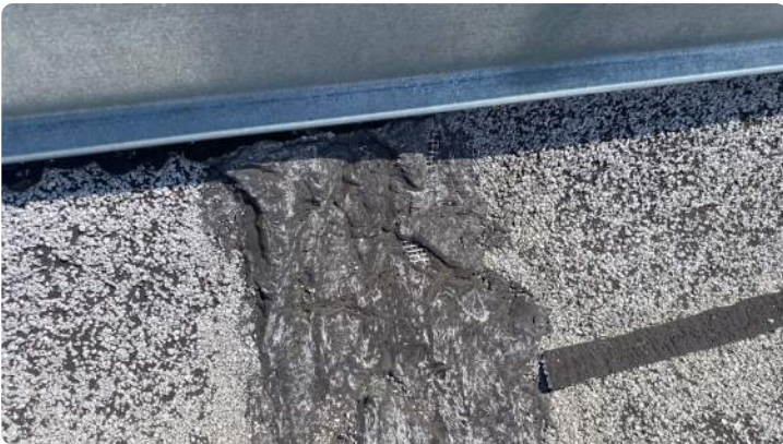
Photo showing skim visible through projection flashings.
