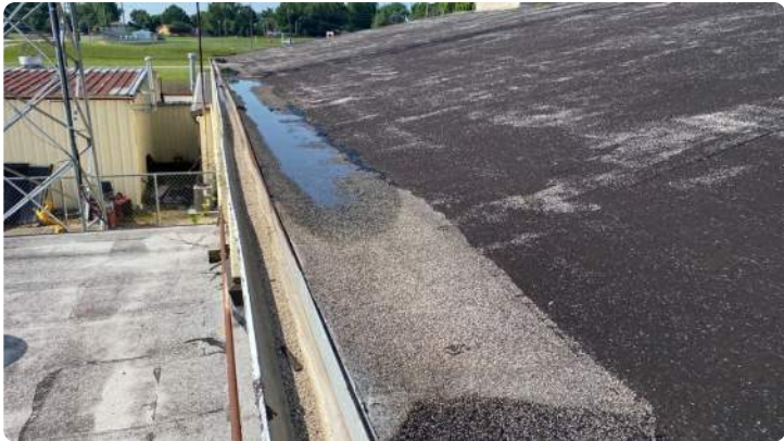
Photo showing condition of the perimeter gutter.
