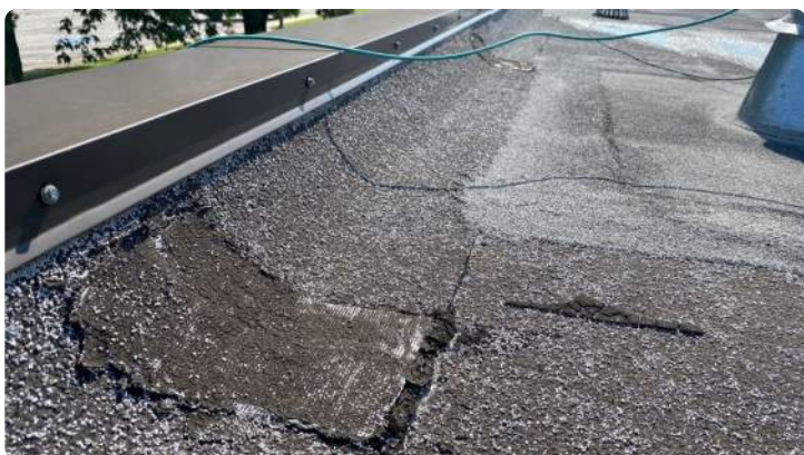
Photo showing condition of the perimeter flashings.
