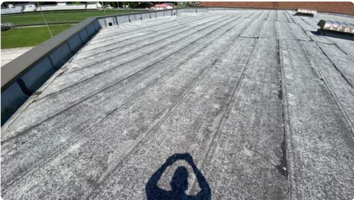
Photo showing overview of Area 03 roof.
