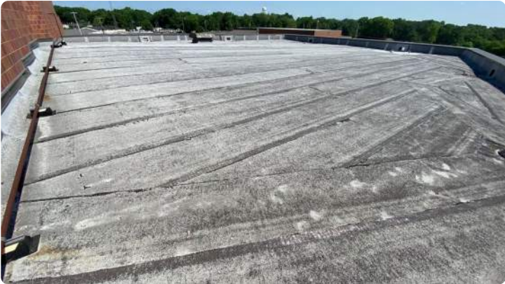
Photo showing overview of Area 02 roof.
