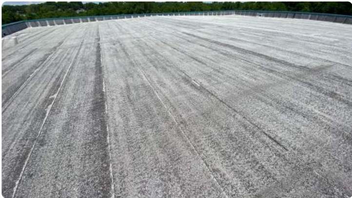
Photo showing overview of Area 04 roof.
