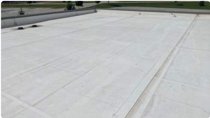
Photo showing overview of Area 16 roof.
