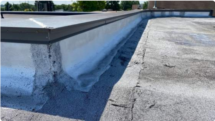
Photo showing condition of the perimeter flashings.
