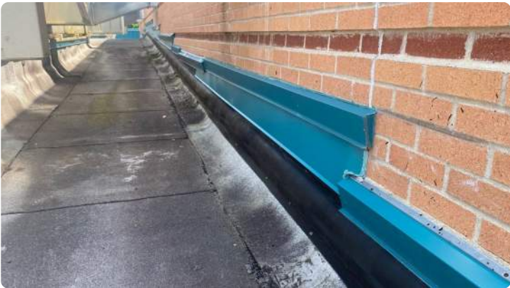
Photo showing condition of the perimeter flashings.
