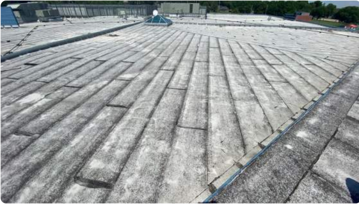
Photo showing overview of Area 05 roof.
