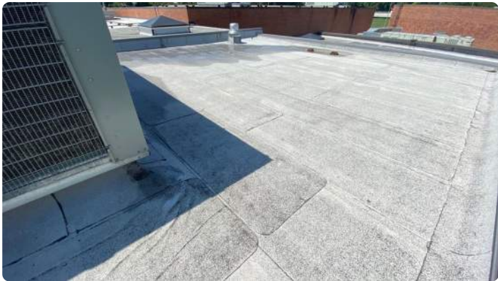
Photo showing overview of Area 12 roof.
