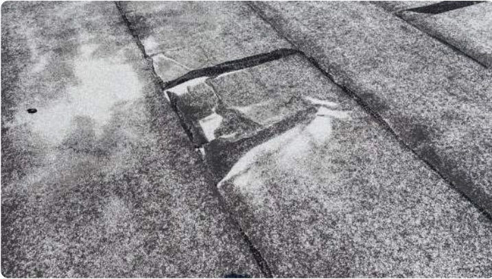
Photo showing area where field is wrinkled with fish-mouths.
