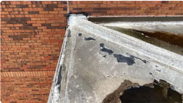
Photo showing condition of the perimeter flashings.
