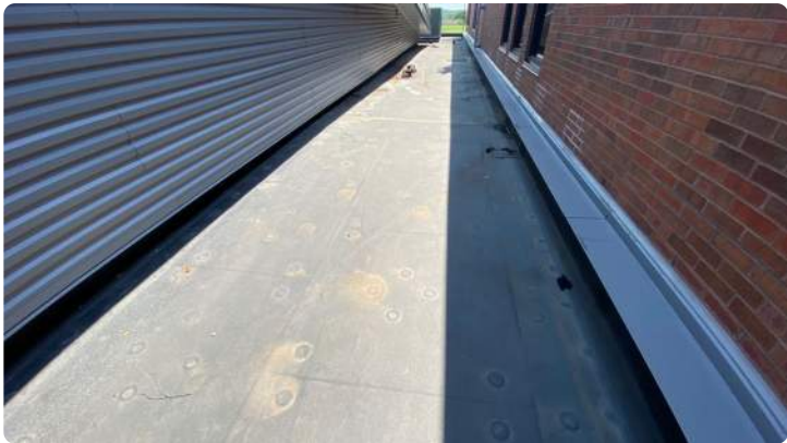
Photo showing additional overview of Area 10 roof.
