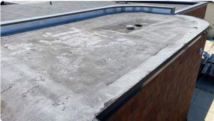
Photo showing overview of additional small roof section.
