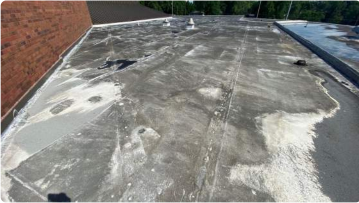
Photo showing overview of Area 01 roof.
