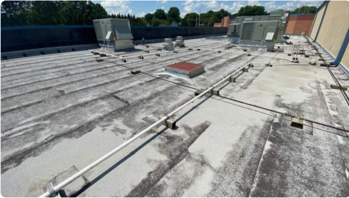
Photo showing overview of Area 04 roof.
