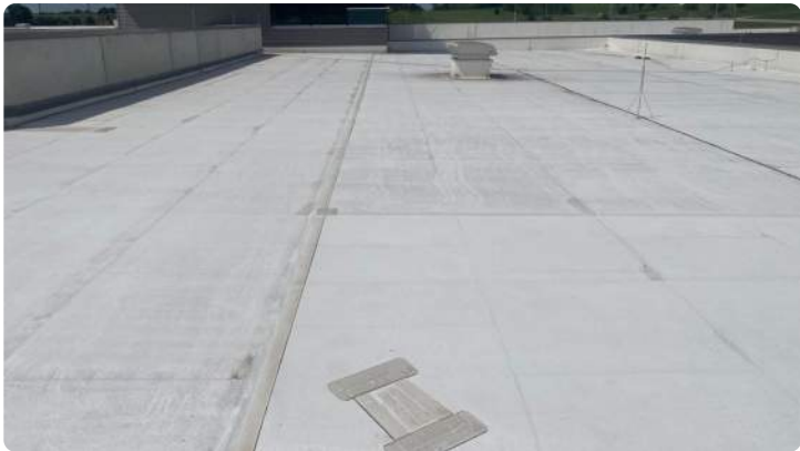
Photo showing additional overview of Area 08 roof.
