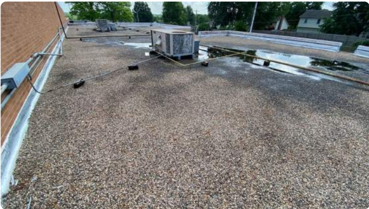
Photo showing overview of Area 18 roof.
