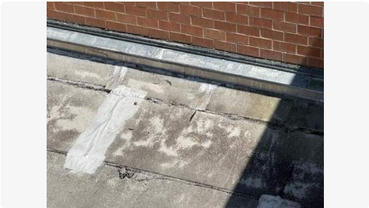
Photo showing condition of the perimeter flashings.
