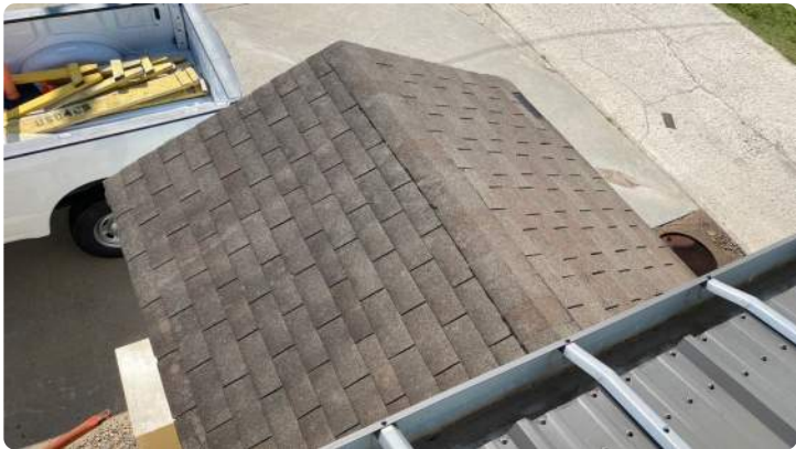
Photo showing adjacent shingle roof.
