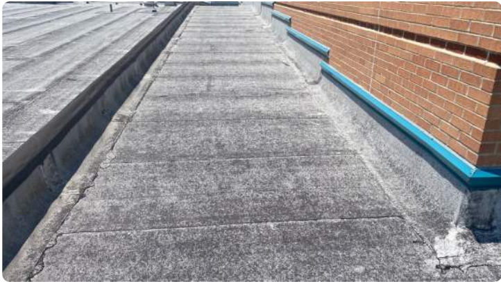
Photo showing condition of the perimeter flashings.
