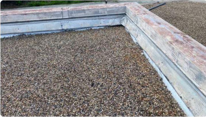
Photo showing condition of the perimeter flashings.
