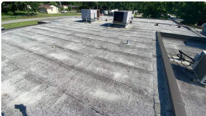
Photo showing overview of Area 03 roof.
