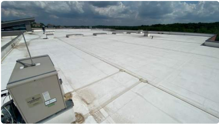
Photo showing overview of Area 05 roof.
