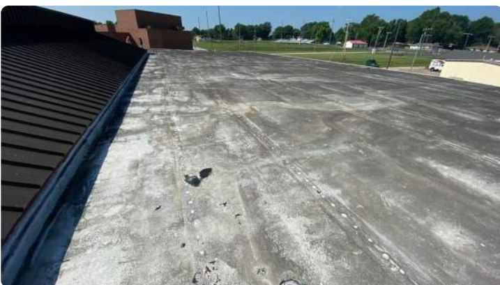
Photo showing additional overview of Area 01 roof.
