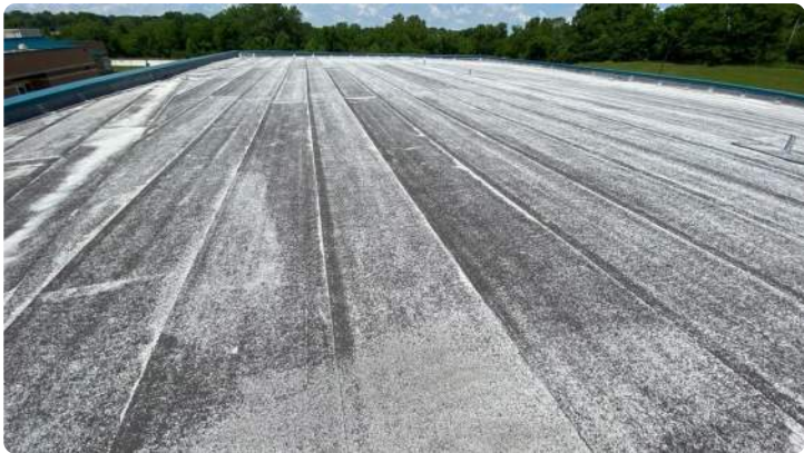
Photo showing overview of Area 11 roof.
