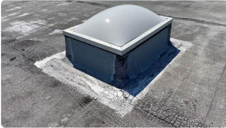
Photo showing aluminum coated skylight flashings.
