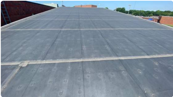
Photo showing overview of Area 11 roof.
