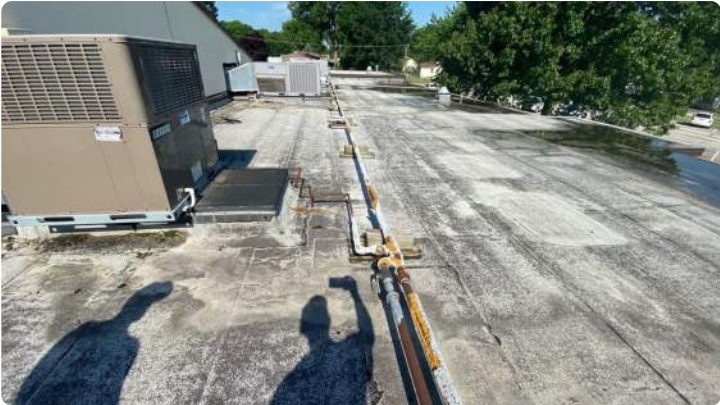
Photo showing overview of Area 02 roof.
