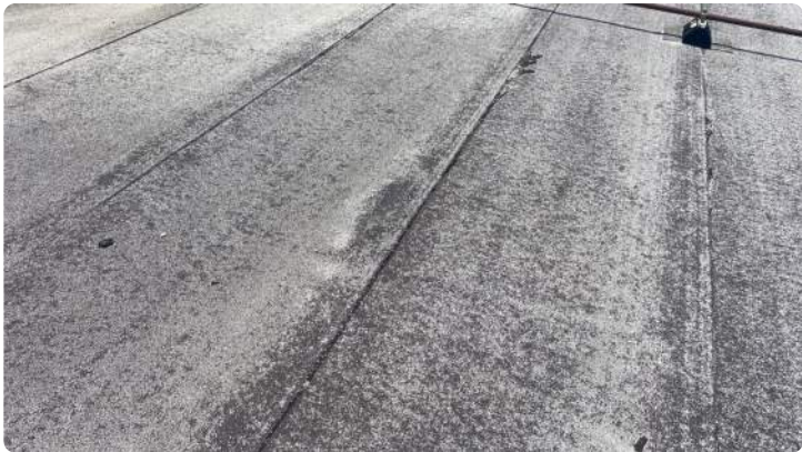
Photo showing skim exposed in the field.
