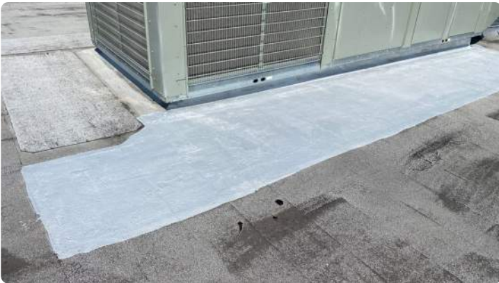
Photo showing aluminum coating around projection.
