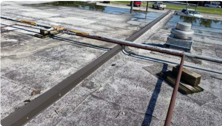
Photo showing condition of the expansion joint.
