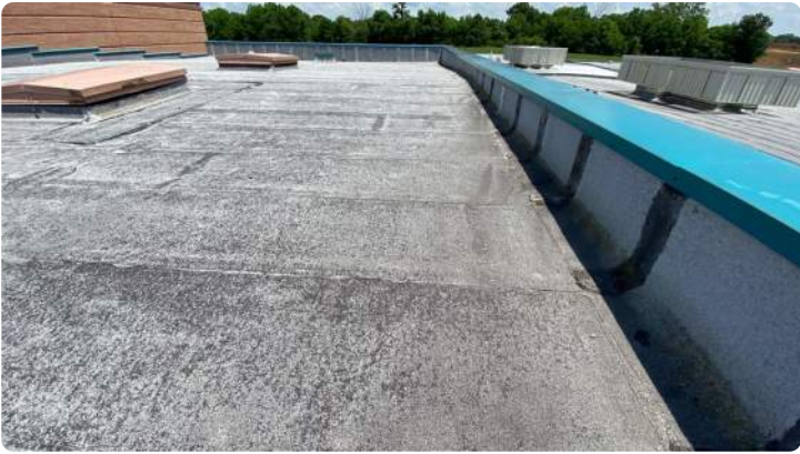
Photo showing condition of the perimeter flashings.
