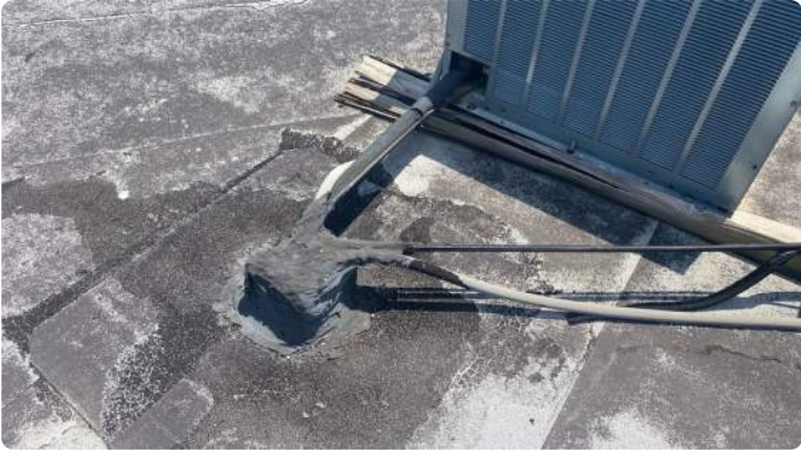
Photo showing condition of the pitch pan.
