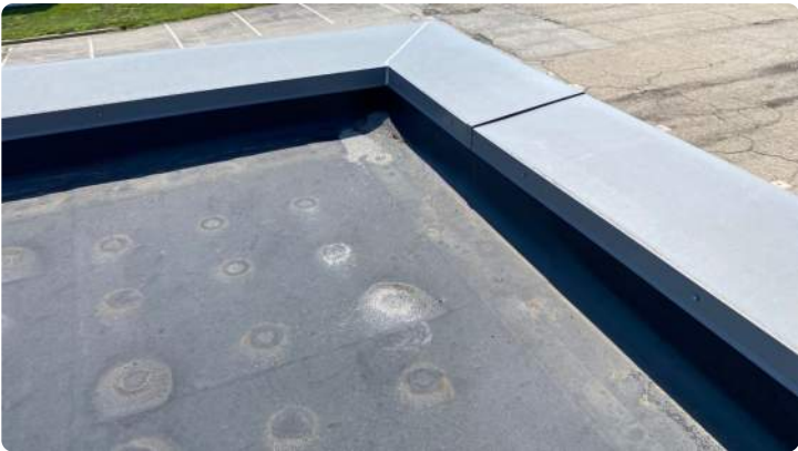
Photo showing condition of the perimeter flashings.
