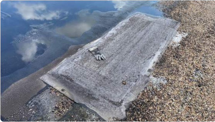
Photo showing area of gravel BUR repaired with base sheet.
