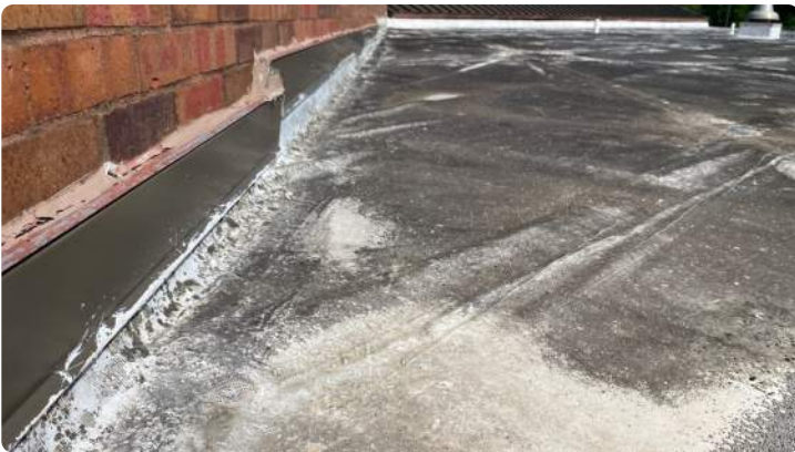
Photo showing condition of the perimeter flashings and loose membrane.
