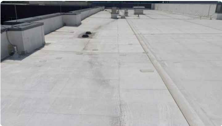
Photo showing additional overview of Area 13 roof.
