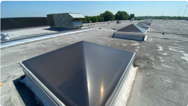
Photo showing additional overview of Area 07 roof.
