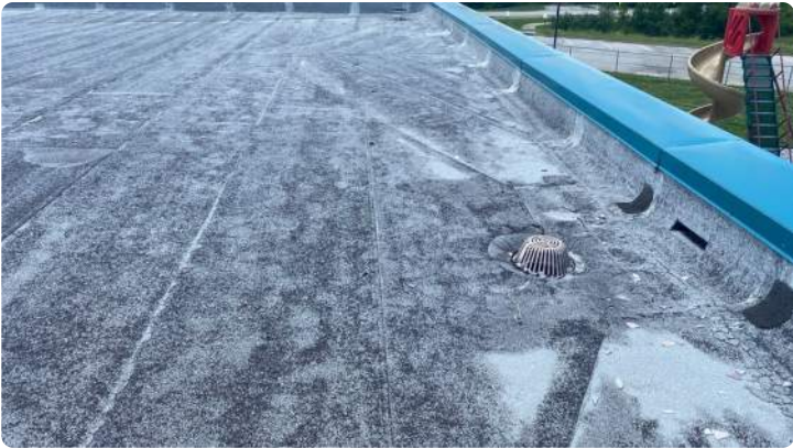
Photo showing condition of the perimeter flashings.
