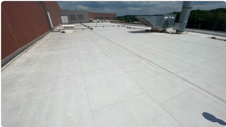
Photo showing overview of Area 06 roof.
