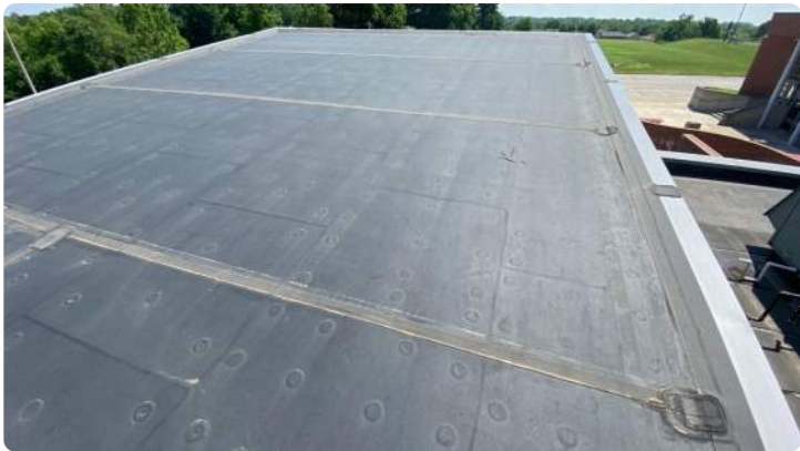
Photo showing additional overview of Area 11 roof.
