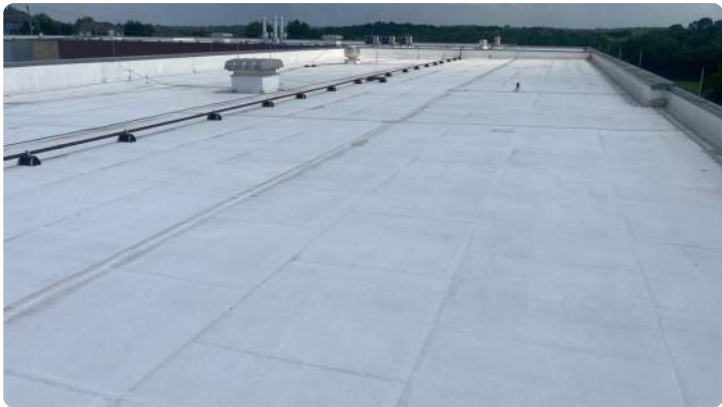
Photo showing overview of Area 10 roof.
