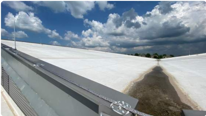
Photo showing additional overview of Area 15 roof.
