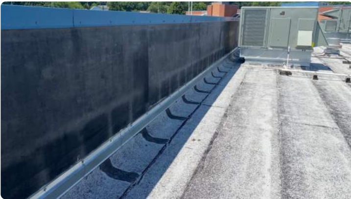
Photo showing condition of the perimeter flashings.
