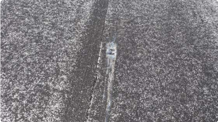
Photo showing skim showing through
