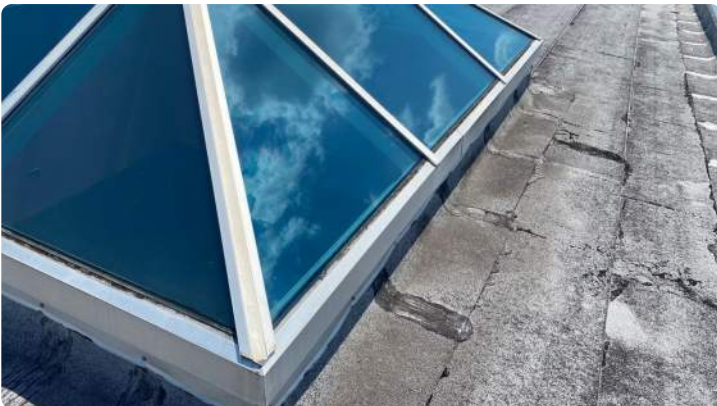
Photo showing condition of the skylight.
