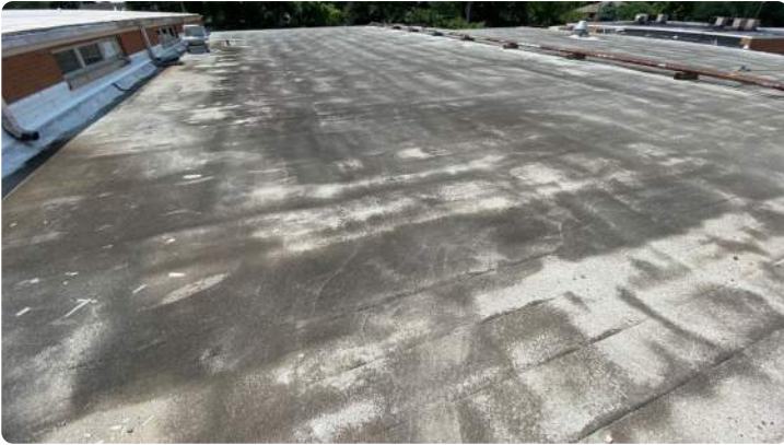
Photo showing overview of Area 22 roof.
