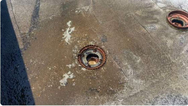
photo showing cleared drain.
