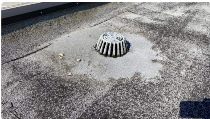
Photo showing granules piled up around drain.
