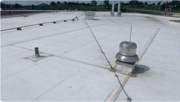
Photo showing overview of Area 12 roof.
