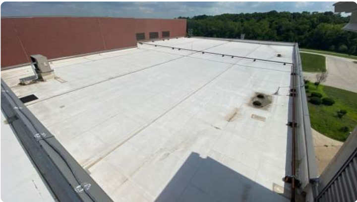
Photo showing overview of the Area 04 roof.
