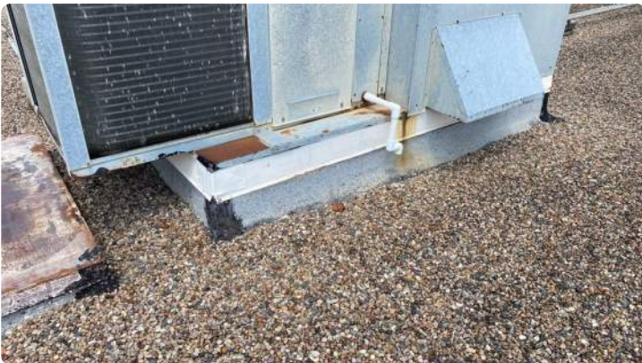
Photo showing condition of projection flashings.
