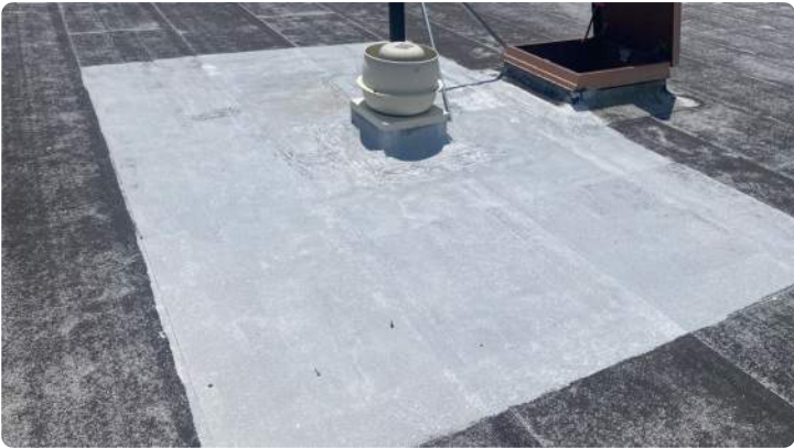
Photo showing area coated with aluminum.
