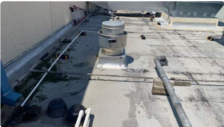
Photo showing additional overview of Area 01 roof.
