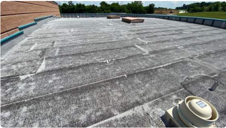
Photo showing overview of Area 03 roof.
