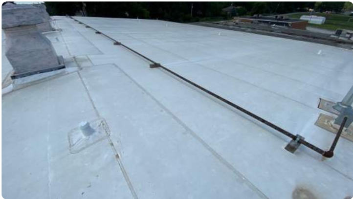
Photo showing overview of Area 21 roof.
