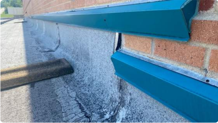
Photo showing condition of the perimeter flashings.
