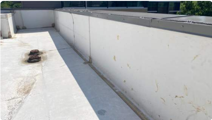
Photo showing condition of the perimeter flashings.
