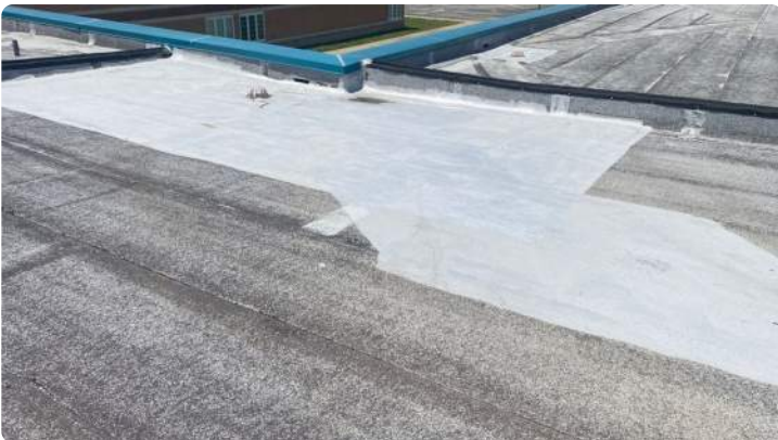
Photo showing section of roof previously coated.
