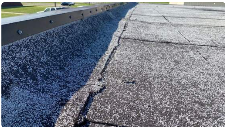
Photo showing condition of the perimeter flashings.
