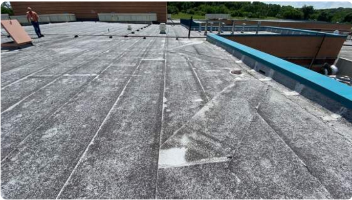
Photo showing overview of Area 01 roof.
