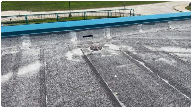
Photo showing condition of the perimeter flashings.
