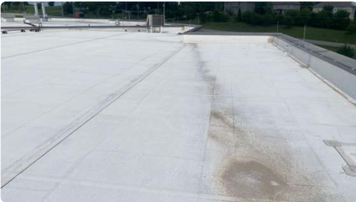
Photo showing additional overview of Area 11 roof.
