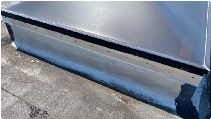
Photo showing condition of the skylight flashings.
