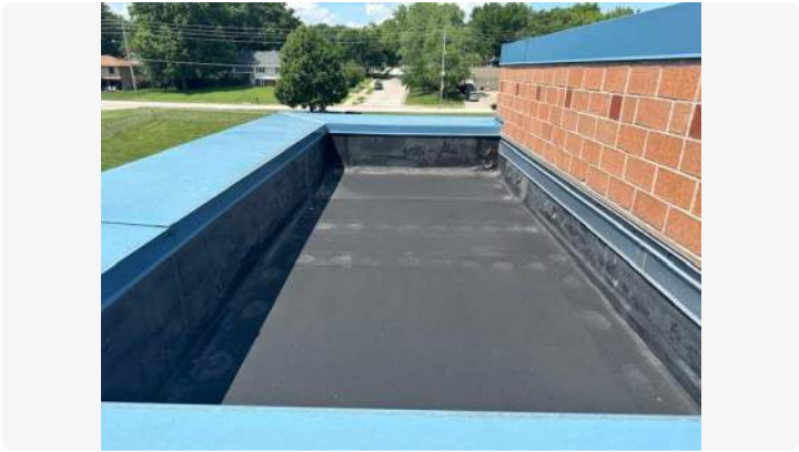
Photo showing adjacent EPDM section.
