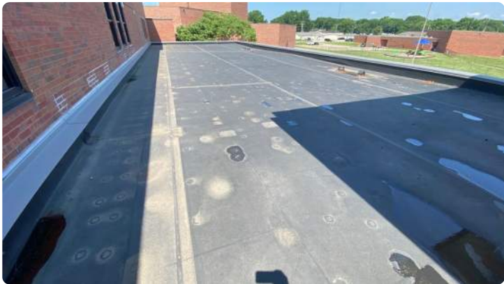
Photo showing overview of Area 10 roof.
