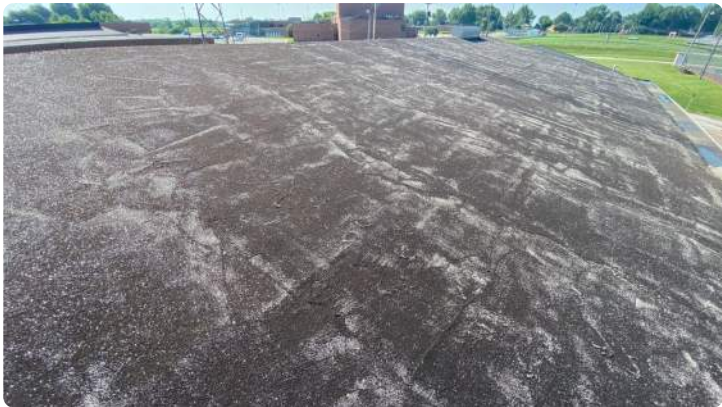
Photo showing overview of Area 04 roof.
