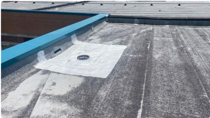
Photo showing additional area around drain coated with aluminum.
