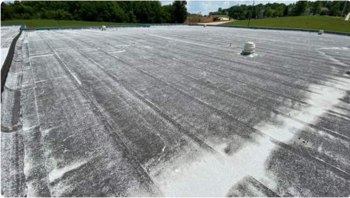
Photo showing overview of Area 09 roof.
