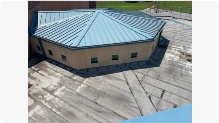
Photo showing additional overview of Area 07 roof.
