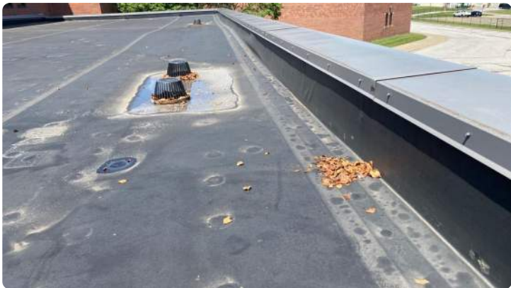
Photo showing condition of the perimeter flashings.
