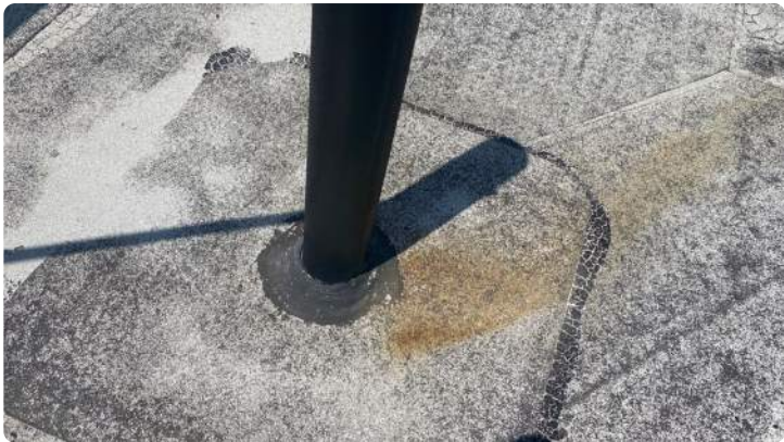
Photo showing vent flashings.
