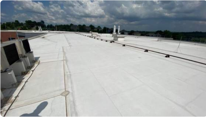
Photo showing overview of Area 11 roof.
