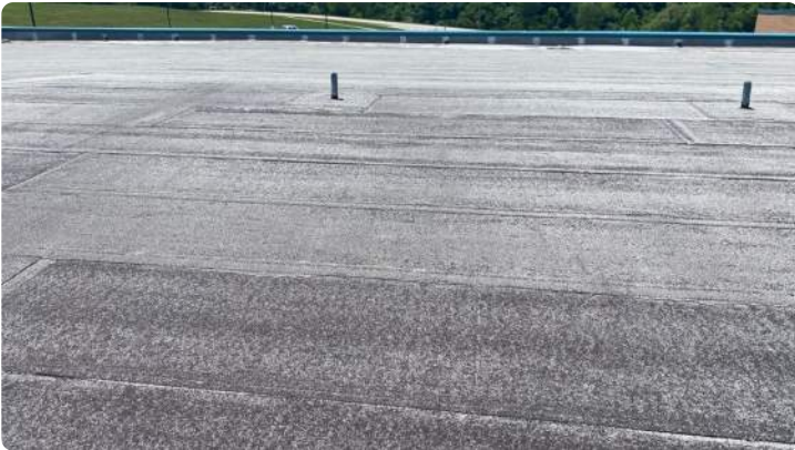
Photo showing additional overview of Area 07 roof.
