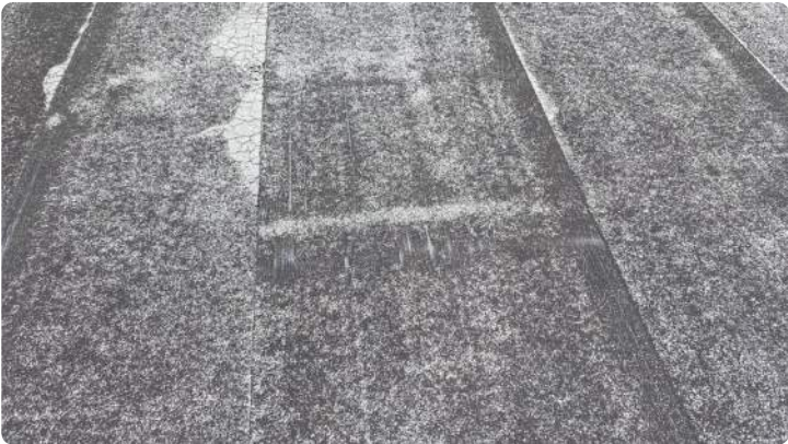
Photo showing skim exposed in field.
