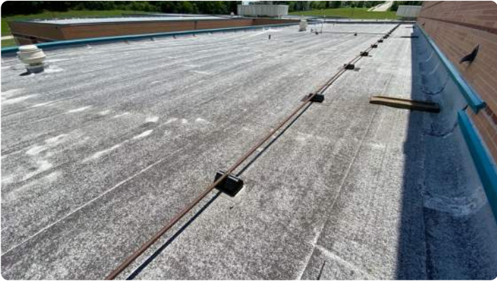
Photo showing overview of Area 02 roof.
