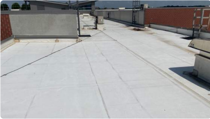
Photo showing overview of Area 02 roof.
