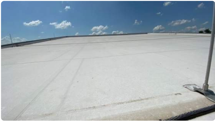
Photo showing overview of Area 03 roof.
