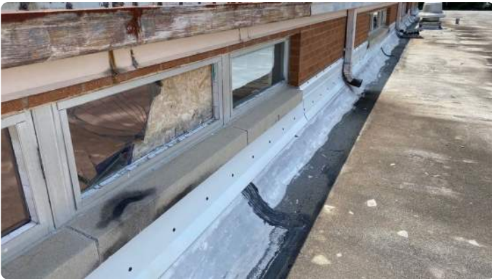
Photo showing condition of the perimeter flashings.
