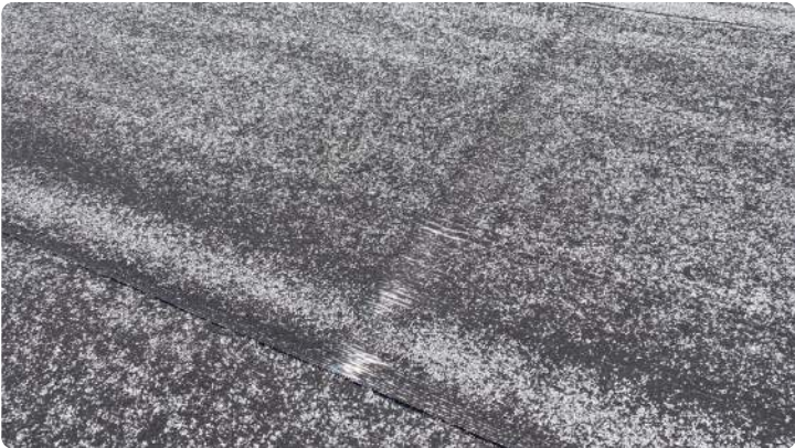
Photo showing skim exposed in field.
