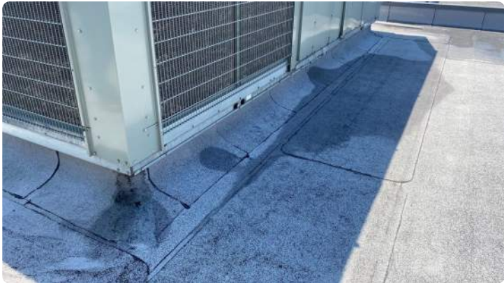
Photo ahowing condition of the perimeter flashings.
