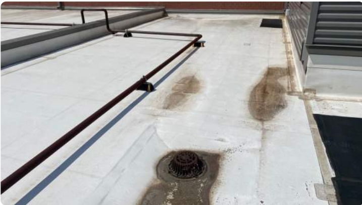
Photo showing additional overview of Area 07 roof.
