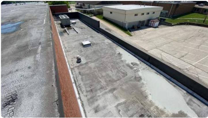
Photo showing overview of Area 14 roof.
