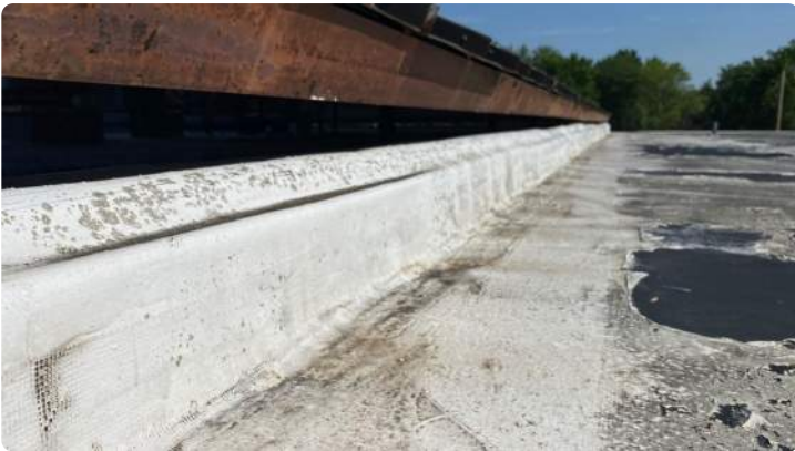
Photo showing condition of the perimeter flashings.
