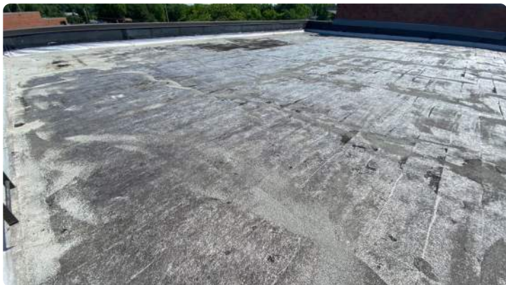
Photo showing overview of Area 06 roof.
