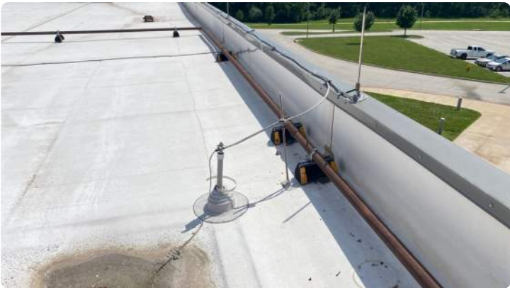
Photo showing condition of the perimeter flashings.
