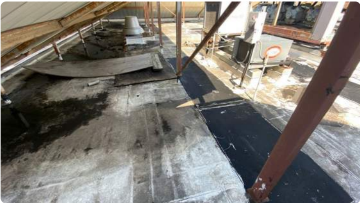
Photo showing overview of Area 03 roof.
