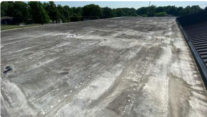
Photo showing additional overview of Area 01 roof.
