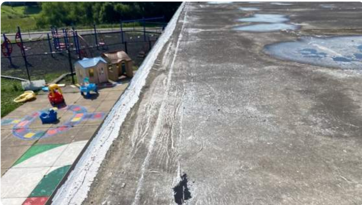
Photo showing condition of the perimeter flashings.
