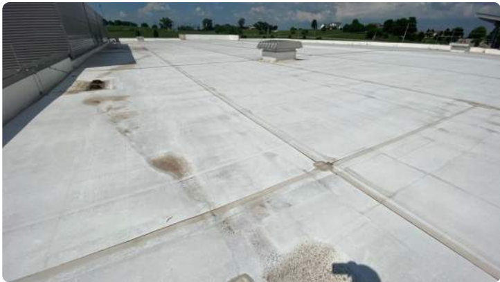
Photo showing overview of Area 14 roof.
