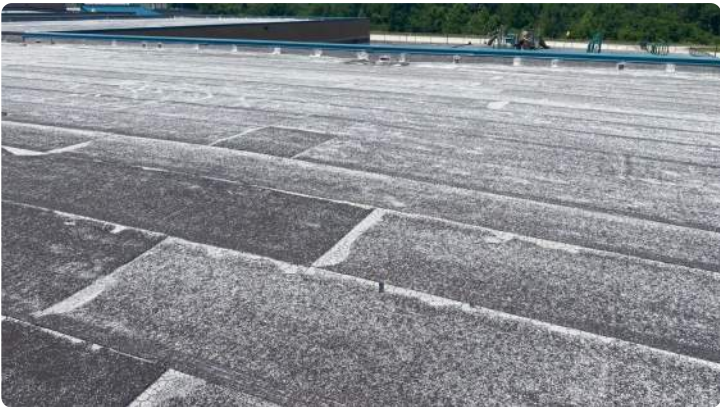
Photo showing exposed skim in deteriorated field.
