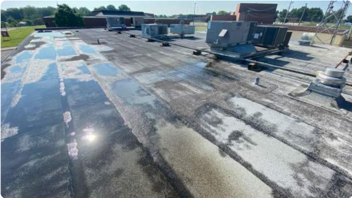
Photo showing overview of Area 01 roof.
