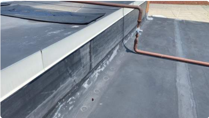
Photo showing condition of the perimeter flashings.
