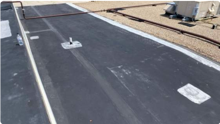
Photo showing overview of Area 16 roof.
