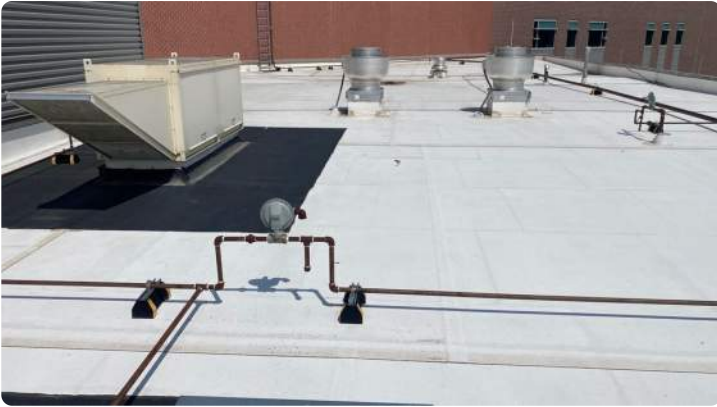
Photo showing overview of Area 07 roof.
