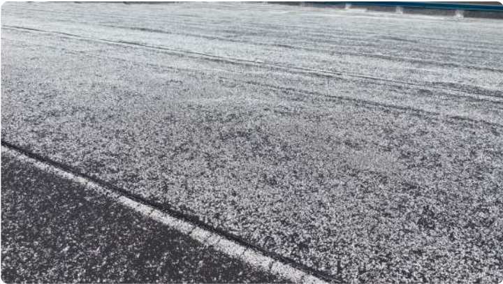
Additional photo of skim showing though field.
