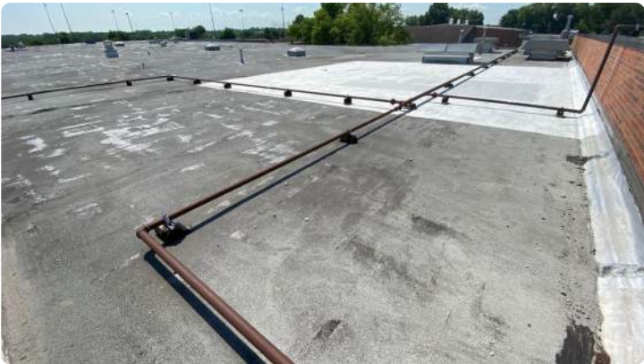
Photo showing overview of Area 07 roof.
