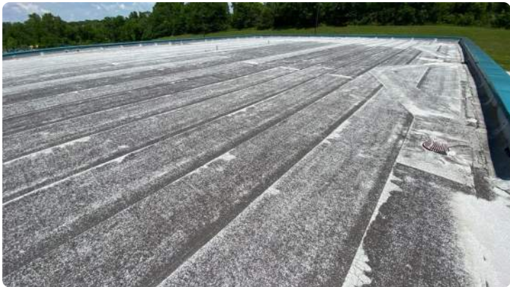
Photo showing overview of Area 10 roof.
