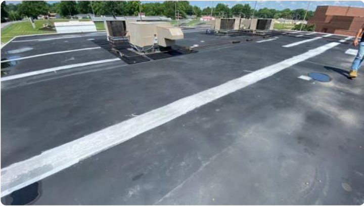
Photo showing overview of Area 15 roof.
