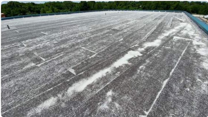
Photo showing overview of Area 05 roof.
