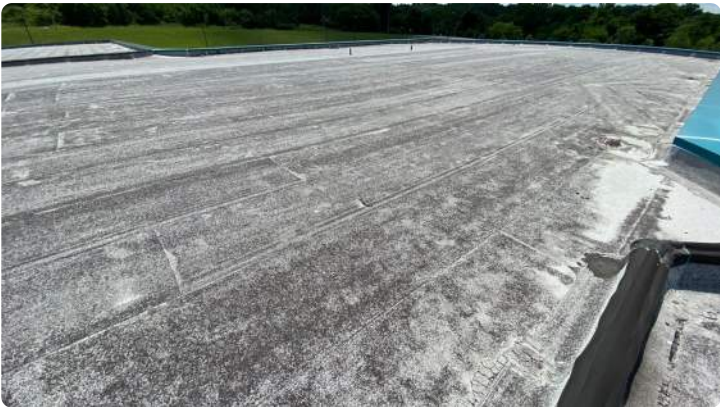
Photo showing overview of Area 06 roof.
