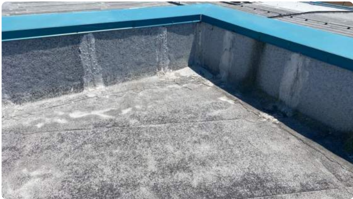
Photo showing condition of the perimeter flashings.
