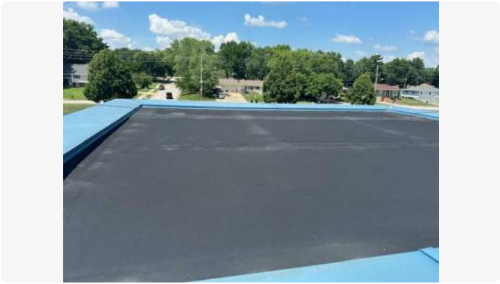
Photo showing additional EPDM section.
