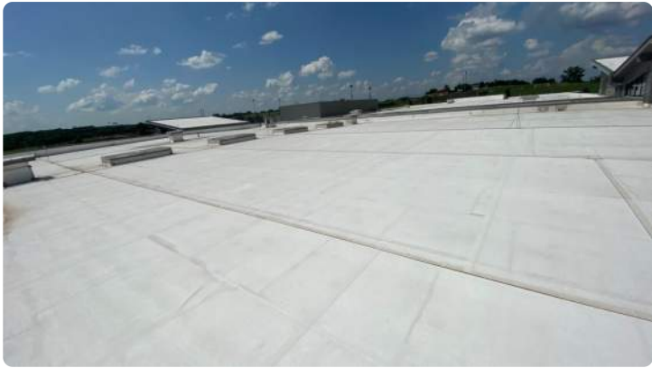
Photo showing additional overview of Area 05 roof.
