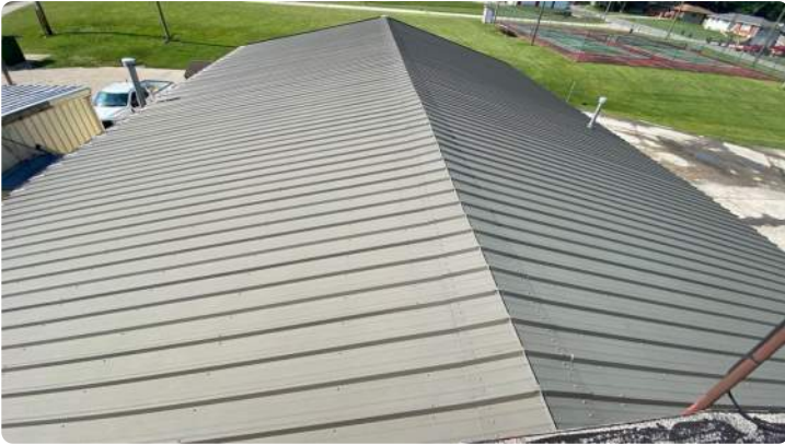
Photo showing overview of Area 05 roof.
