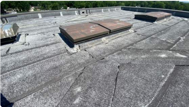
Photo showing additional overview of Area 04 roof.
