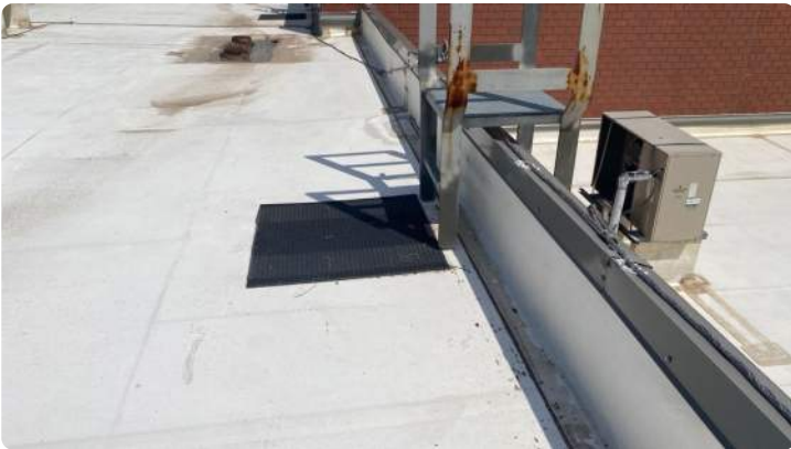
Photo showing condition of the perimeter flashings.
