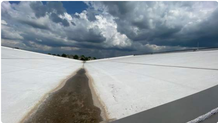
Photo showing overview of Area 15 roof.
