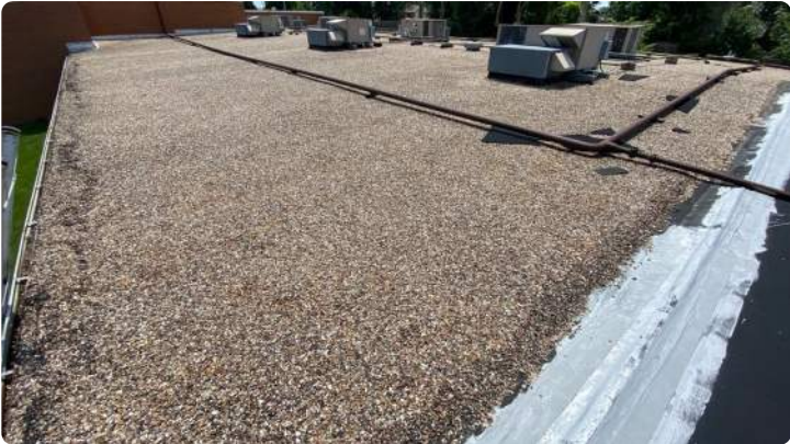
Photo showing overview of Area 17 roof.
