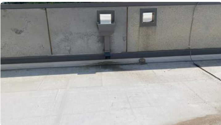
Photo showing additional photo of the perimeter flashings.
