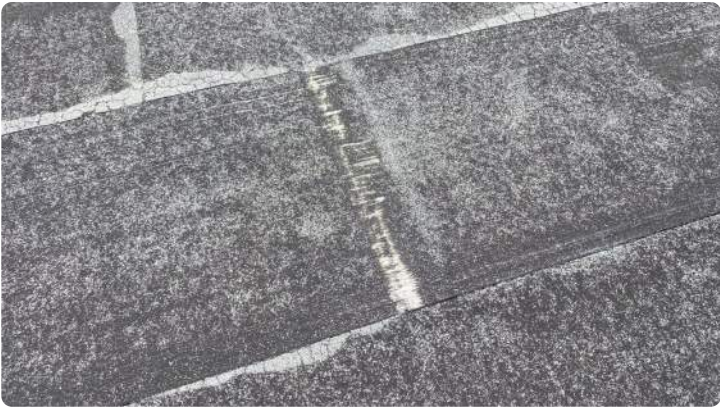
Photo showing skim exposed in field.
