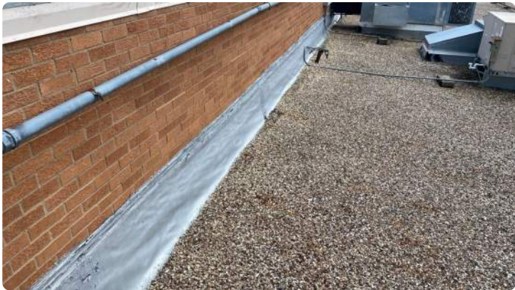
Photo showing condition of the perimeter flashings.
