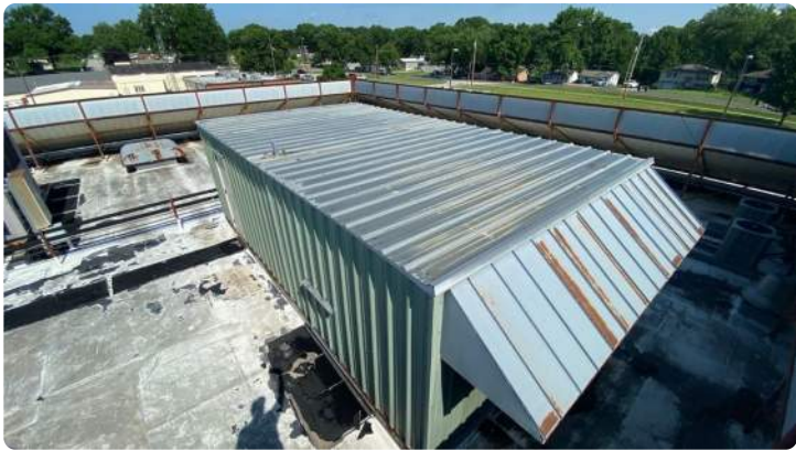
Photo showing condition of the central metal penthouse.
