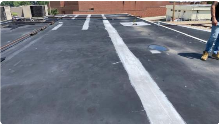
Photo showing a seam coated on EPDM membrane.
