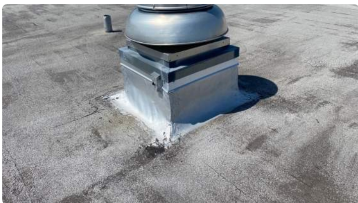
Photo showing aluminum coated projection flashings.
