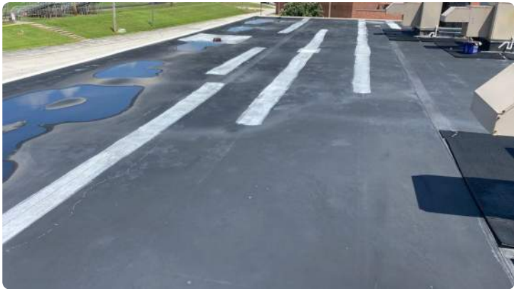
Photo showing additional coated seams.
