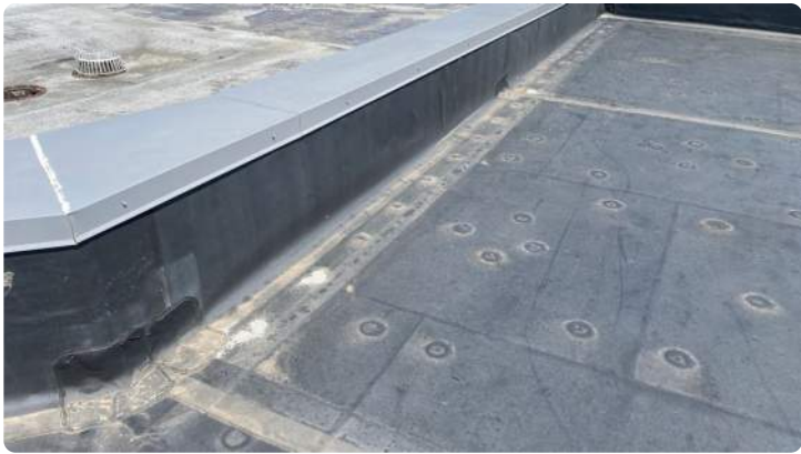
Photo showing condition of the perimeter flashings.
