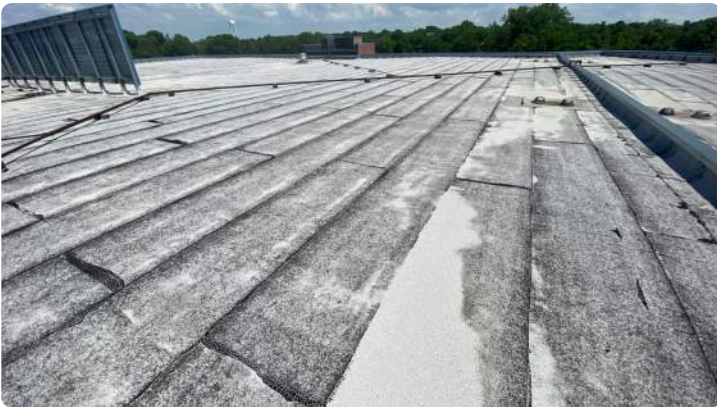
Photo showing additional overview of Area 06 roof.
