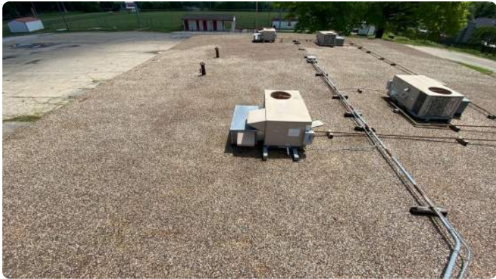
Photo showing additional overview of Area 19 roof.
