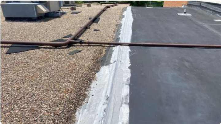
Photo showing connection from EPDM overlay with gravel BUR area.
