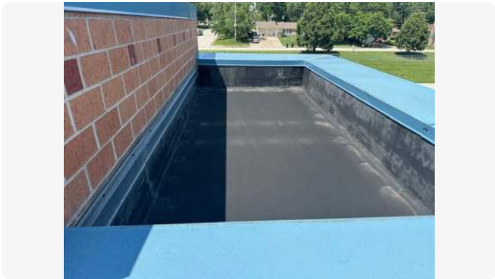
Photo showing additional EPDM section.
