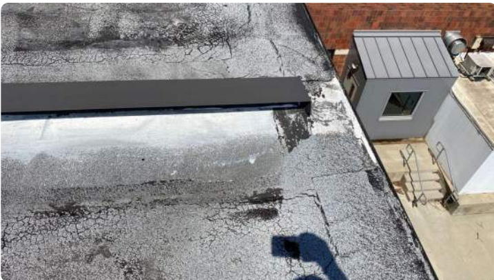
Photo showing condition of expansion joint.
