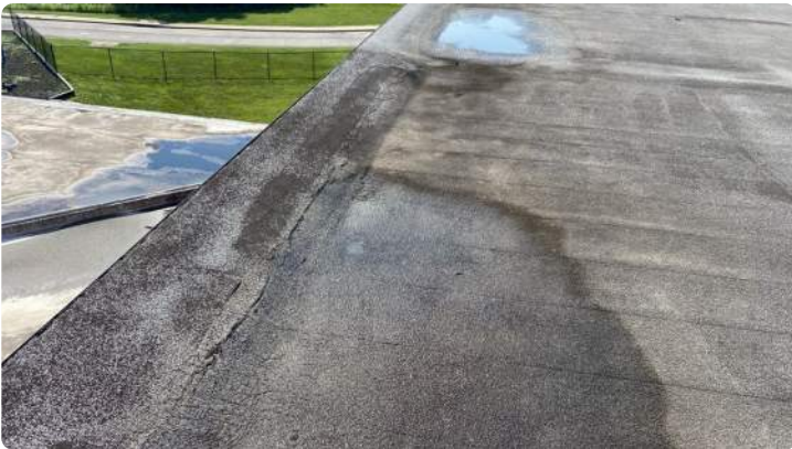
Photo showing condition of the perimeter flashings.
