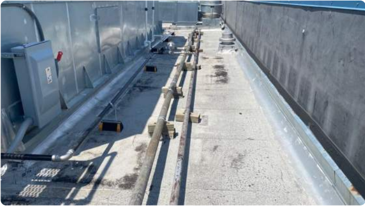
Photo showing overview of Area 01 roof.
