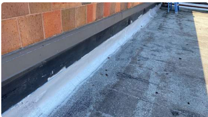
Photo showing condition of the perimeter flashings.
