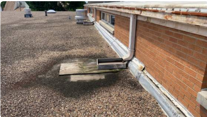
Photo showing condition of the perimeter flashings.
