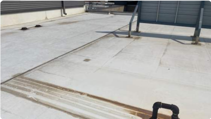
Photo showing additional overview of Area 17 roof.
