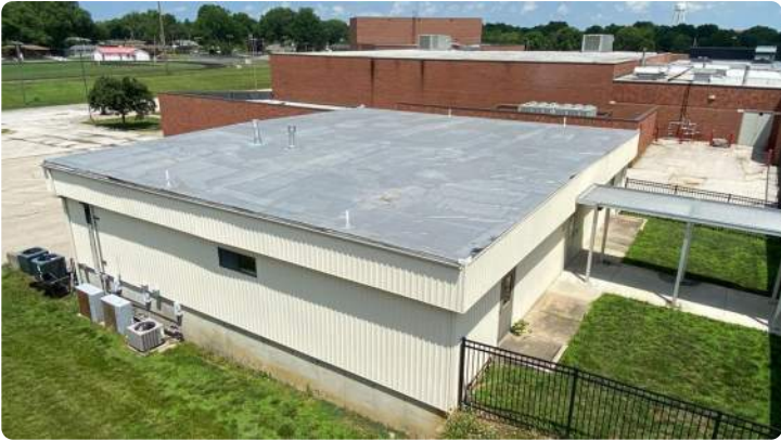
Photo showing overview of Area 24 roof.
