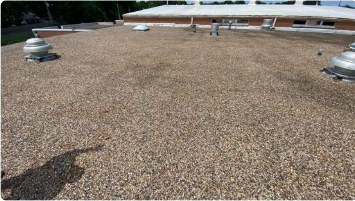
Photo showing overview of Area 20 roof.
