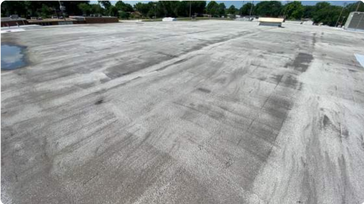
Photo showing overview of Area 13 roof.
