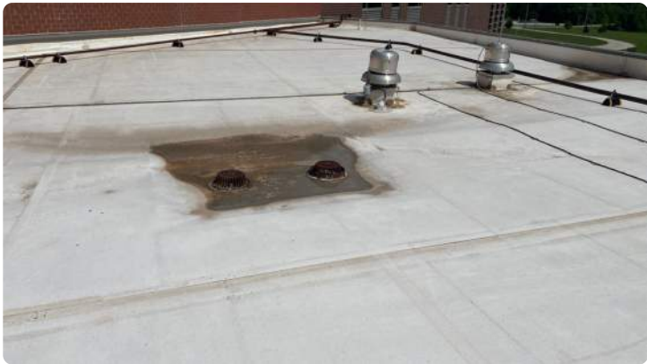
Photo showing additional overview of Area 07 roof.
