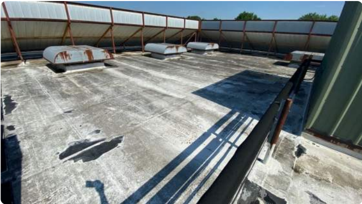
Photo showing additional overview of Area 03 roof.
