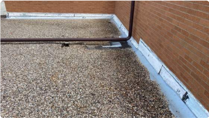
Photo showing condition of the perimeter flashings.
