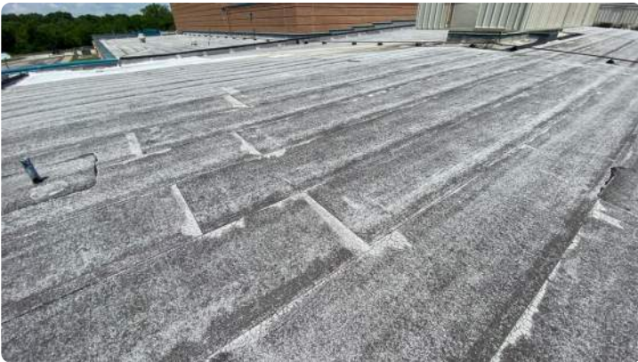
Additional overview of Area 08 roof.
