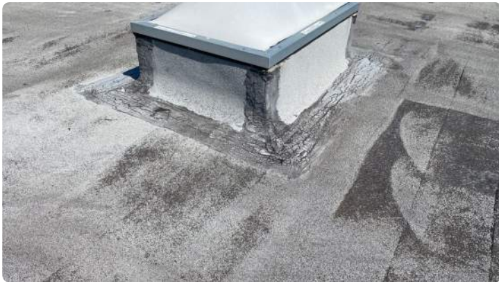
Photo showing condition of projection flashings.
