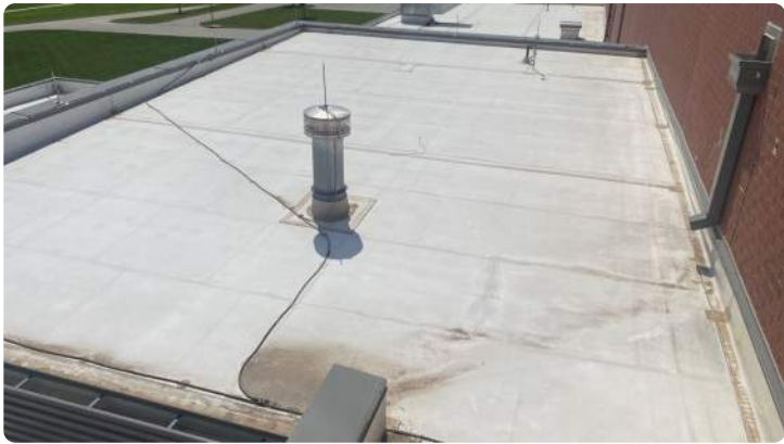
Photo showing overview of Area 09 roof.
