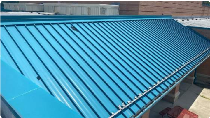
Photo showing condition of adjacent roof.
