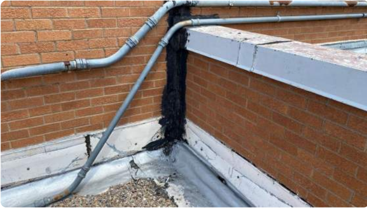
Photo showing a repair made to the corner with roofing mastic.
