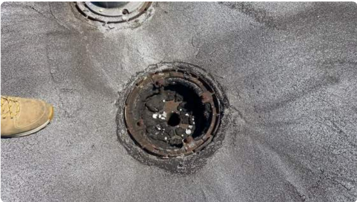
Photo showing condition of drain in small section.
