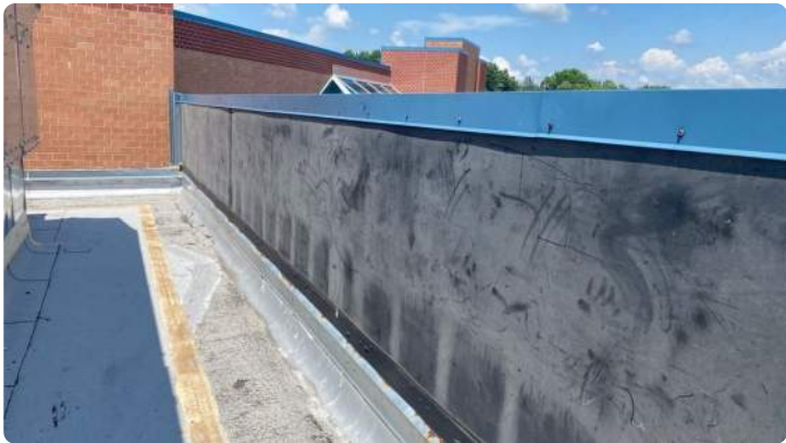
Photo showing condition of wall membrane.
