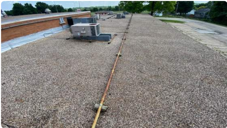
Photo showing overview of Area 19 roof.
