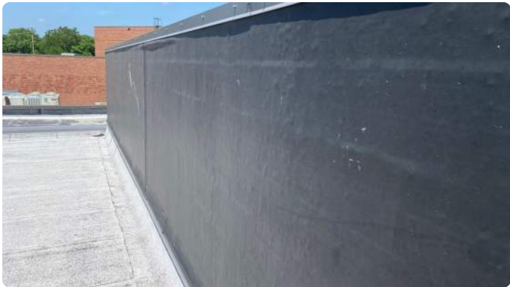
Photo showing condition of the perimeter flashings.
