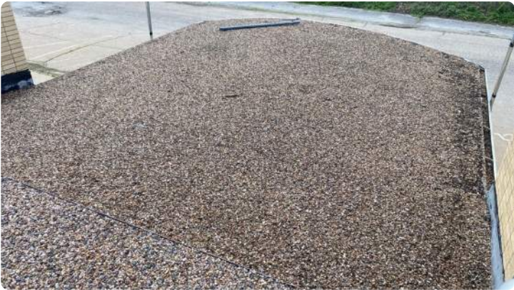
Photo showing overview of smaller section of roof.
