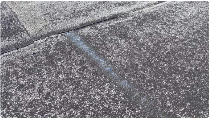
Photo showing skim showing through field.
