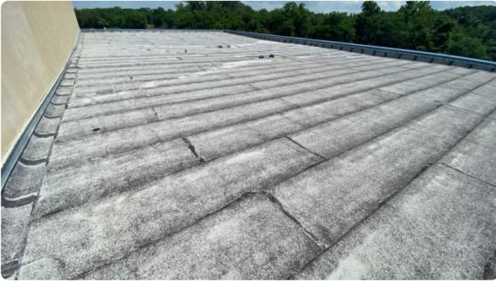
Photo showing overview of Area 03 roof.
