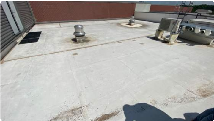
Photo showing overview of Area 01 roof.
