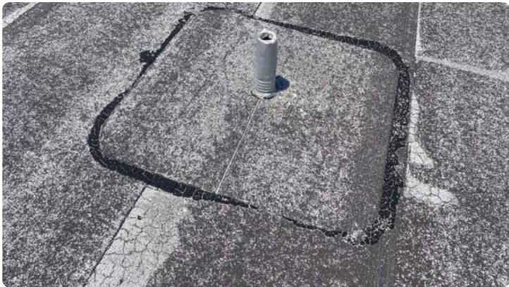
Photo showing skim exposed in target patch.
