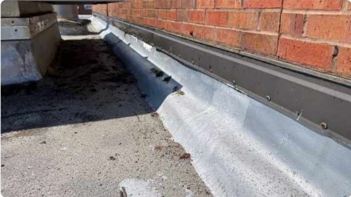
Photo showing condition of the perimeter flashings.
