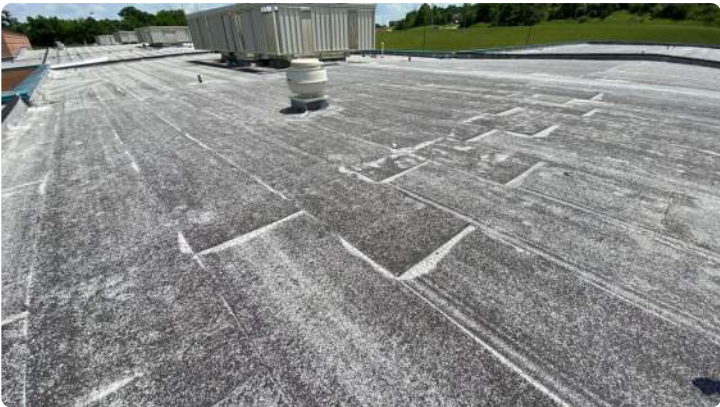
Additional overview of Area 06 roof.
