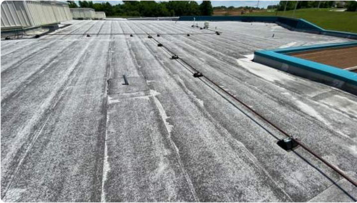
Photo showing overview of Area 08 roof.
