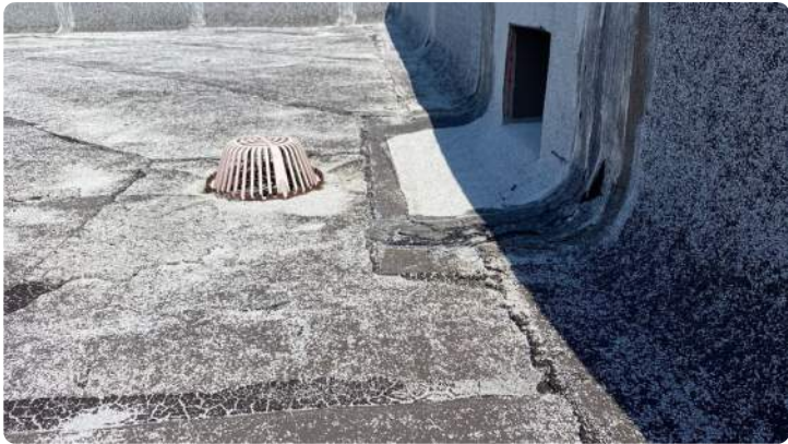
Photo showing condition of the perimeter flashings and drain.
