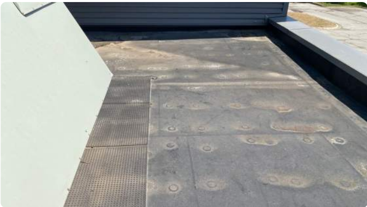
Photo showing additional overview of Area 10 roof.
