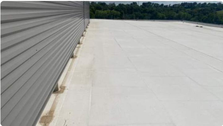
Photo showing additional overview of Area 17 roof.
