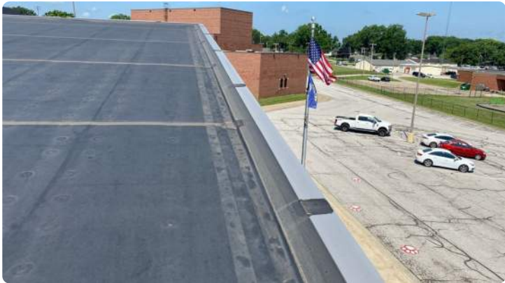
Photo showing condition of the perimeter flashings.
