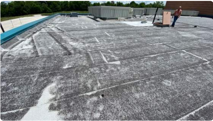
Photo showing additional overview of Area 01 roof.
