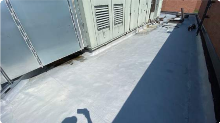
Photo showing overview of Area 01 roof.
