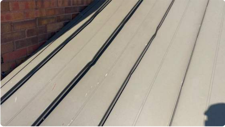
Photo showing additional condition of the metal awning.
