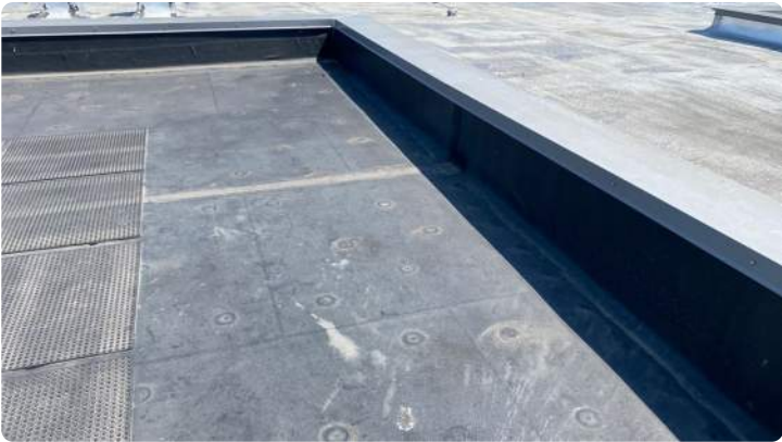
Photo showing condition of the perimeter flashings.
