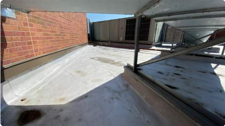
Photo showing additional overview of Area 01 roof.
