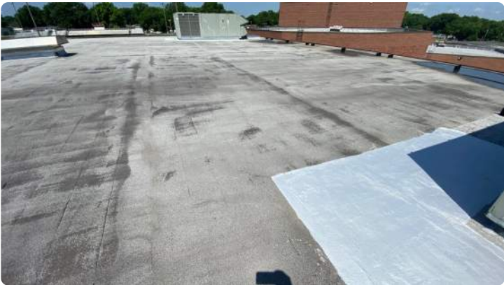
Photo showing additional overview of Area 13 roof.
