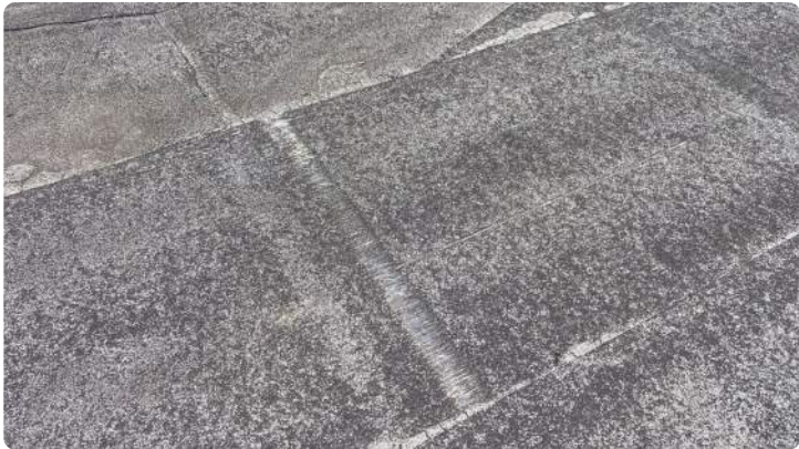
Photo showing skim showing through field.
