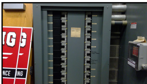
Branch Circuit Panelboards
