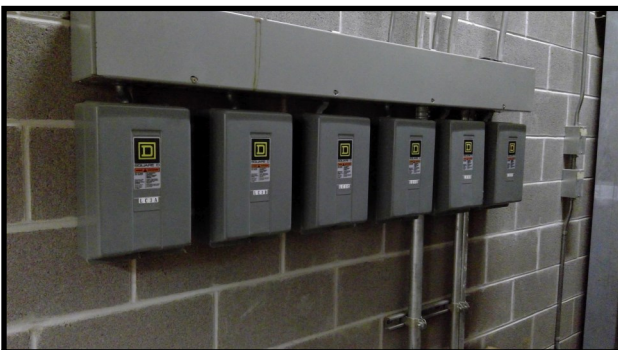
Exterior Lighting Controls
