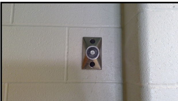
Electromagnetic Door Holds
