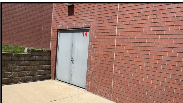
Brick Around Door-Effervescence
