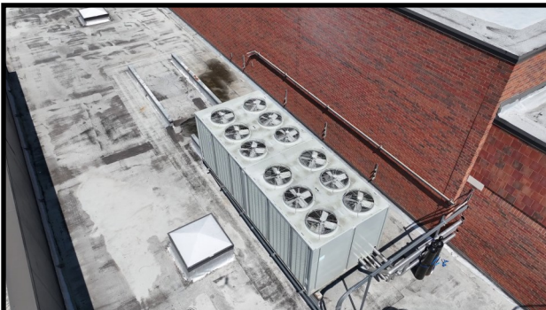
Air Cooled Condensing Units
