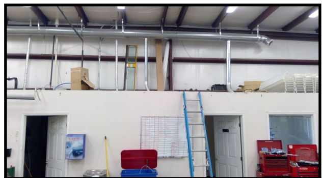
Air Distribution Ductwork
