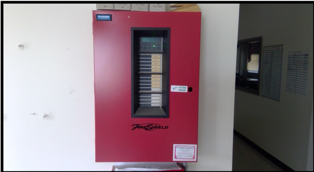
Fire Alarm Control Panel
