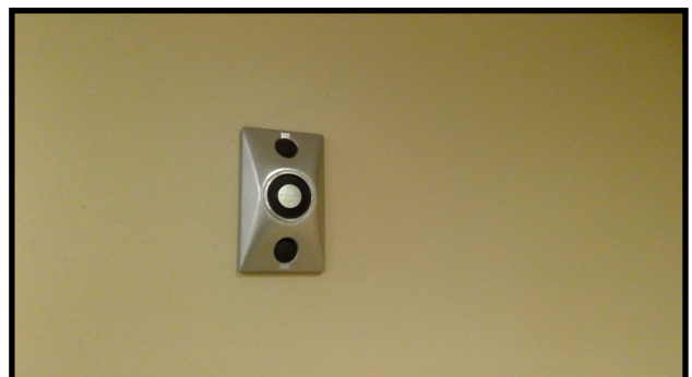
Electromagnetic Door Holds
