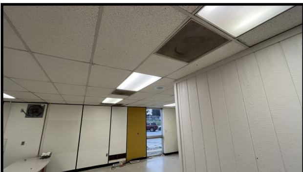
Room Finishes—Water Damage
