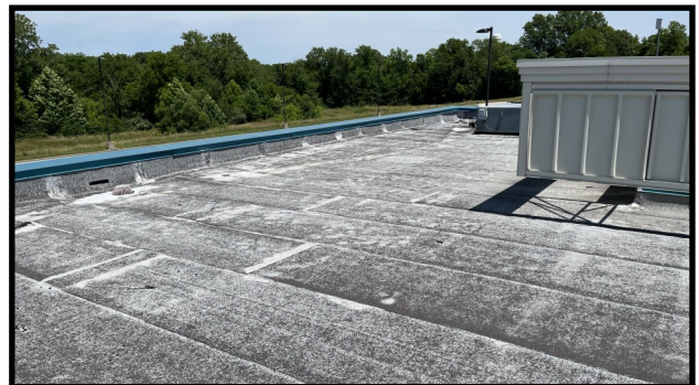
Modified Bitumen Roof
