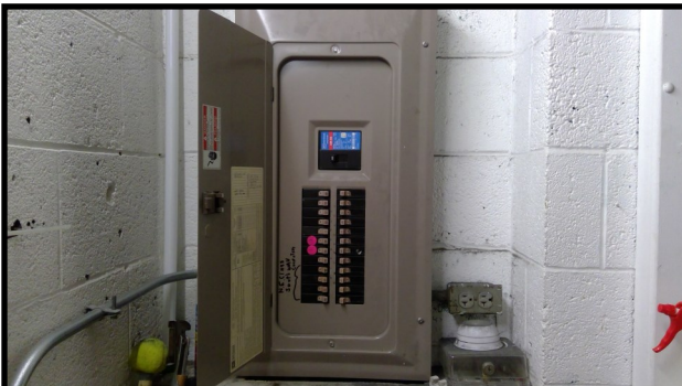
Branch Circuit Panelboards
