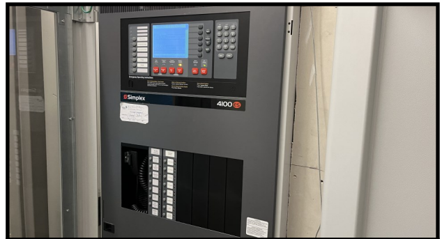
Fire Alarm Control Panel
