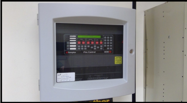
Fire Alarm Control Panel
