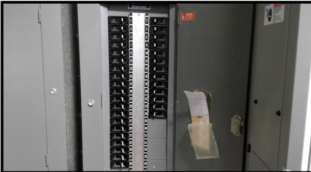
Branch Circuit Panelboards
