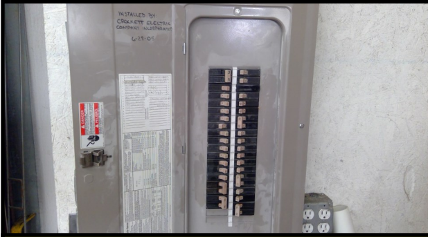
Interior Branch Circuit Panelboards
