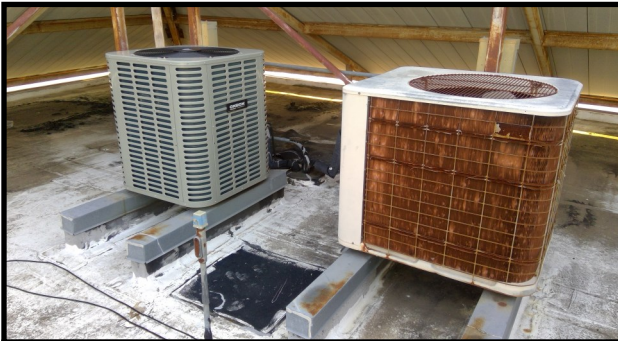
1985 Addition Condensing Units
