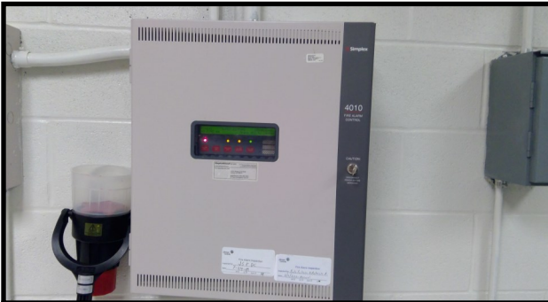
Fire Alarm Control Panel
