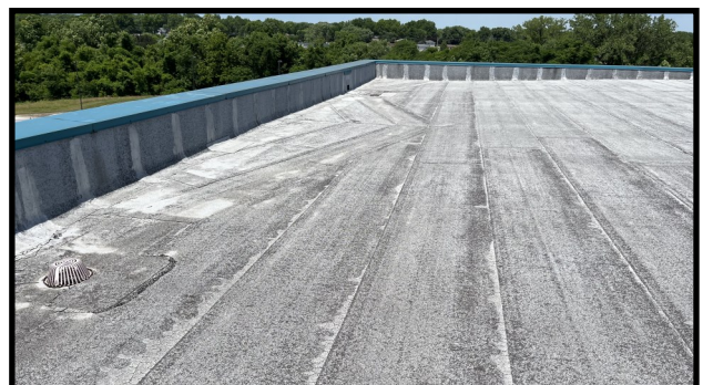
Roof Cracking and Blistering
