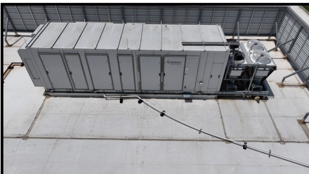
Pool Dehumidification Unit
