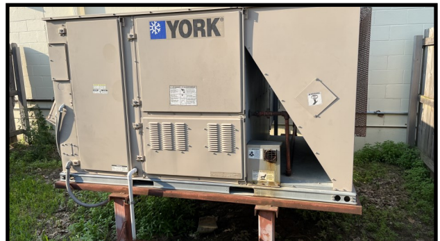
Grade Mounted Packaged Units
