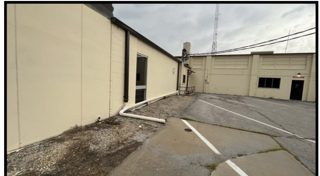
Roof Drain Piping
