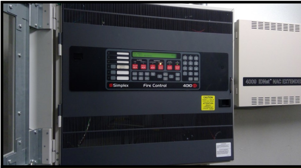
Fire Alarm Control Panel
