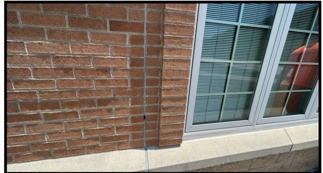
Brick Control Joints
