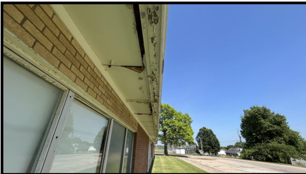
Soffit—Wood Rot
