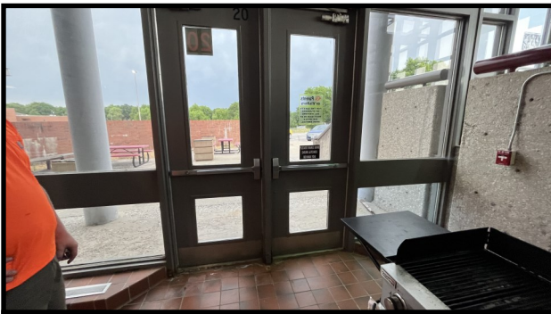
Hollow Metal Curtain Wall
