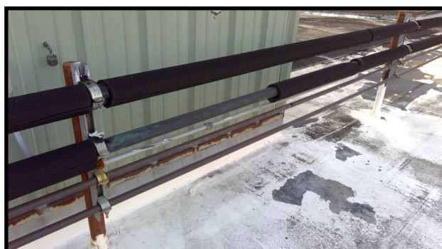
HVAC Piping Insulation
