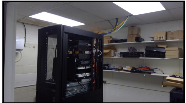
Floor Mounted IT Equipment Racks
